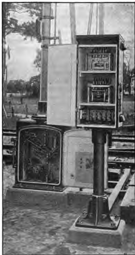
Fig. 204. Galvanometer Track Relays and Style "B" Signal. Washington, Baltimore and Annapolis Ry.
