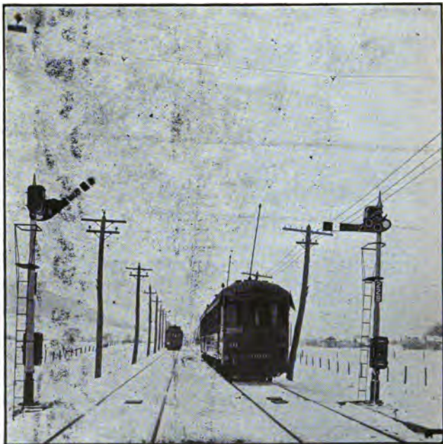
Fig. 197. Three Position Signaling on a High Speed Double Track Interurban Road. New York State Railways.
