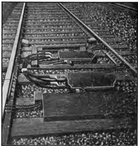
Fig. 91. Track Layout of Two Heavy Traction Impedance Bonds.
