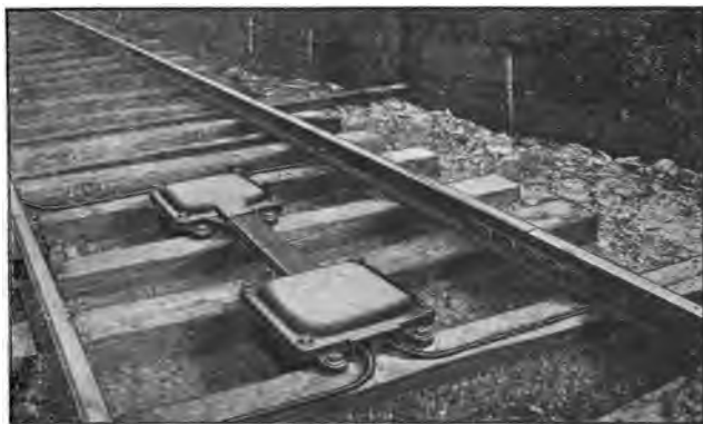
Fig. 92. Track Layout of Two Interurban Road Impedance Bonds.
