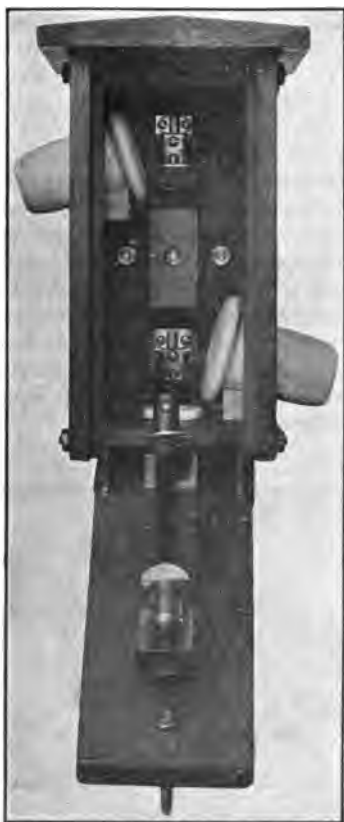
Fig. 188. Expulsion Fuse Cut-Out for Lines over 2200 Volts.
