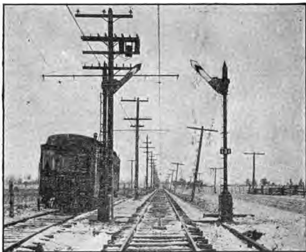
Fig. 12. Interurban Electric Road Signaling Indianapolis, Columbus & Southern
