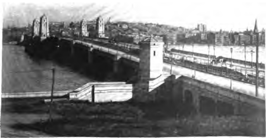
Copyright Brown Bros. CHARLES STREET BRIDGE, BOSTON, MASS. Page 339
