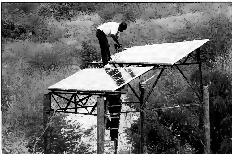
STANDING over solar panels, a worker installs the solar modules that power the water pump. Frank Viscomi, a university engineer, helped install the pump which provided over 5,000 gallons of water on a daily basis. Photo courtesy of Mary Tacy.
