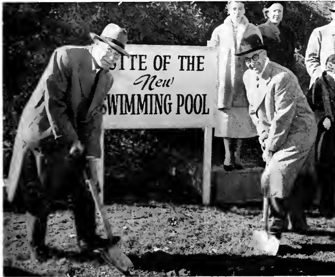
Trustees Alfred G. Freas of Tenafly, N. J. (Left) and Robert L. Rooke '13, of Westfield, N. J., perform for the photographers during the ground-breaking ceremonies for Bucknell's new swimming pool, which were held on Homecoming Day morning. The pool, which these two trustees are giving to the University, is expected to be completed by the fall of 1956.
