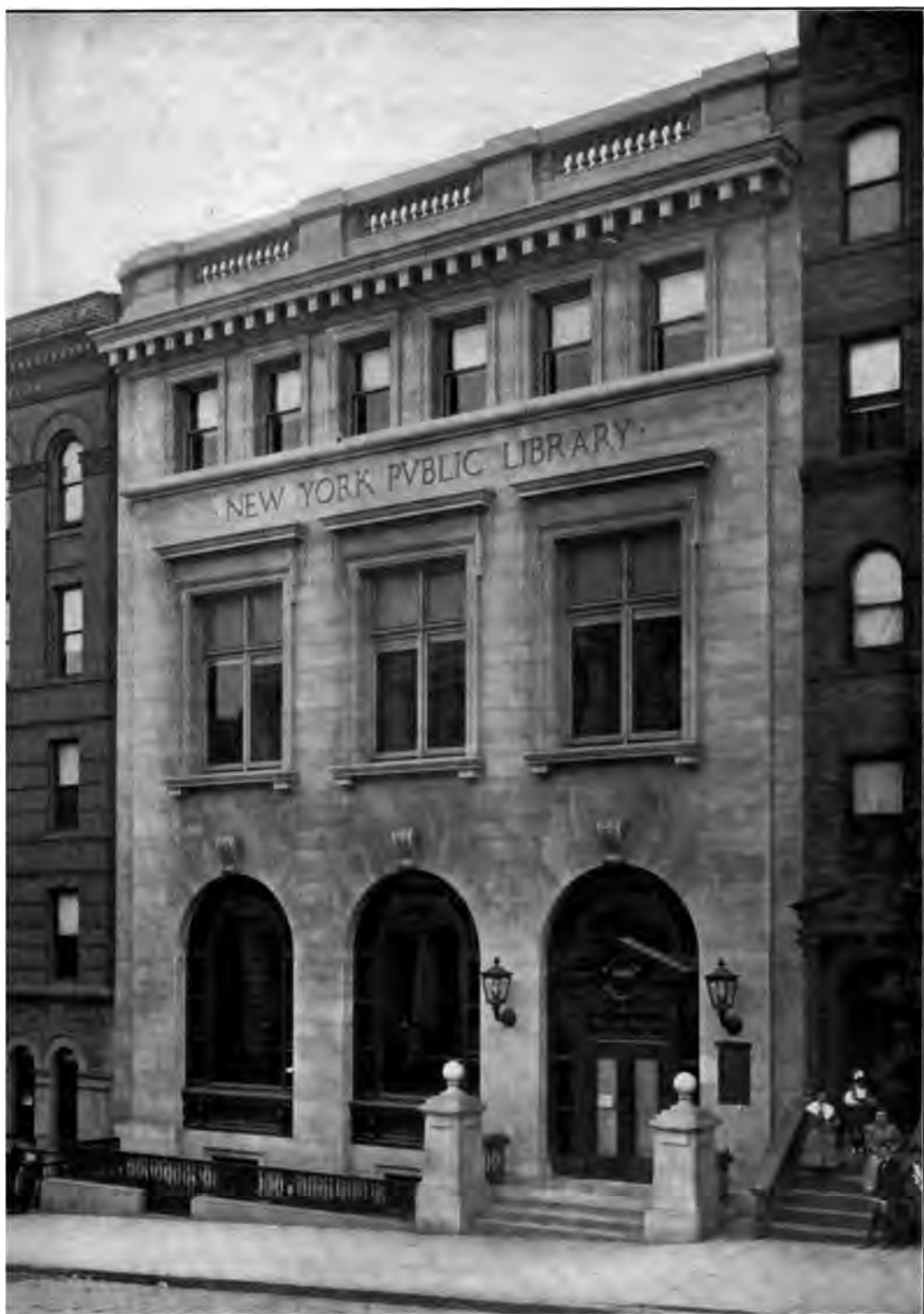
FRONT ELEVATION. NINETY-SIXTH STREET BRANCH, 112 EAST 96TH STREET. NEW YORK PUBLIC LIBRARY—CARNEGIE GIFT.
