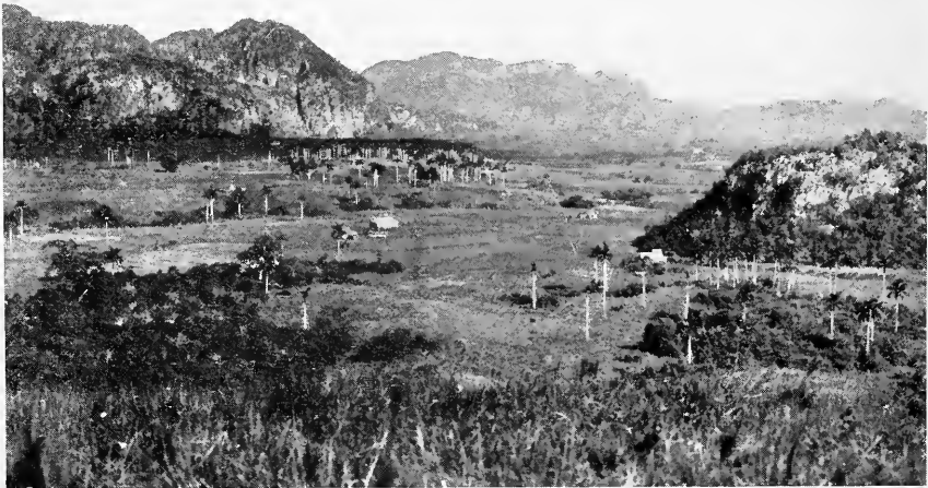
Photograph by American Photo Studios
