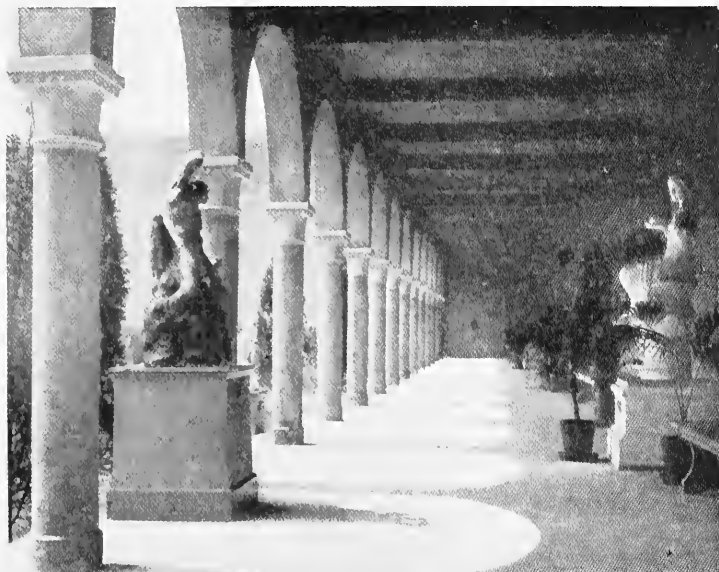
CLOISTER, GARDEN COURT, FINE ARTS BUILDING
