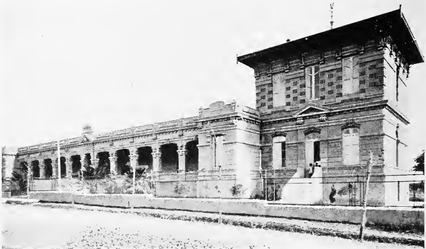
TYPE OF MODERN RURAL SCHOOL BUILDING IN URUGUAY
