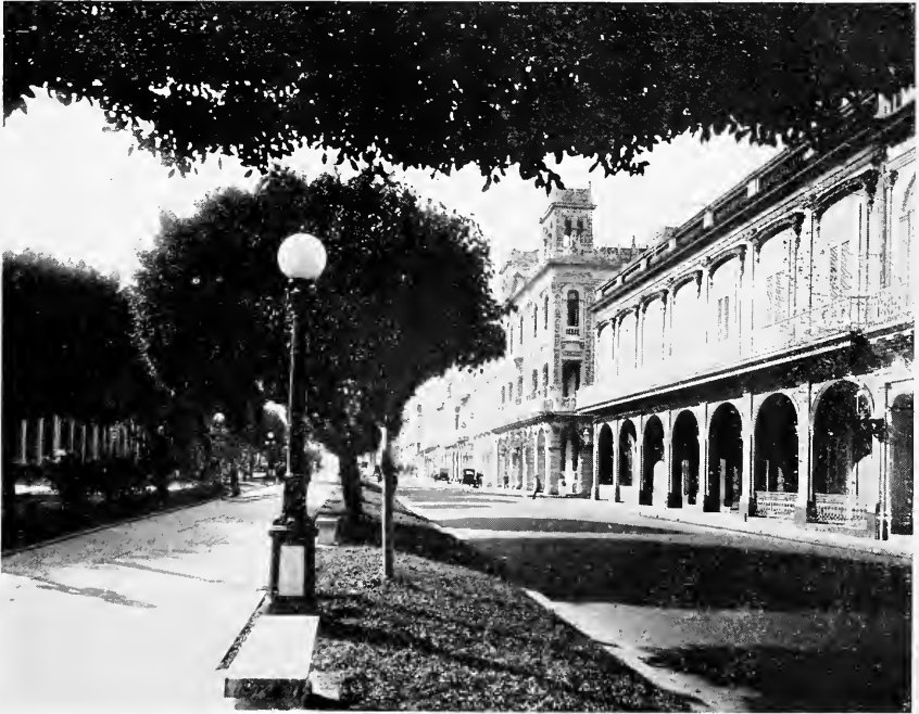
Photograph by American Photo Studios
