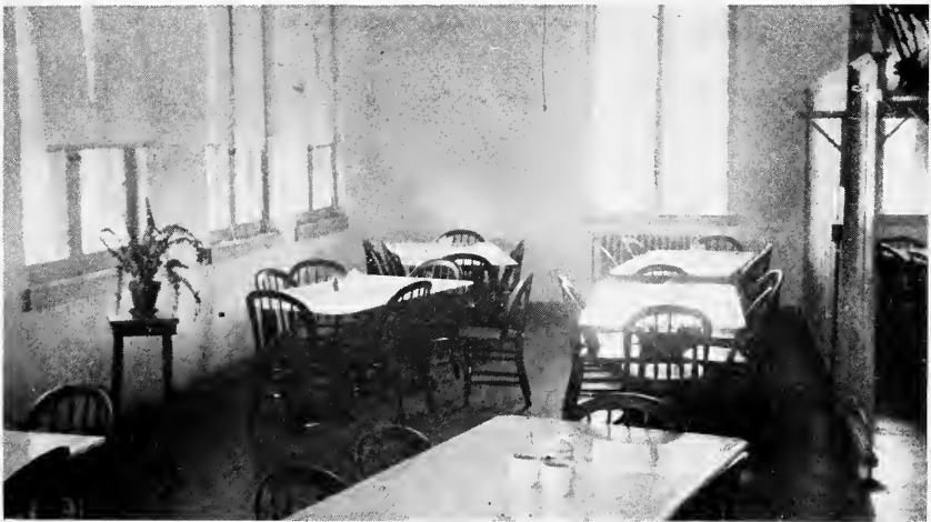
DINING-ROOM COMPARTMENTS, MARINE HOSPITAL NO. 66
