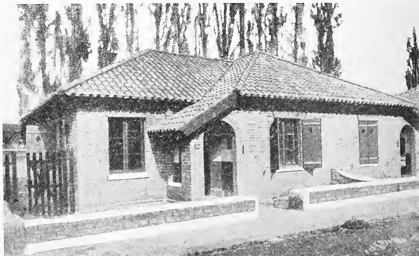
TYPICAL LOW-PRICED HOUSE IN THE GROUP ERECTED IN SANTIAGO, WITH GOVERNMENT AID, BY WORKERS IN THE PRINTING TRADES
