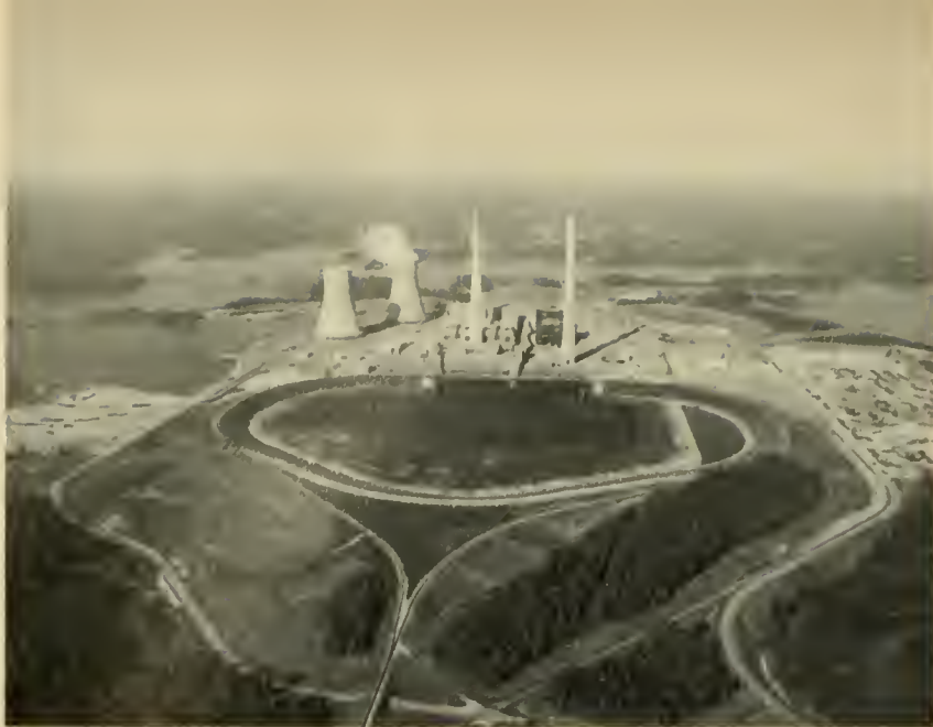
An aerial view of Georgia Power's Plant Scherer, Juliette, Ga.
