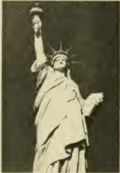
A pre-restoration photo doesn't reveal the structural weaknesses engineers discovered in the Statue.
