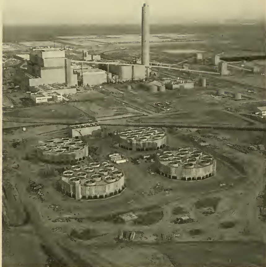
The Intermountain Power Project as it stood one year ago. The cooling towers are in the foreground; the coal handling area is at upper right; and the waste disposal areas are in the background.
