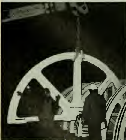
During the 1984 restoration of the cable cars in San Francisco, Calif., hard-hatted workers installed the sheave wheels.
