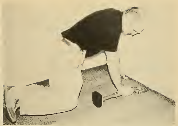
A carpet layer, right, demonstrates the knee kicker. Below right is the power carpet stretcher, a "knee-saving" device.
