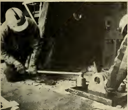
Every major piece of equipment with a turning shaft was leveled and aligned by Millwrights. Included in their work were the two 750 megawatt generators.
