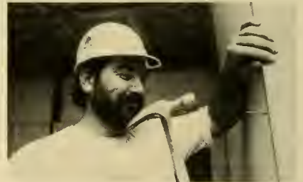
Brian Bailey, Local 906, Glendale, Ariz., looks pleased to be pounding another nail in place for this community service project.
