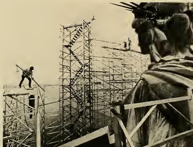
The 300-ton scaffolding was in place for a year and a half while crews worked to complete their work on schedule. Photo © Dan Cornish/ESTO.
