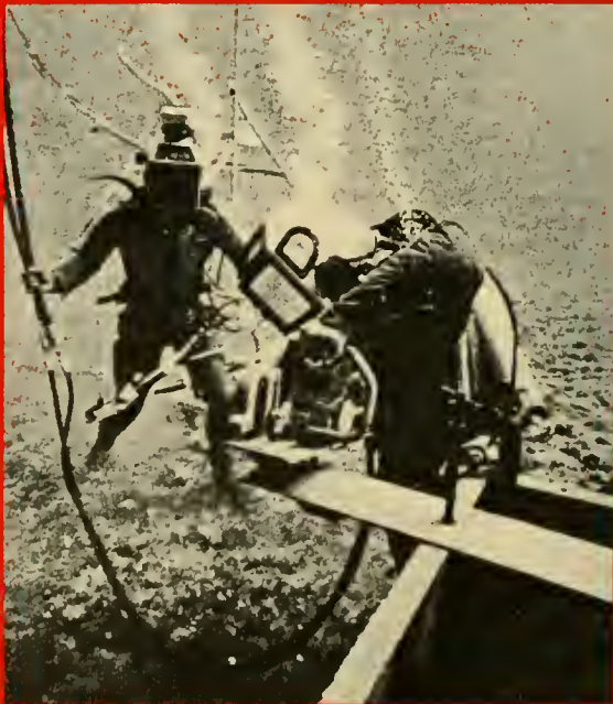
ABOVE: A diagram from the book showing how a six-inch rubber suction hose and a waterjet hose are used while tunneling under a shipwreck to place slings.
