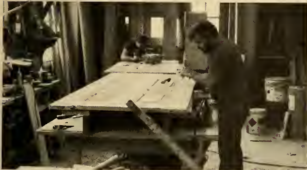
Barry N. Hahn, foreground, and Kenneth W. Wehr Jr., background, work on doors to be installed in the U.S. Department of State's Diplomatic Reception Rooms.
