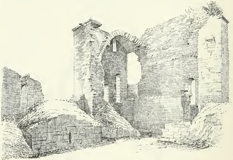
FIG. 224.—Glengarnock Castle. View from North-East Angle of Courtyard.
