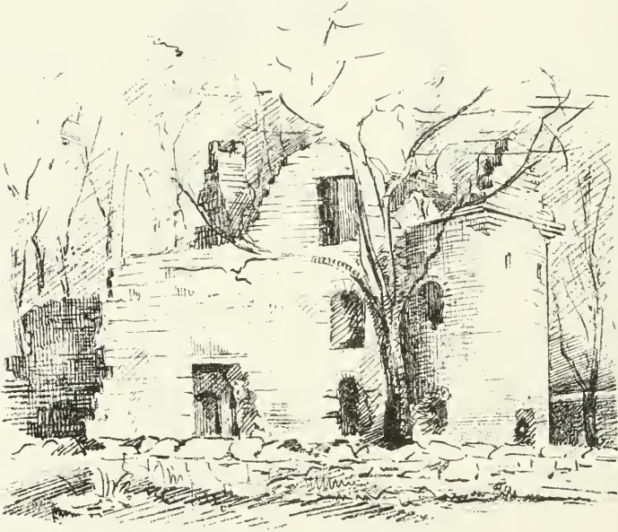
FIG. 555.—Esslemont Castle. View from South.
