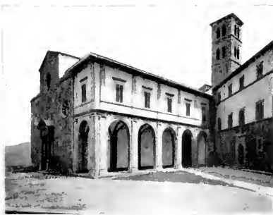
CATHEDRAL, CORTONA (Designed by Antonio da Sangallo?)
