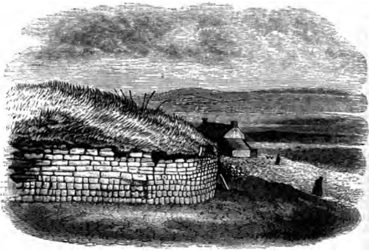
The Station of House-steads; south-west corner.
