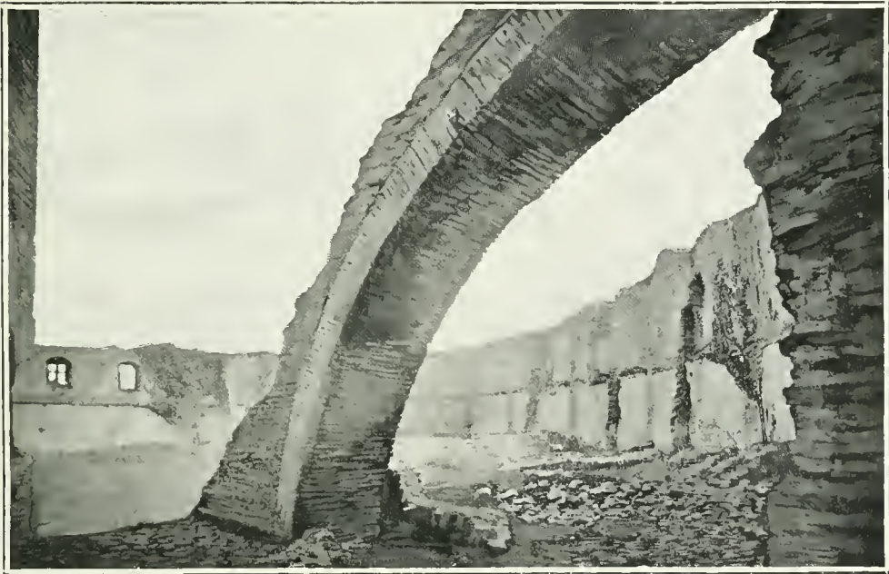
MONTANER. — Contrefort des fortifications.
