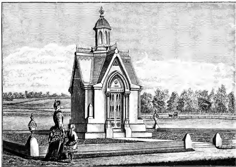
MONUMENTAL CHAPEL, FREDERICKSBURG, PA.
