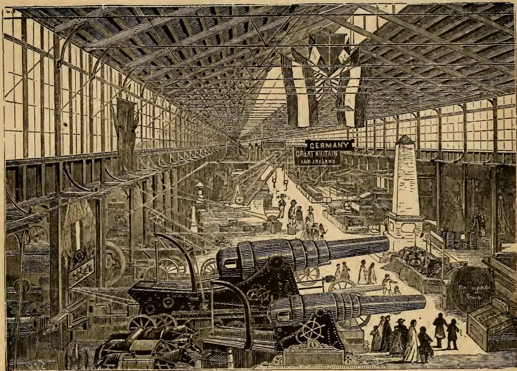
GENERAL VIEW OF THE INTERIOR OF MACHINERY HALL.
