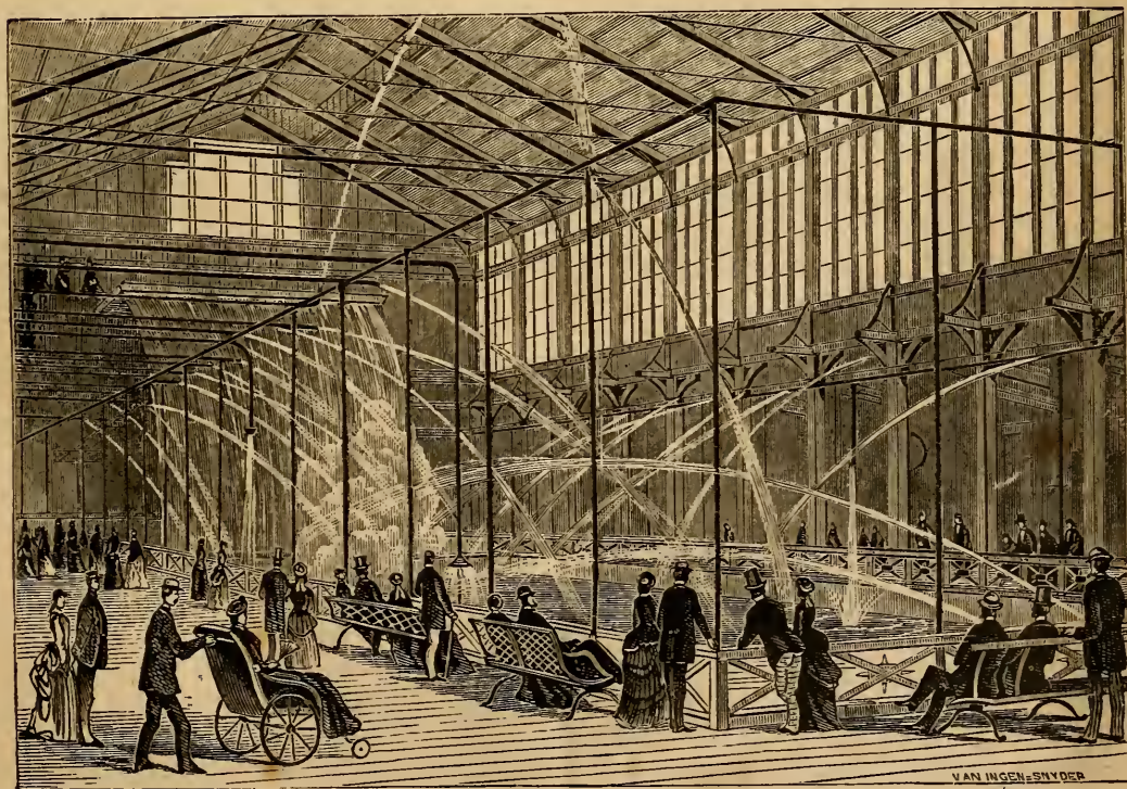
THE HYDRAULIC BASIN, IN MACHINERY HALL.
