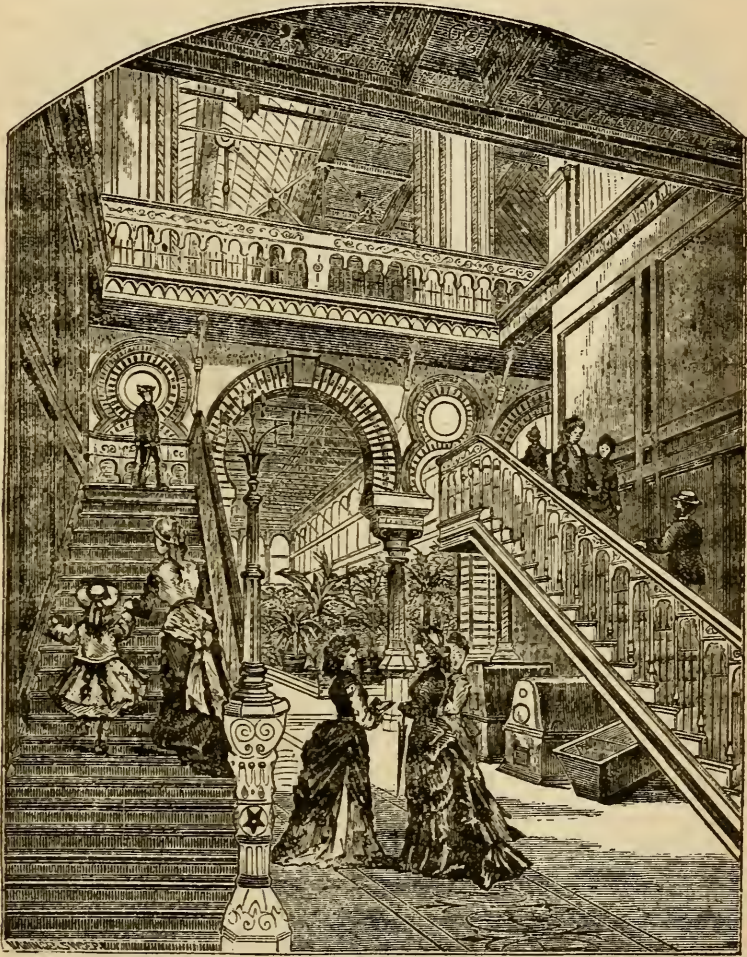
STAIRWAY IN HORTICULTURAL HALL.
