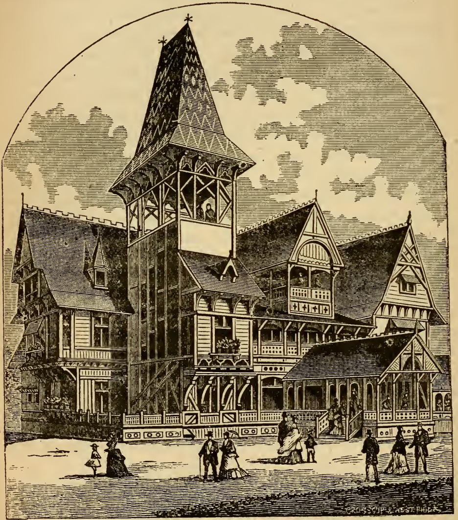
NEW JERSEY STATE BUILDING.
