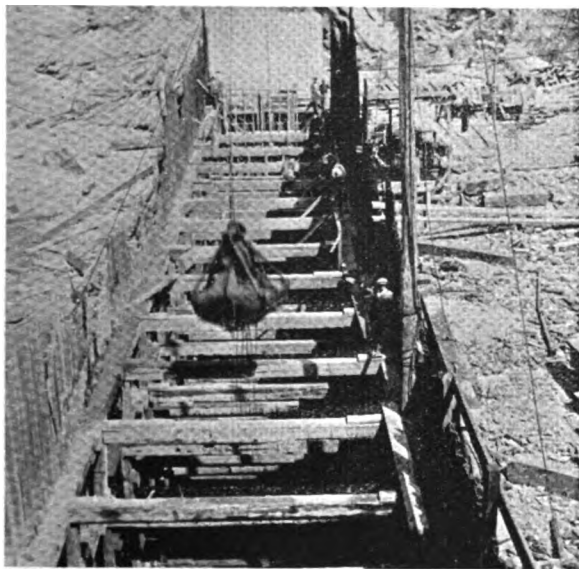
TIMBERING OF DEEP-CORE WALL TRENCH.
