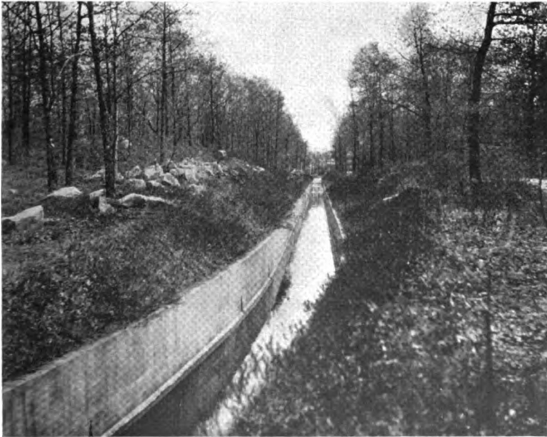
FIG. 4. — 8 FT. OPEN SECTION OF INTERCEPTING DRAIN — NOVEMBER, 1921.
