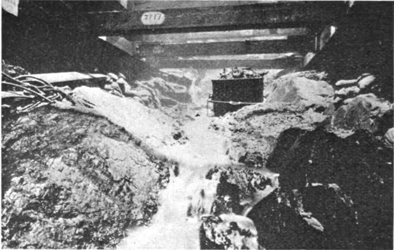
BOTTOM OF DEEP CORE-WALL TRENCH.
