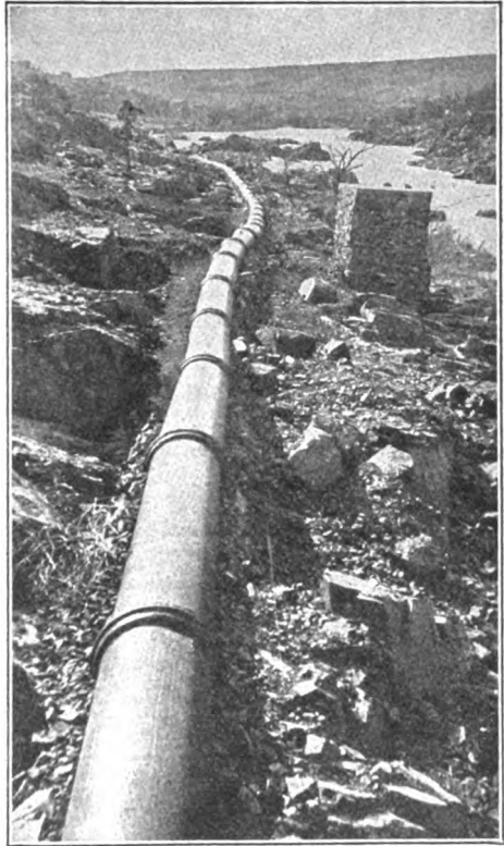
24" Line looking South from Dam through Medicine Canyon.
