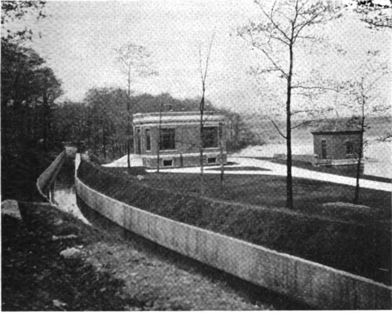
FIG. 3. — AUXILIARY PUMPING STATION AND INTAKE, ALSO 10 FT. OPEN SECTION OF INTERCEPTING DRAIN — NOVEMBER, 1921.
