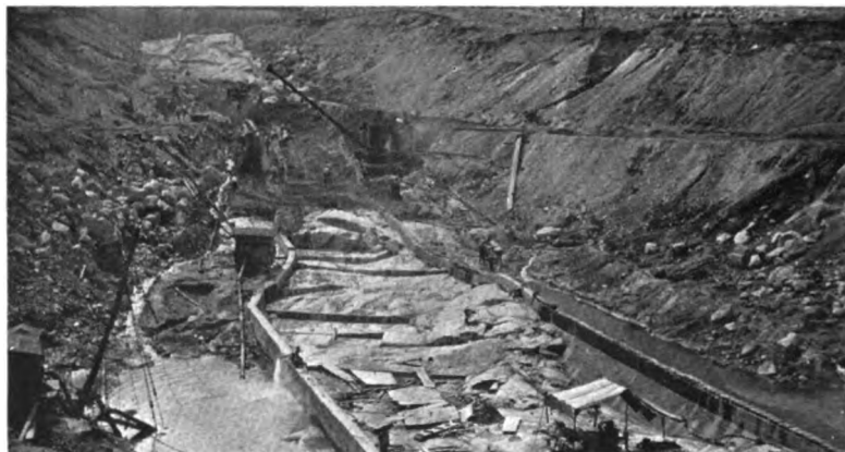
MAIN DAM, SCITUATE RESERVOIR.
