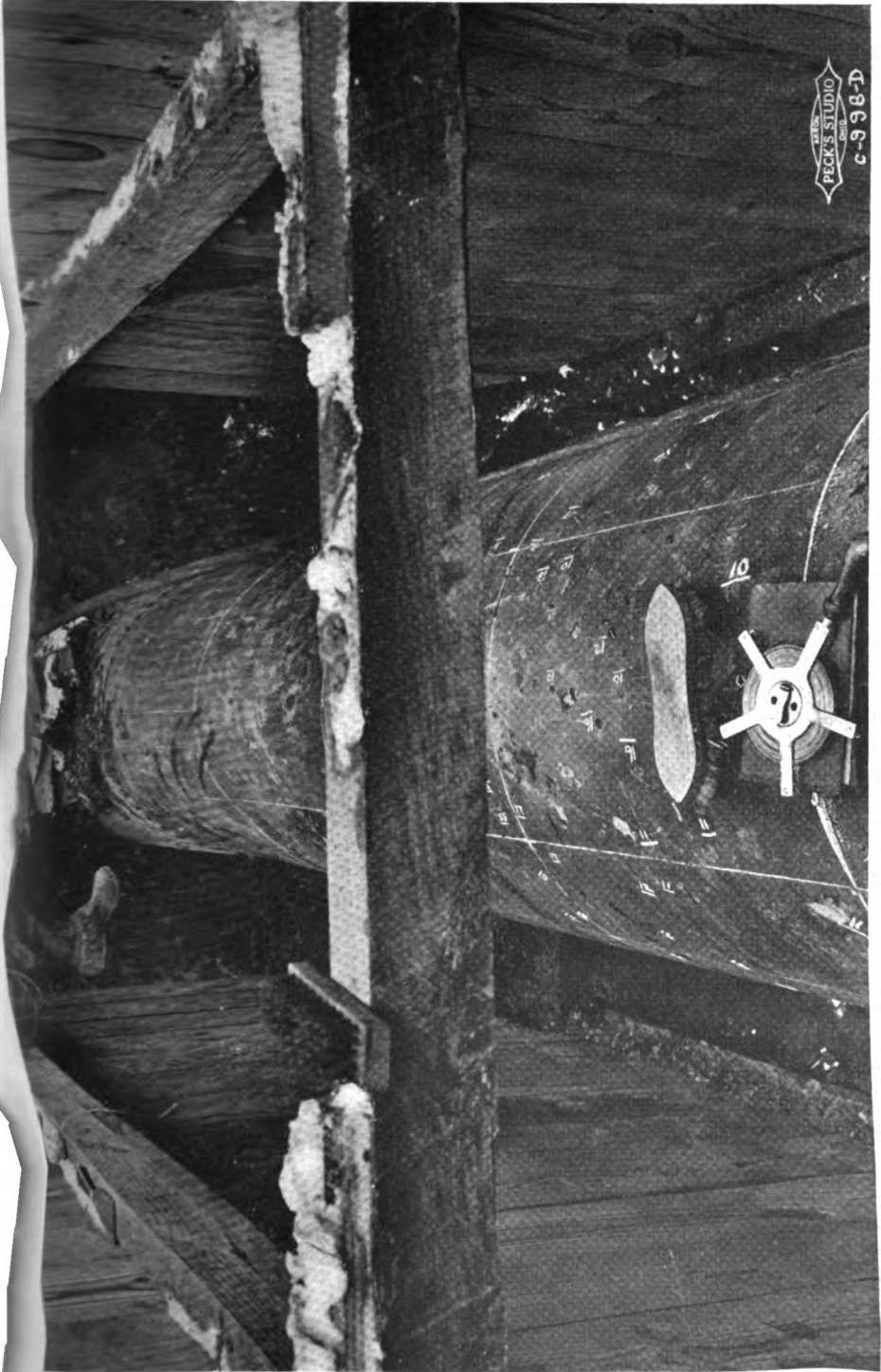
PLATE III. PHOTOGRAPH OF CORRODED STEEL PIPE AT STATION 440.
