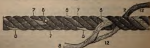
FIG. 81. SPlicing OF ROPES.
