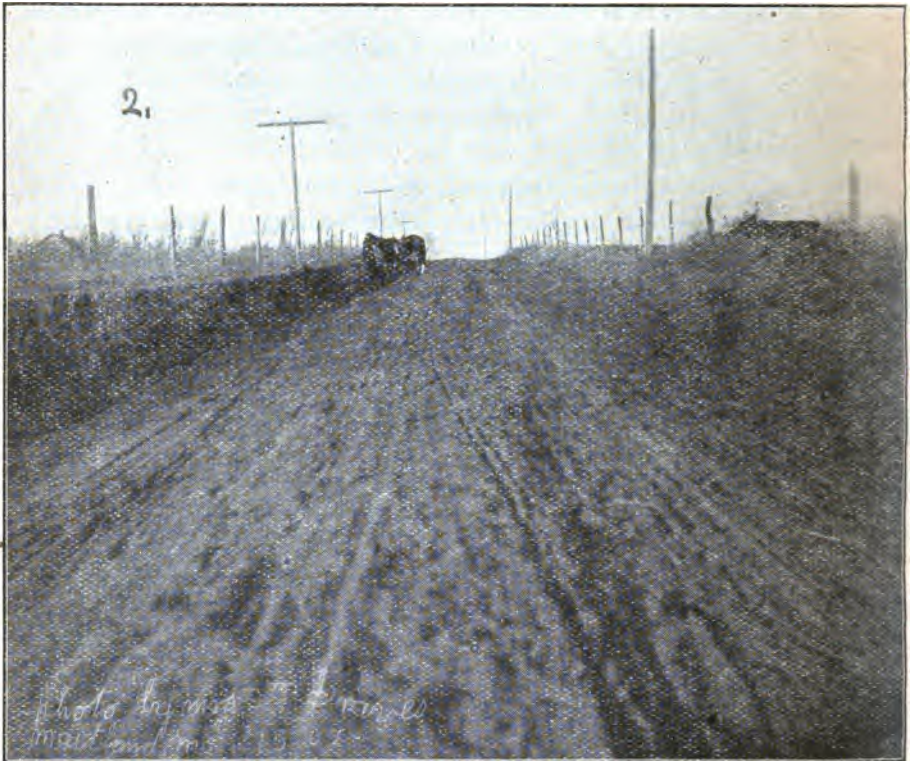
From a photograph taken of Mr. King's road, showing smooth surface.
