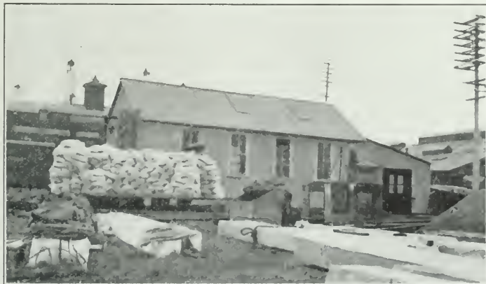
Fig. 4. Pile Carrying Test Load.
