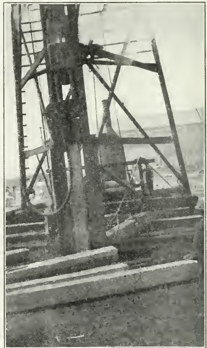
Fig. 2. A Concrete Pile Under the Hammer.
