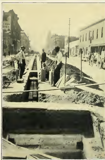
Conduits in Course of Construction
