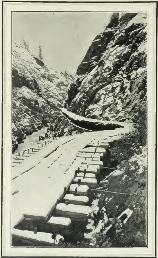
All Repairs Must Be Made When Snow Is Deep Along the Flume
