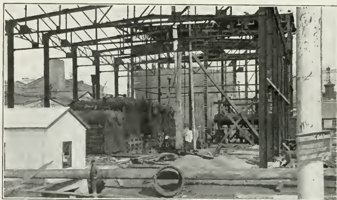
Station under Construction.
