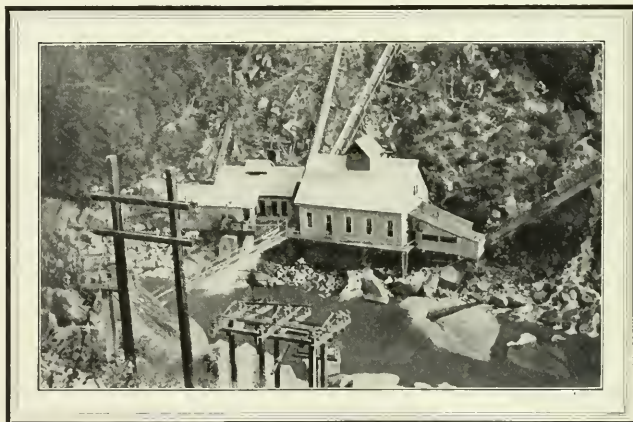
The Nevada Power House on the South Yuba River
