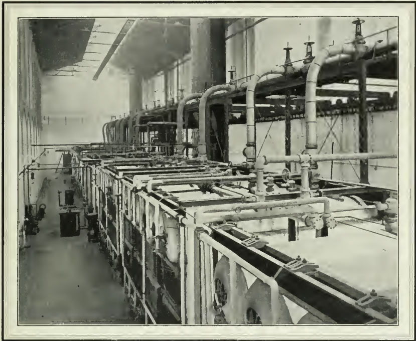
View in the Boiler Room, Looking South
