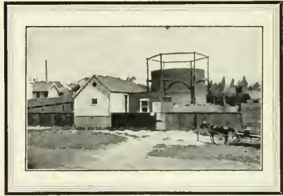
The Office, the Meter-room, and the Gas Holder to Which a Second Lift Was Added While In Use
