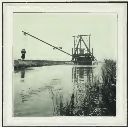
A Dredger Throwing Up a Levee
