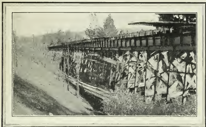
Pipe-line and elevated flume near Gold Run
