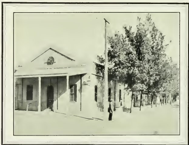
Original Gas Works Building, Second and B Streets, Showing One of Old Cast-Iron Retorts at Corner, Between Men
