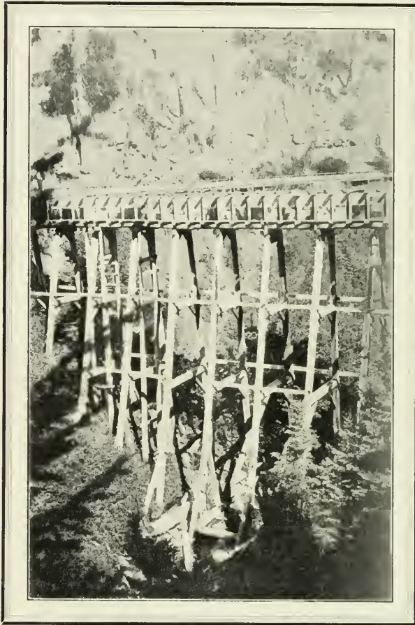
A Section of High Flume near Steep Hollow. Note Man on Top
