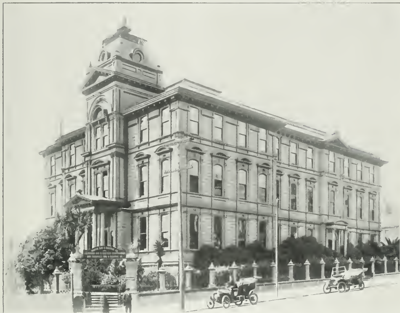
The Convent at Franklin and Eddy Streets, the Company's Home for Three Years, from the Second Month After the Fire until the Removal to its Own New Building
