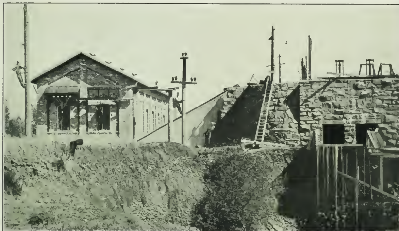
Folsom Power House and Granite Forebay
