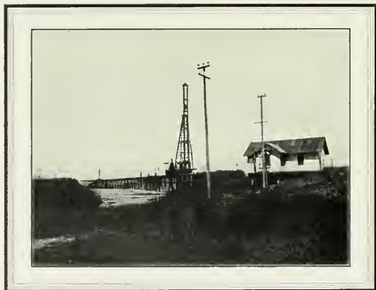
The Orwood 200-Horsepower Pumping Plant
