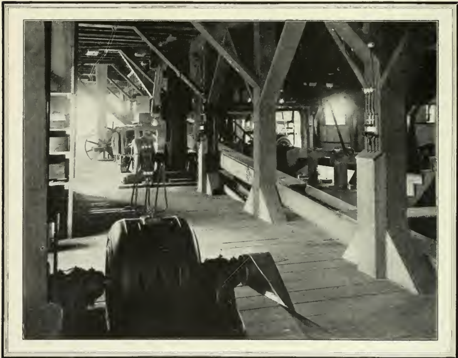
A view inside the old Folsom Sawmill—in the foreground the motor that operated the endless chain pulling logs up out of the pond; in the centre the motor that operated the edger; on the right the small amount of shafting that operated the cut-off, the sawdust conveyor, and the live rolls
