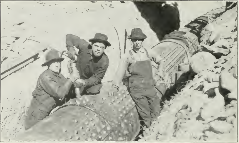
Fig. 3. Riveting.
