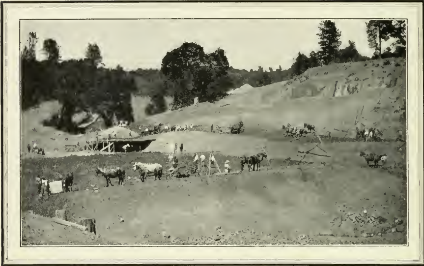
Building the core of the dam for Lake Arthur
