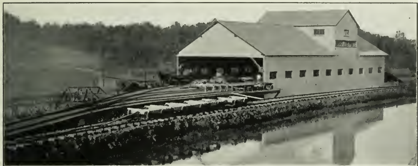
Down-stream end of the old Folsom Sawmill, showing horse-drawn lumber cars, and the railroad leading to the lumber yard; to the left the sawdust chute down into the river; and in the background the Folsom steel bridge across the American river
