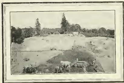
Lake Arthur Dam in the Making
