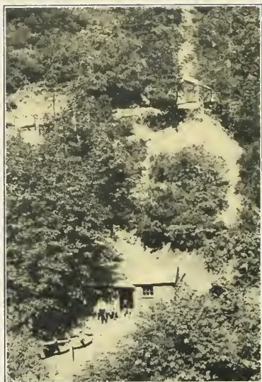
Tunnel Entrance, Morning Glory Mine, Alleghany
