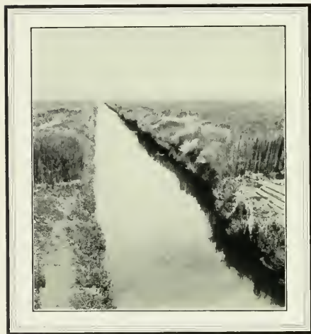
A Main Drainage Ditch
