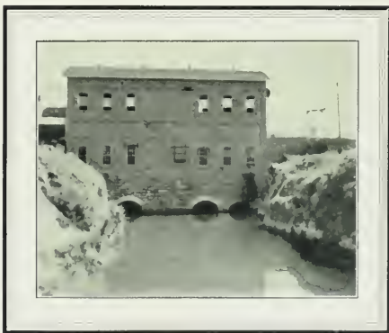
The Folsom Power House, With Outflow Canal Through Solid Granite
