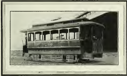
One of the Later Horse Cars Run By Storage Battery
