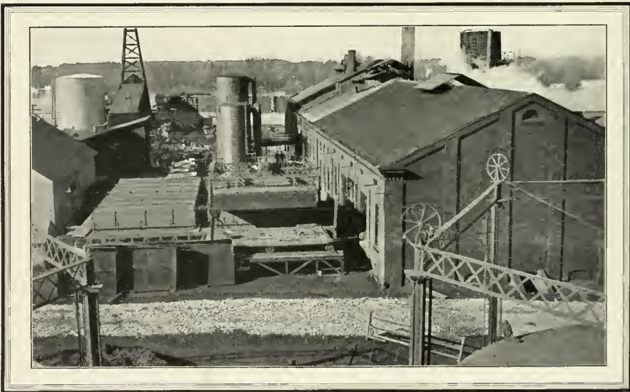
General View at the Sacramento Gas Works
