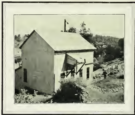
Secondary Plant at Folsom Power Station, Run by Outflow From First
