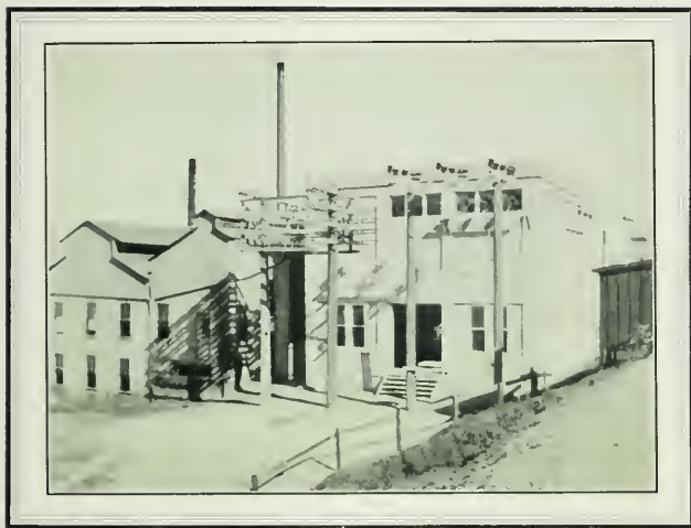
Gas Works and Electric Substation, View Taken from Levee
