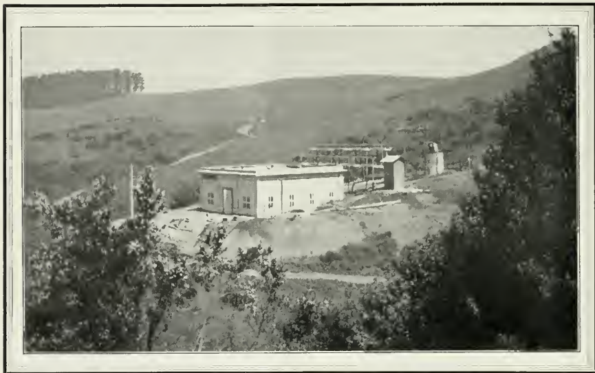
(FIG. 1) THE RIDGE SUBSTATION
