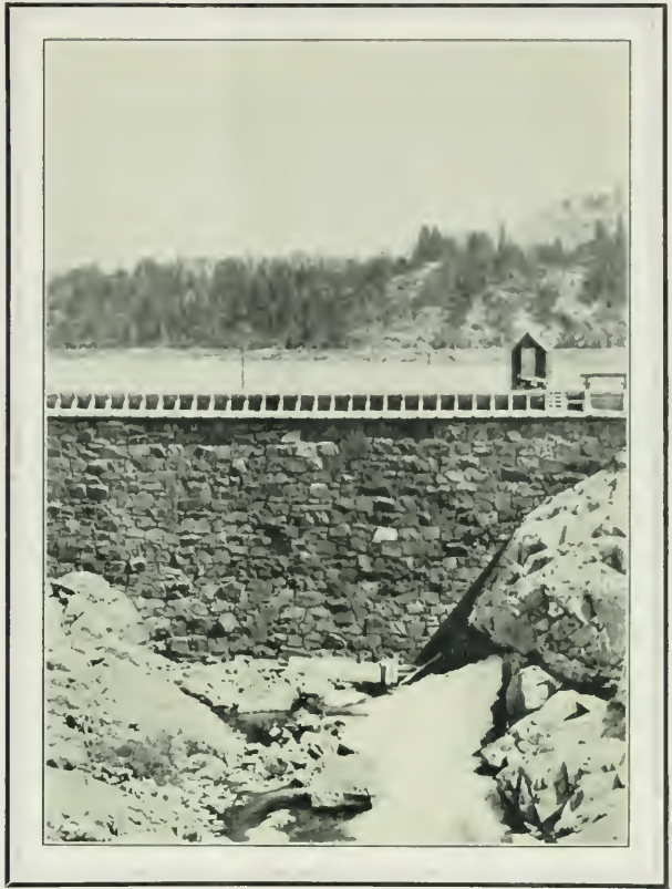
DAM AT LAKE SPAULDING
