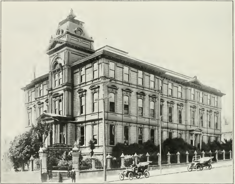
General Offices, Pacific Gas and Electric Company, Southwest Corner Franklin and Ellis Streets, since June, 1906.
