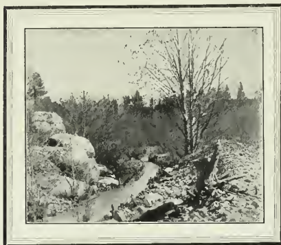
The Ditch Flowing Into Lake Vera, Bringing Water from the Deer Creek Power House
