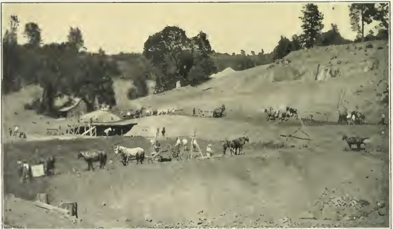
Lake Arthur Dam During Construction
