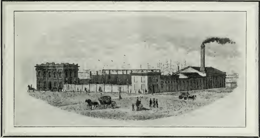
GAS WORKS AT FIRST AND HOWARD STREETS
