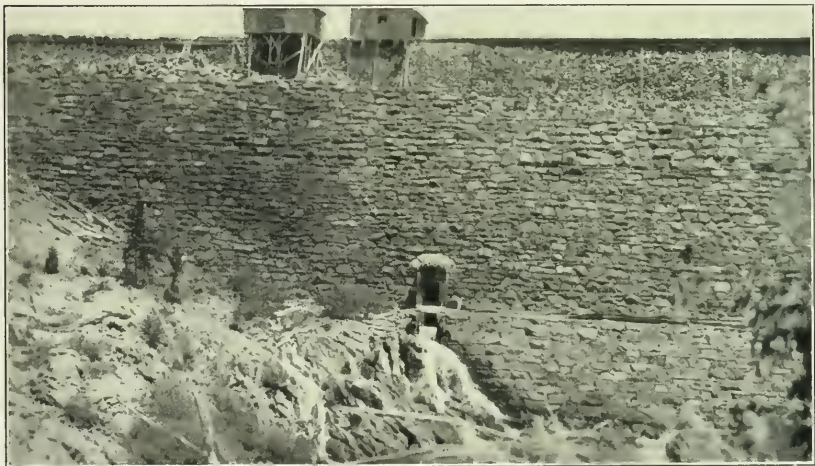
DOWNSTREAM FACE OF FORDYCE DAM
