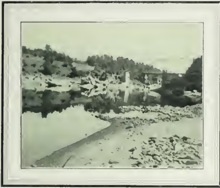
County Bridge Across American River; Also Old Stone Abutment That Supported First Transcontinental Railroad Bridge
