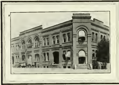
The Electric Power House and Substation
