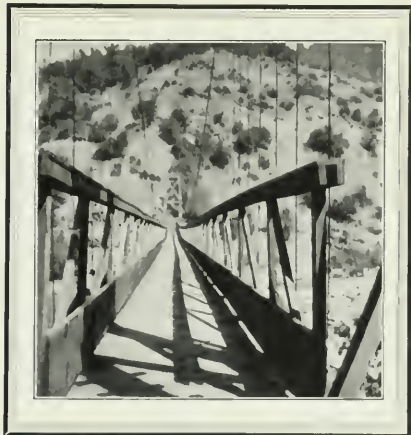
The suspension bridge across the Yuba River at the Colgate plant—for man and horse
