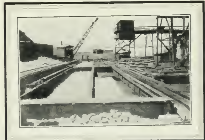
Where the Lampblack Is Separated From the Water
