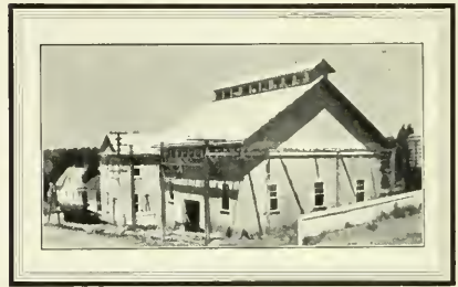
The Grass Valley Substation of Today
