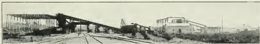
Plant of the Natoma Rock-crushing Company, near Folsom, where the tailings from gold dredgers are made into ballast for railroads and streets
