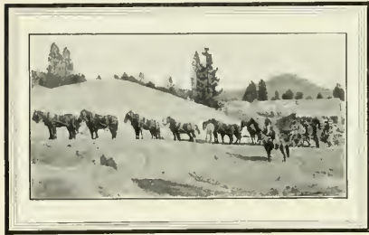
Hauling the Machinery to the Power House in 1895
