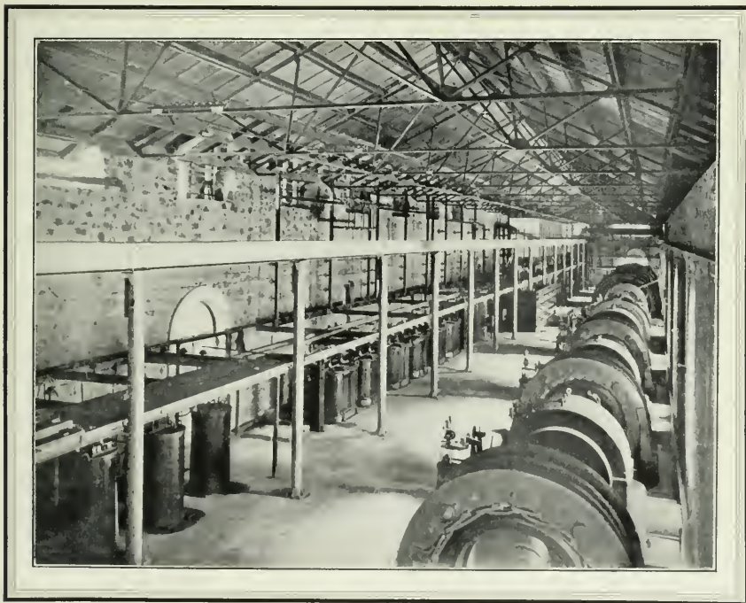
Interior View of Colgate Power House, Looking Upstream
