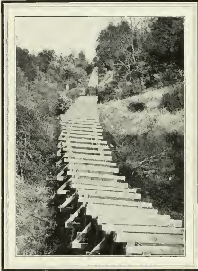
A section of rapid-flume from Lake Frances
