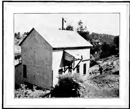
Secondary Plant at Folsom Power Station, Run by Outflow From First
