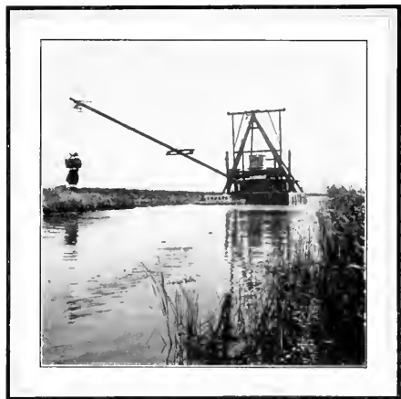
A Dredger Throwing Up a Levee
