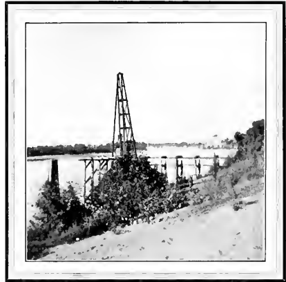
Pier on Sacramento River Where Fuel-Oil Is Delivered at the Gas Works
