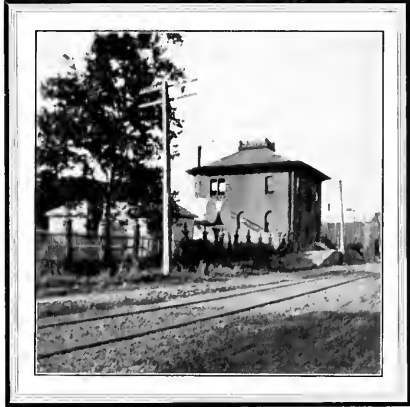
The Old Office Building at the Sacramento Works
