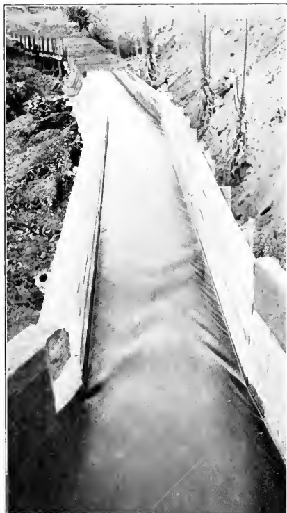
WATER LEAVING ALTA POWER HOUSE
