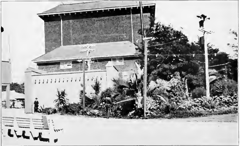
View of Idora Park Transformer House and Terminal Pole
