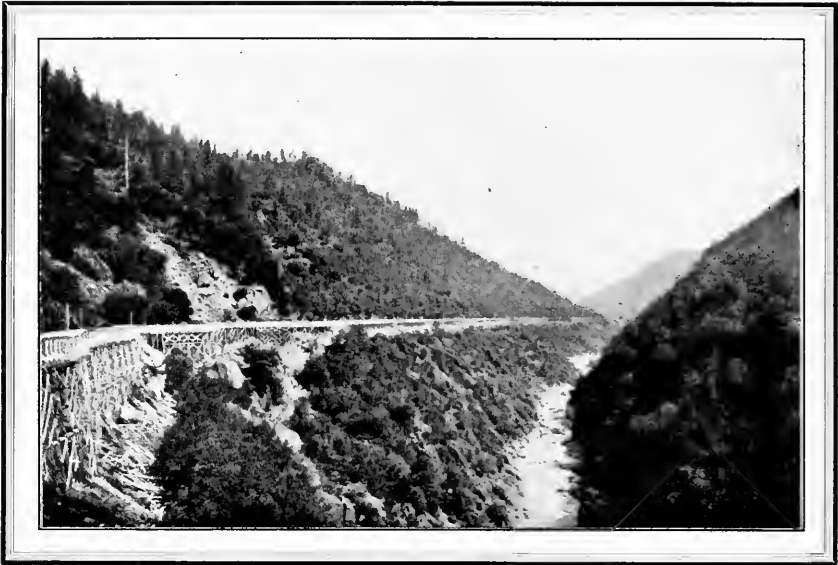
Four Miles of the Colgate Flume in Sight
