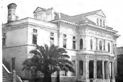
Second Month After the Fire—Loughborough Residence, Northwest Corner O'Farrell and Franklin Streets
