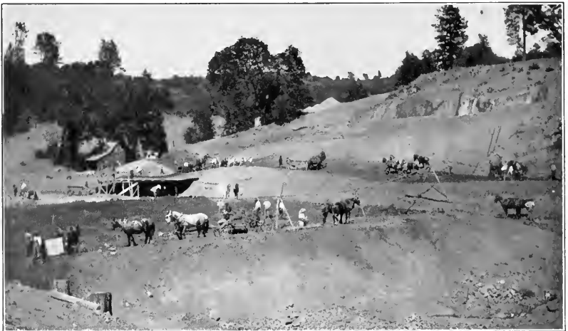
Lake Arthur Dam During Construction
