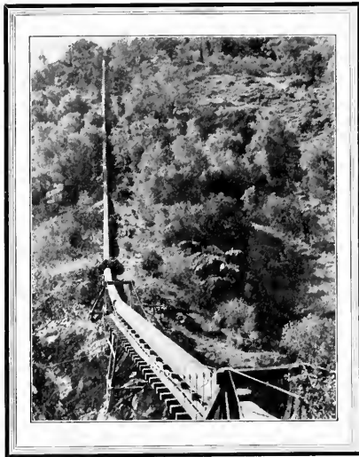
An inverted syphon carrying the Brown's Valley ditch across a cañon below the Yuba power plant
