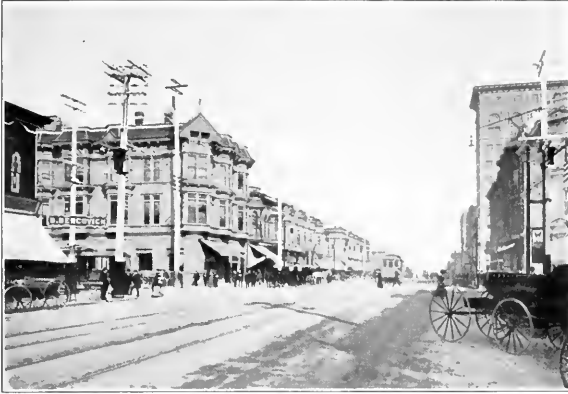
A Mass of Poles and Wires on Broadway at Eleventh Street
