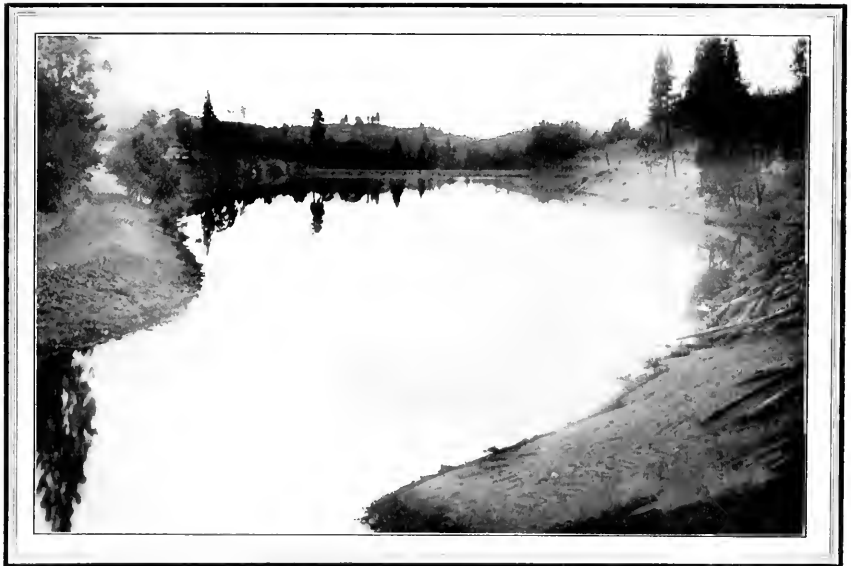
Lake Arthur, looking toward the dam. County Road is at right.
