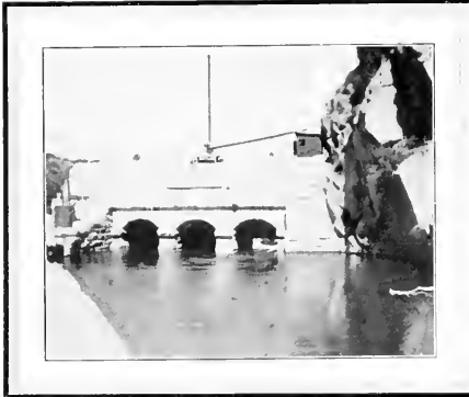
Downstream Face of Canal Headgates, Showing Massive Granite Bluff at Right
