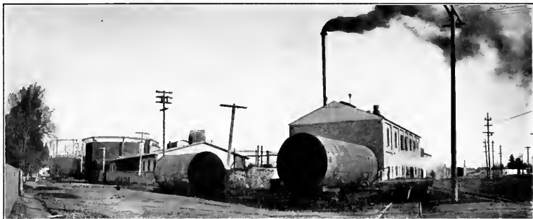
General View of the Gas Works at San Jose
