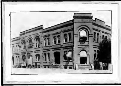
The Electric Power House and Substation
