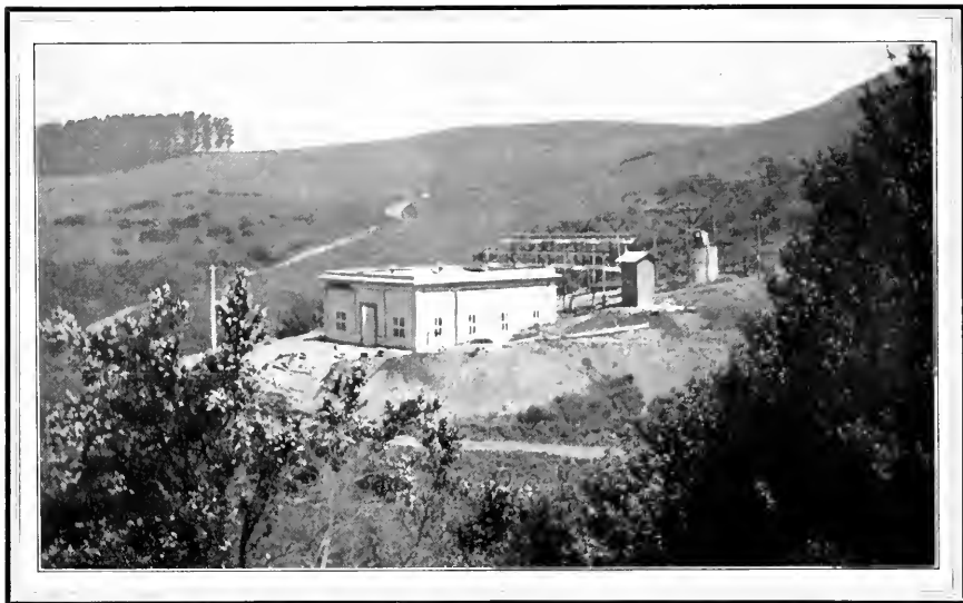
(FIG. 1) THE RIDGE SUBSTATION
