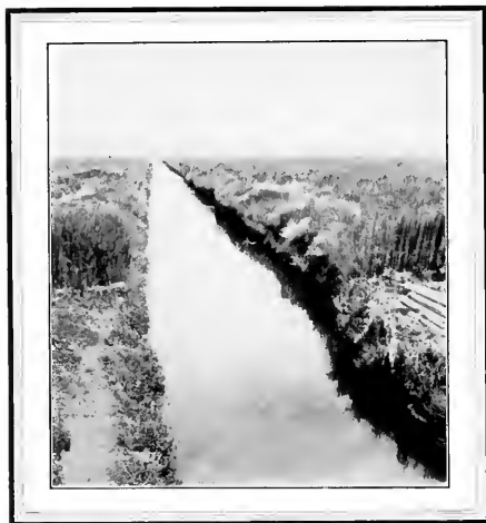
A Main Drainage Ditch
