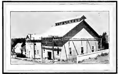
The Grass Valley Substation of Today
