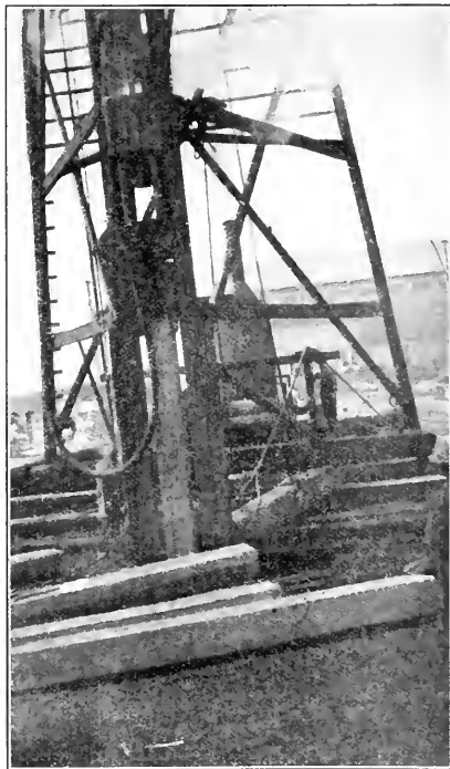
Fig. 2. A Concrete Pile Under the Hammer.
