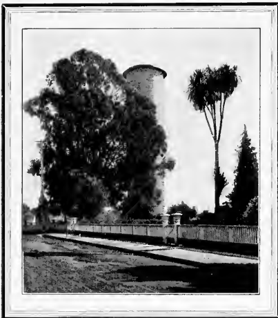
The Water Tower in Napa
