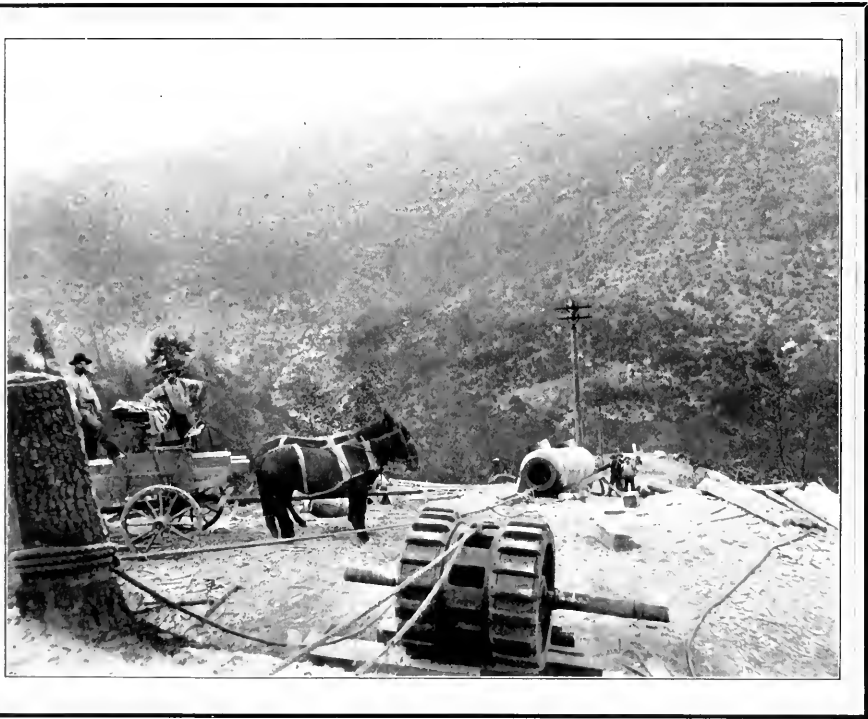
Where the Massive Machinery Was Unloaded at the Top of the Ridge to Be Skidded Down Half a Mile
