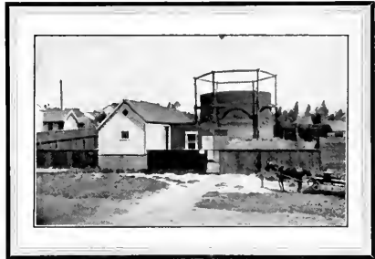
The Office, the Meter-room, and the Gas Holder to Which a Second Lift Was Added While In Use
