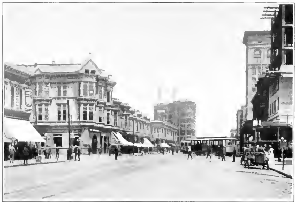
The Same Scene, after the Underground Conduit Took the Wires
