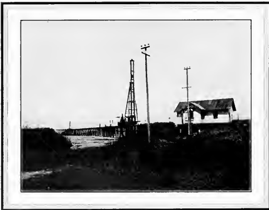
The Orwood 200-Horsepower Pumping Plant
