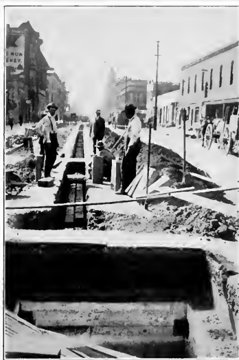
Conduits in Course of Construction
