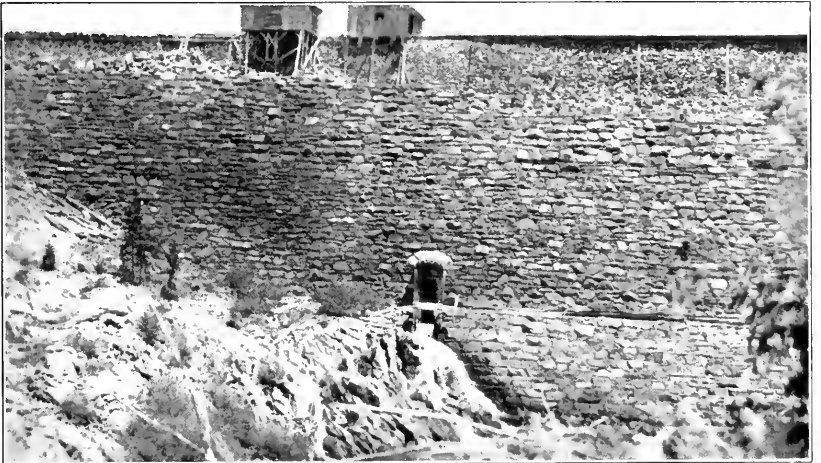
DOWNSTREAM FACE OF FORDYCE DAM
