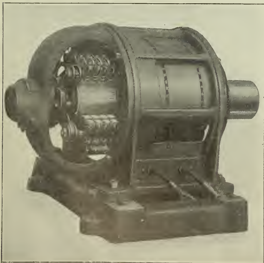
FIG. 363. GENERAL ELECTRIC SINGLE-PHASE COMPENSATED REPULSION MOTOR
