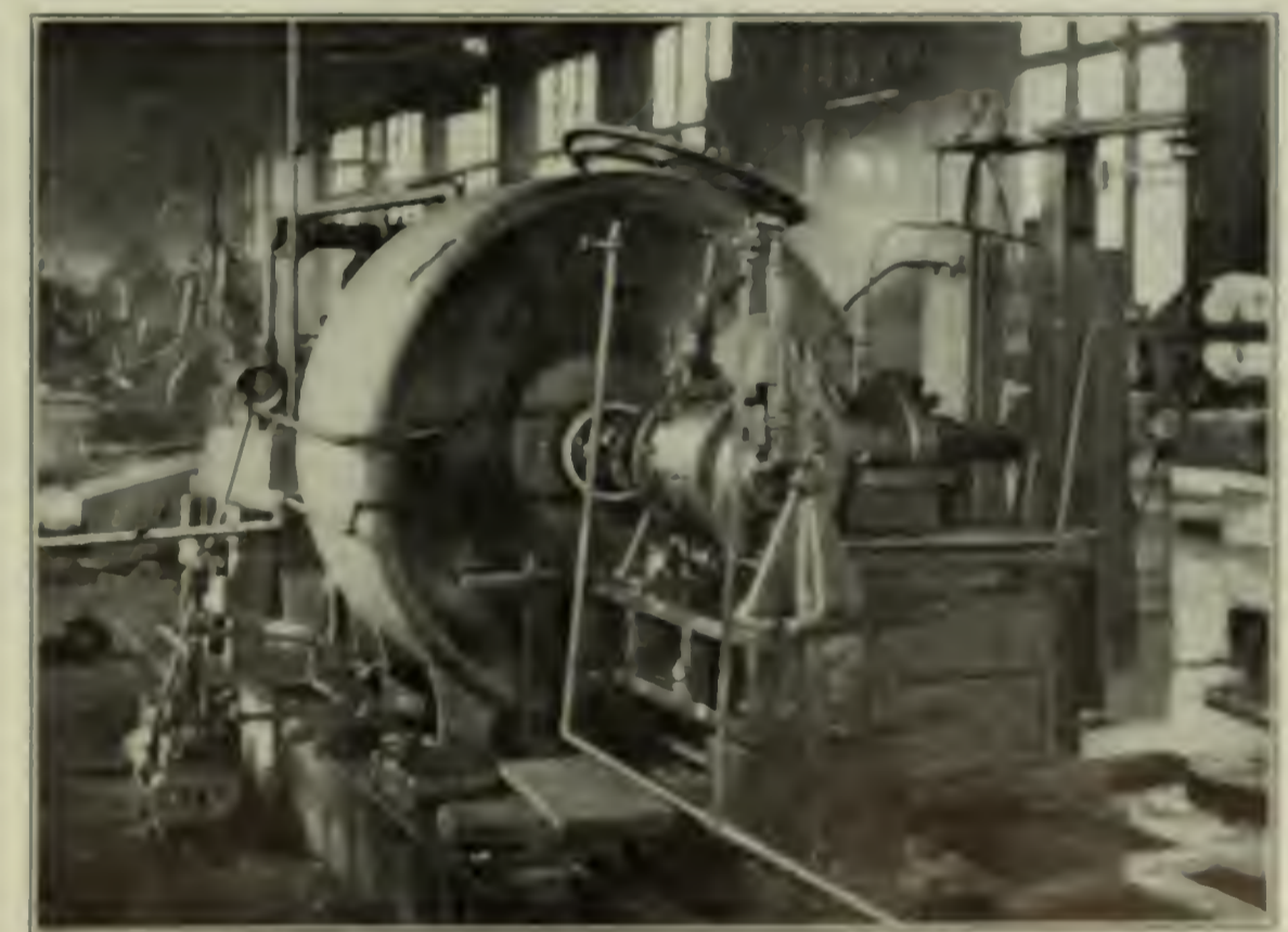
FIG. 5. TURBINE READY FOR TESTING
