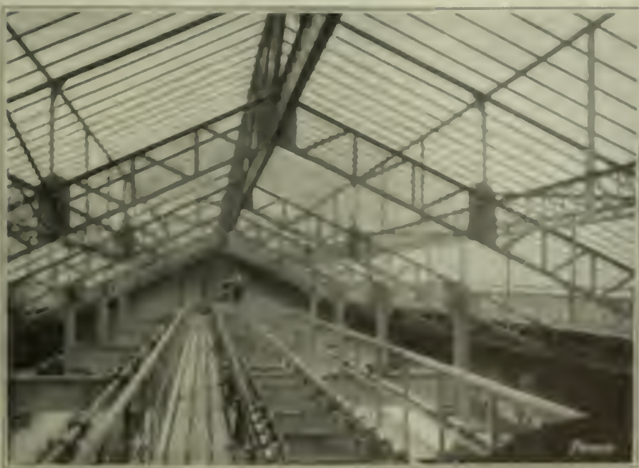
FIG. 5. CONVEYER OVER BOILERS.
