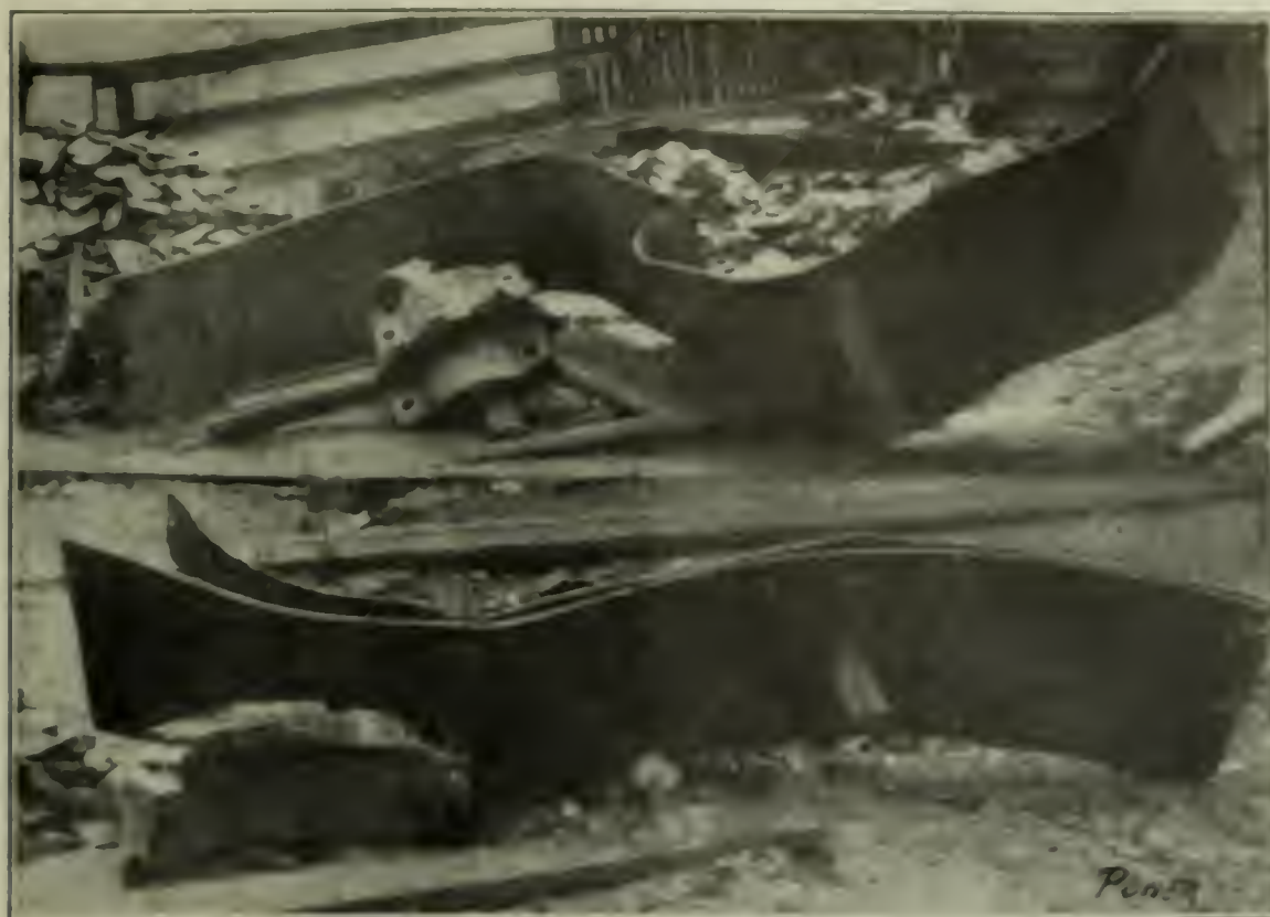
FIG. 3. TWO VIEWS OF THE STEEL RIM
