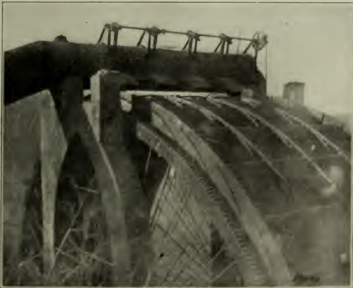
FIG. 4. PENITENCE AND ARRANGEMENT OF GATE CONTROL
