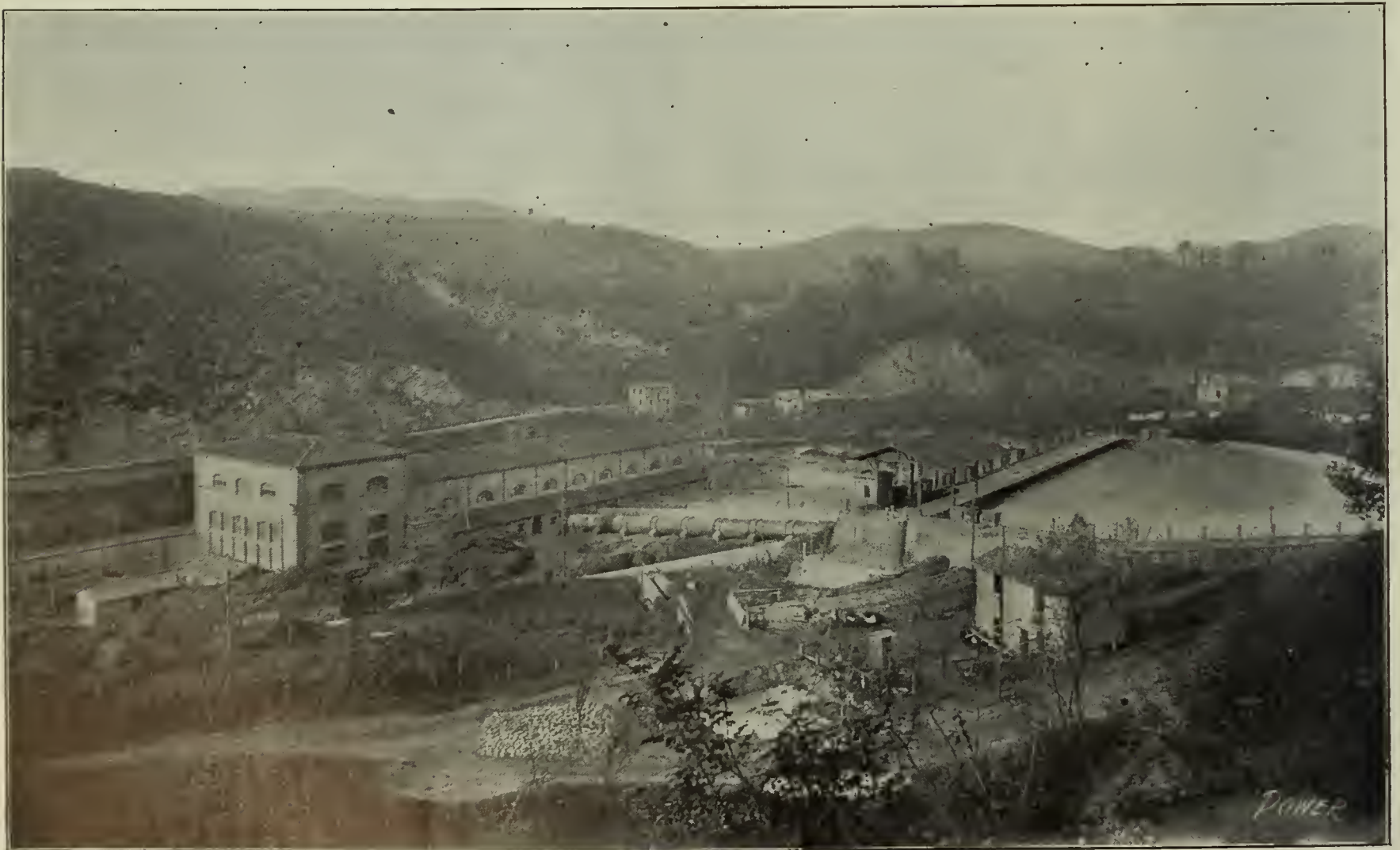
FIG. 1. GENERAL VIEW OF PLANT, SHOWING PENSTOCKS AND RESERVOIR
