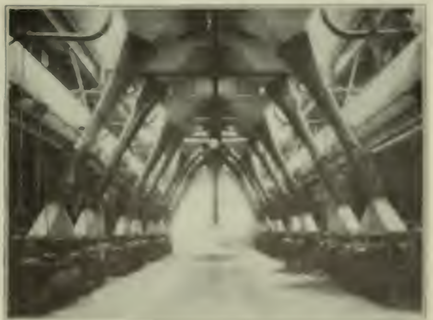
FIG. 6. VIEW OF THE BOILER ROOM.
