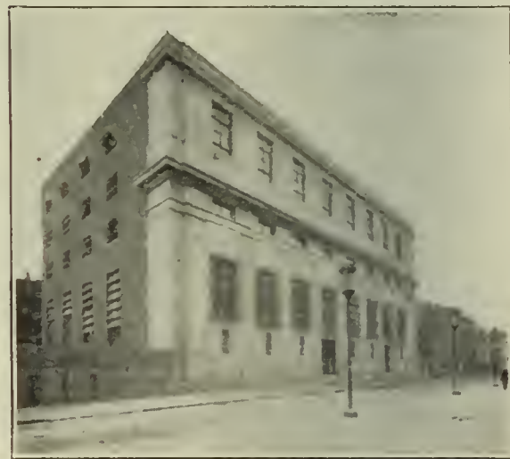
FIG. 3. EXTERIOR VIEW OF SERVICE PLANT
