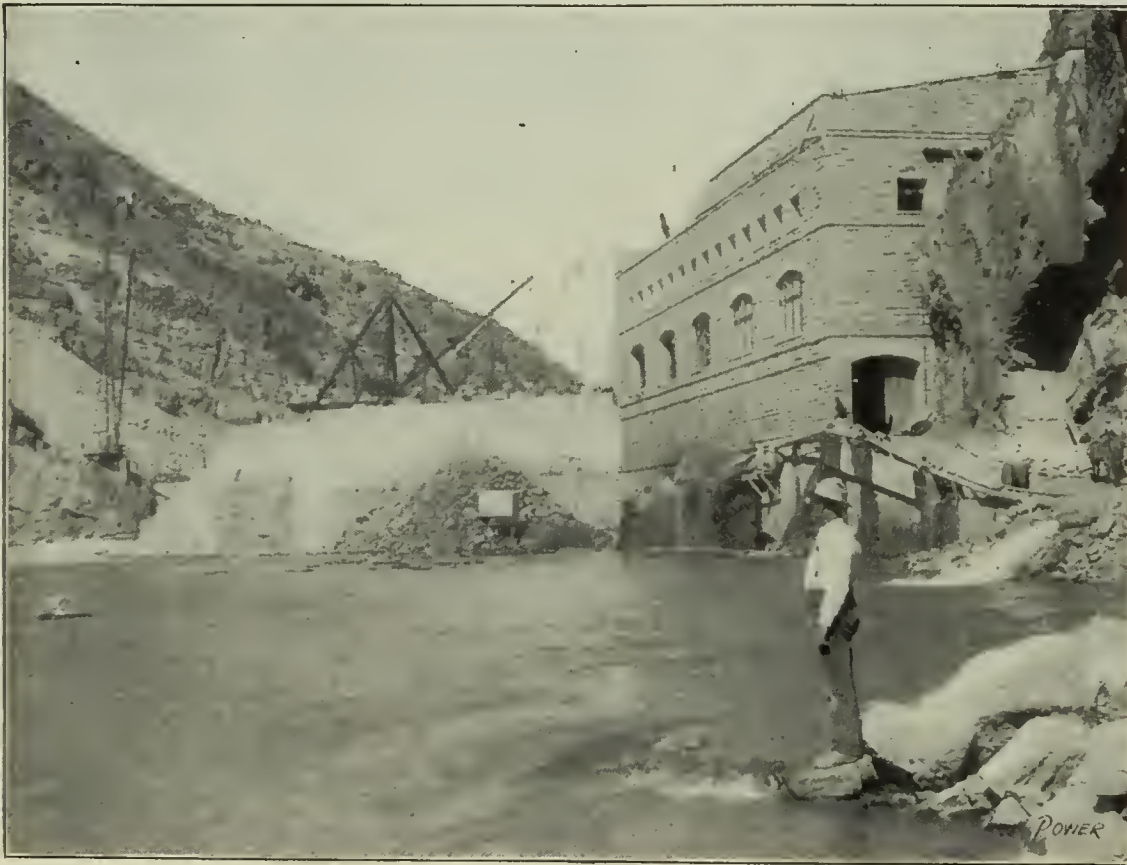
FIG. 1. DAM AND POWER HOUSE AT END OF CANAL
