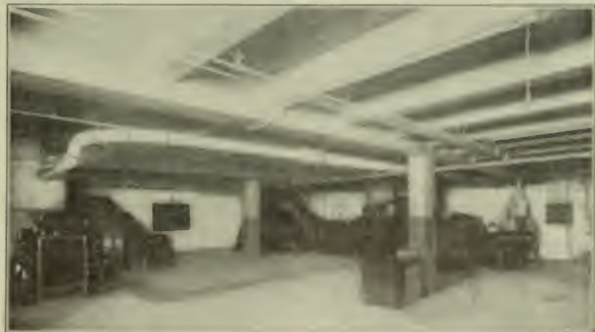
FIG. 4. ENGINE ROOM, SHOWING LARGE RECEIVERS
