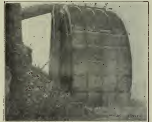
FIG. 2. WITH THE BUCKETS FULL OF WATER THE WHEEL REVOLVED TOWARD THE FOREGROUND
