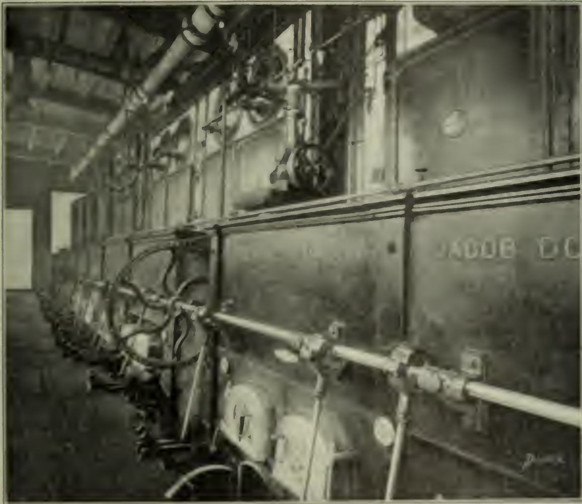
FIG. 1. MECHANISM FOR AUTOMATICALLY SHAKING THE GRATES
