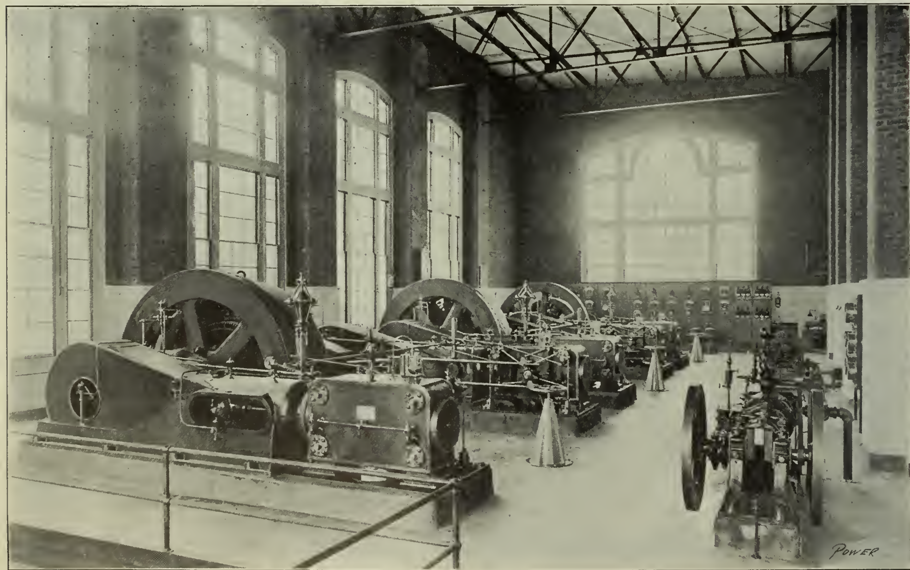
FIG. 1. VIEW OF THE ENGINE ROOM OF THE NEW POWER PLANT OF THE DENNISON MANUFACTURING COMPANY
