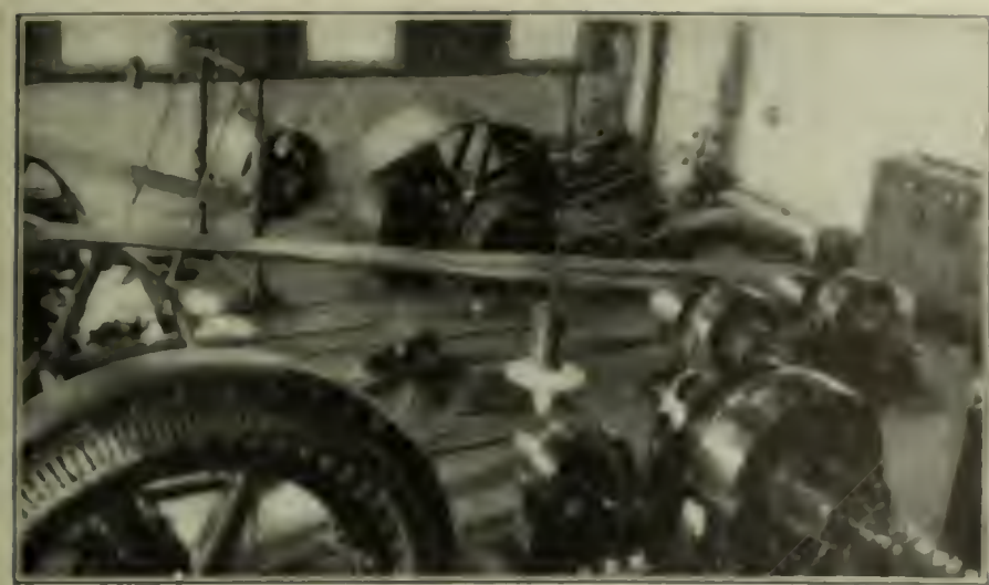
FIG. 5. OLD WAUSAU PLANT
