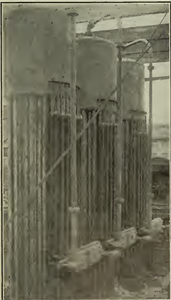
FIG. 20. WICKES VERTICAL BOILER AND FOSTER SUPERHEATER
