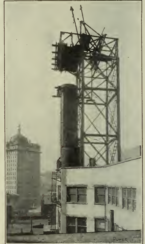
FIG. 2. TOWER IN PROCESS OF CONSTRUCTION
