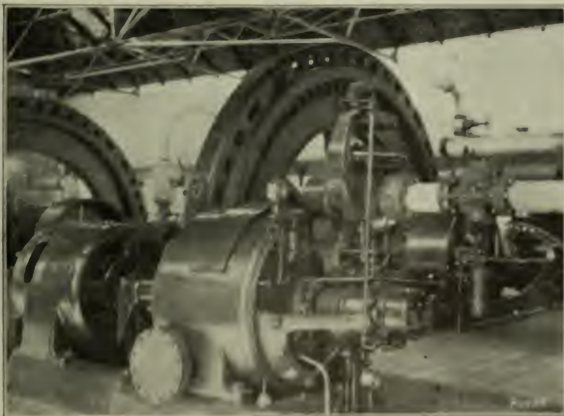
FIG. 1. EXCITER UNIT WITH AUTOMATIC CONTROL
