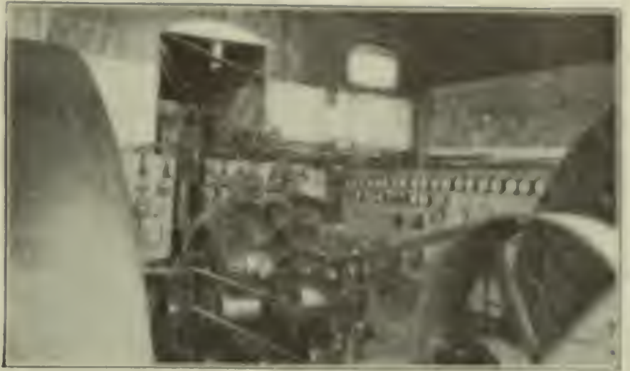
FIG. 6. SWITCHBOARD CONTROL OF OLD PLANT
