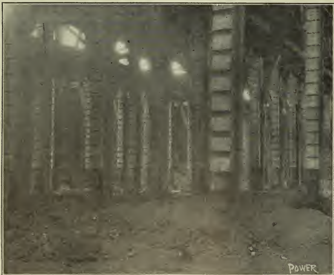
FIG. 4. SHOWING CONSTRUCTION OF VENTILATING CHUTES
