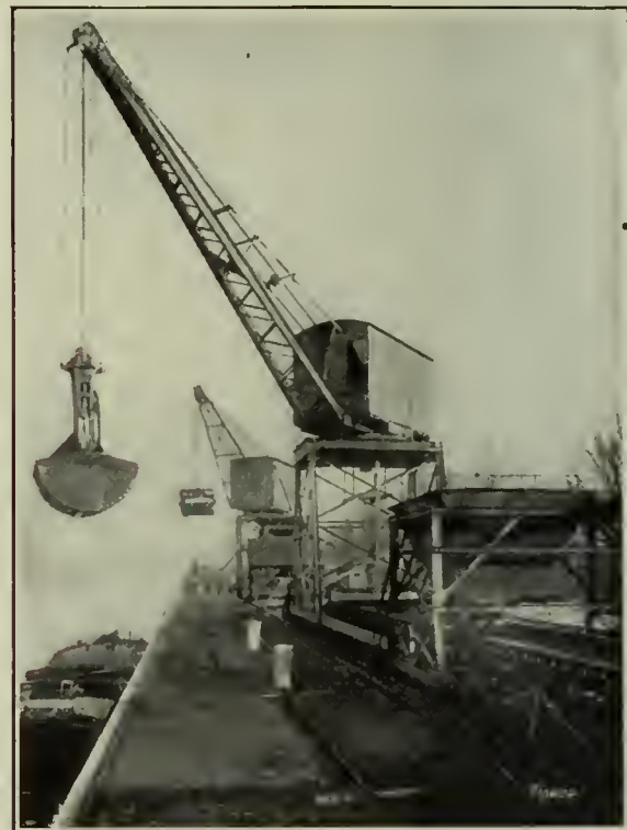
FIG. 3. METHOD OF UNLOADING BARGES
