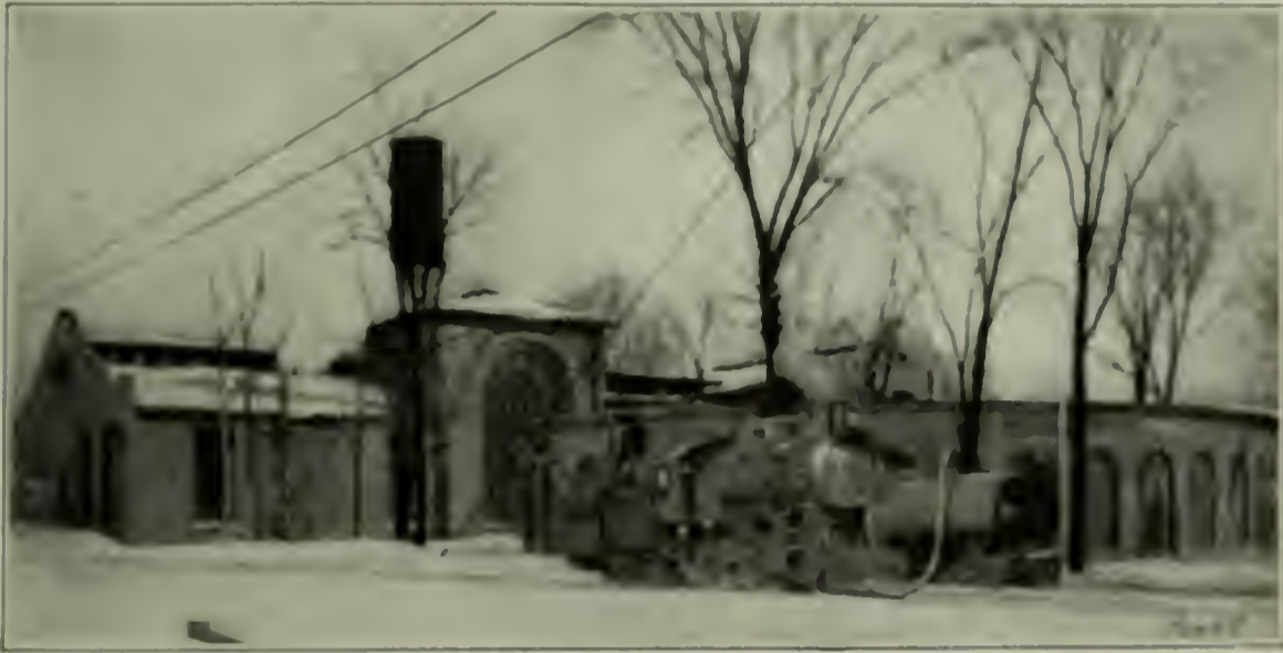
FIG. 1. LOCOMOTIVE PUMPING AIR INTO TANK CAR, FORCING WATER INTO THE RESERVOIR
