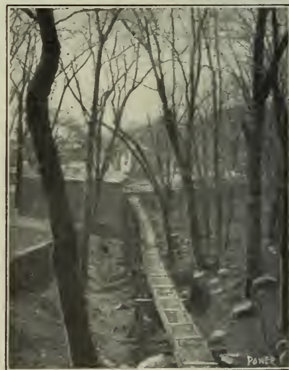
FIG. 2. SLUICWAY RUNNING FROM THE DAM TO THE WATERWHEEL
