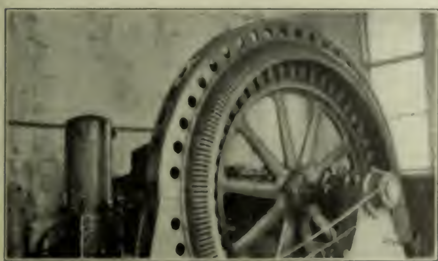
FIG. 7. MAIN GENERATOR IN NEW WAUSAU PLANT
