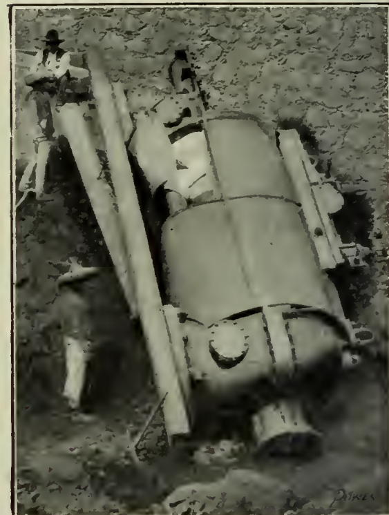
FIG. 2. BROKEN PLATFORM AND LAGGING
