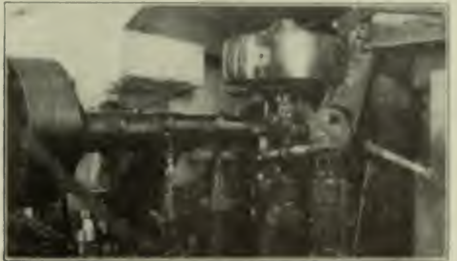
FIG. 8. OIL-PRESSURE GOVERNOR OF MAIN UNIT
