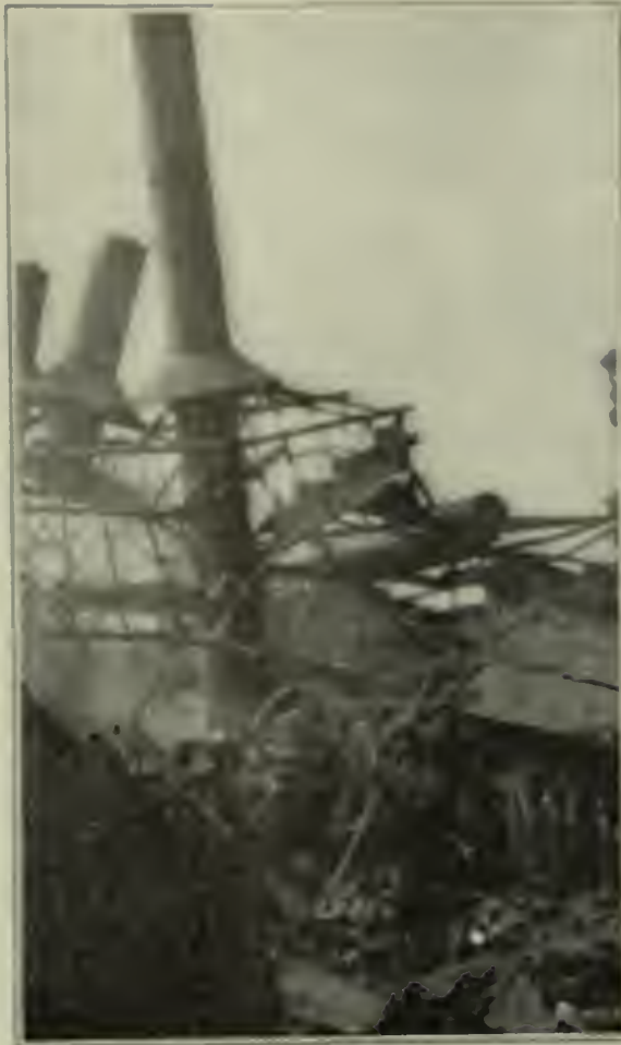
FIG. 2. DAMAGE TO STEELWORK AND STACKS
