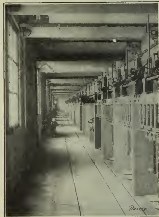
FIG. 8. SWITCH COMPARTMENTS
