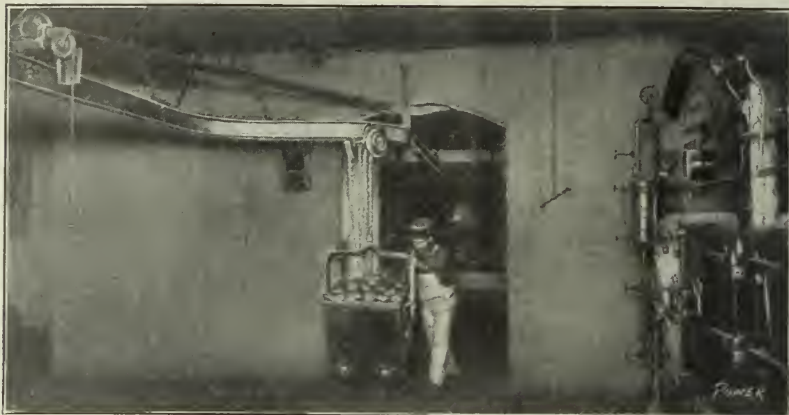
FIG. 2. HOIST PICKING UP ASH CAN
