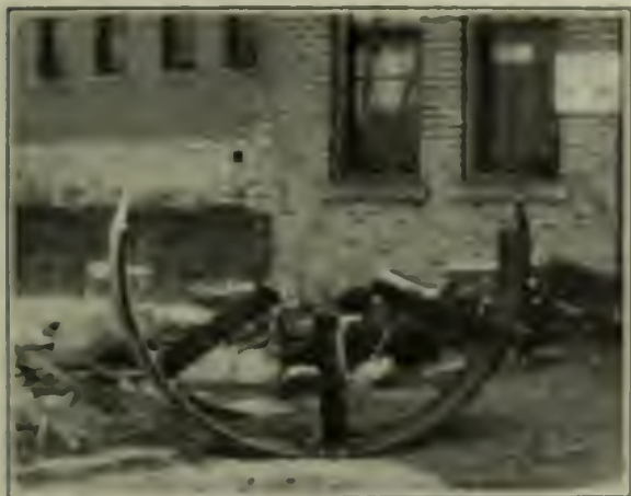
FIG. 4. PART OF BANDWHEEL WITH PIECE OF FLYWHEEL IN BACKGROUND
