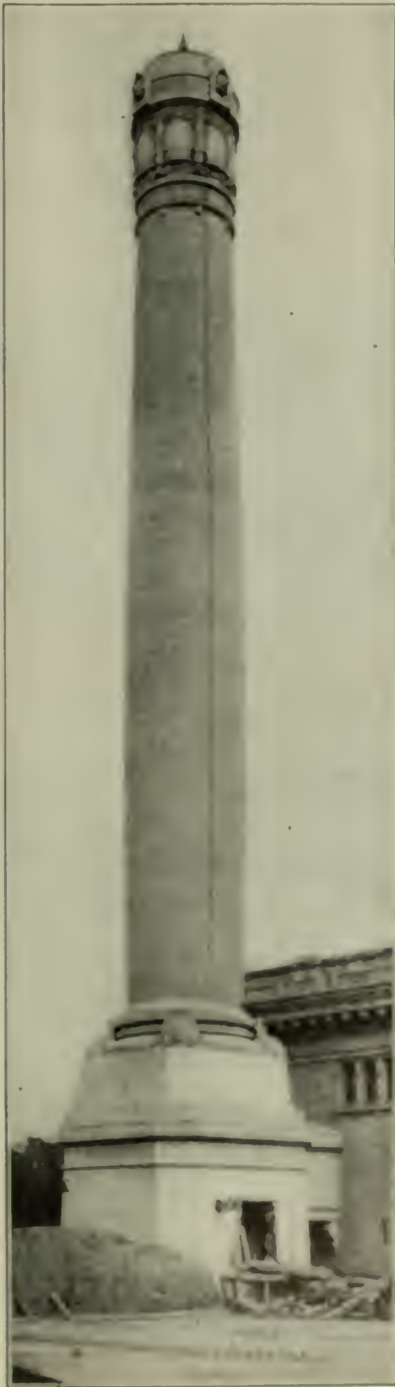
CHIMNEY AT QUEEN LANE FILTER PLANT, PHILADELPHIA
