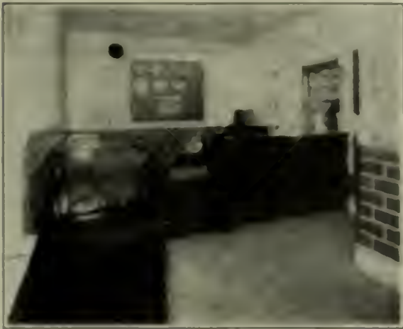
FIG. 11. ENGINEER'S OFFICE AT POWER HOUSE
