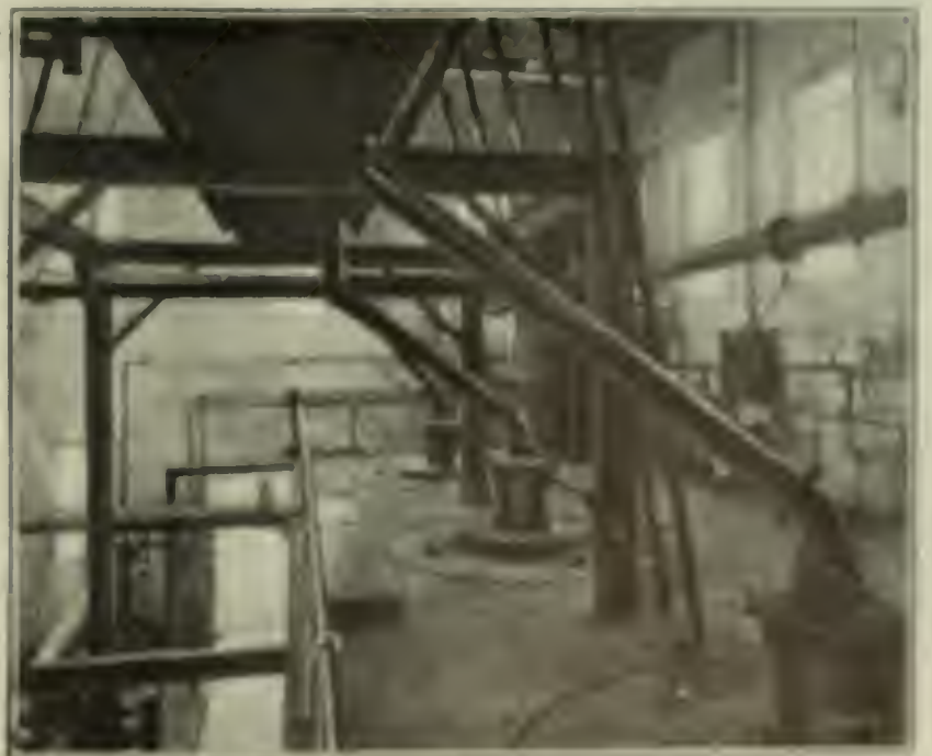
FIG. 2. THE CHARGING FLOOR
