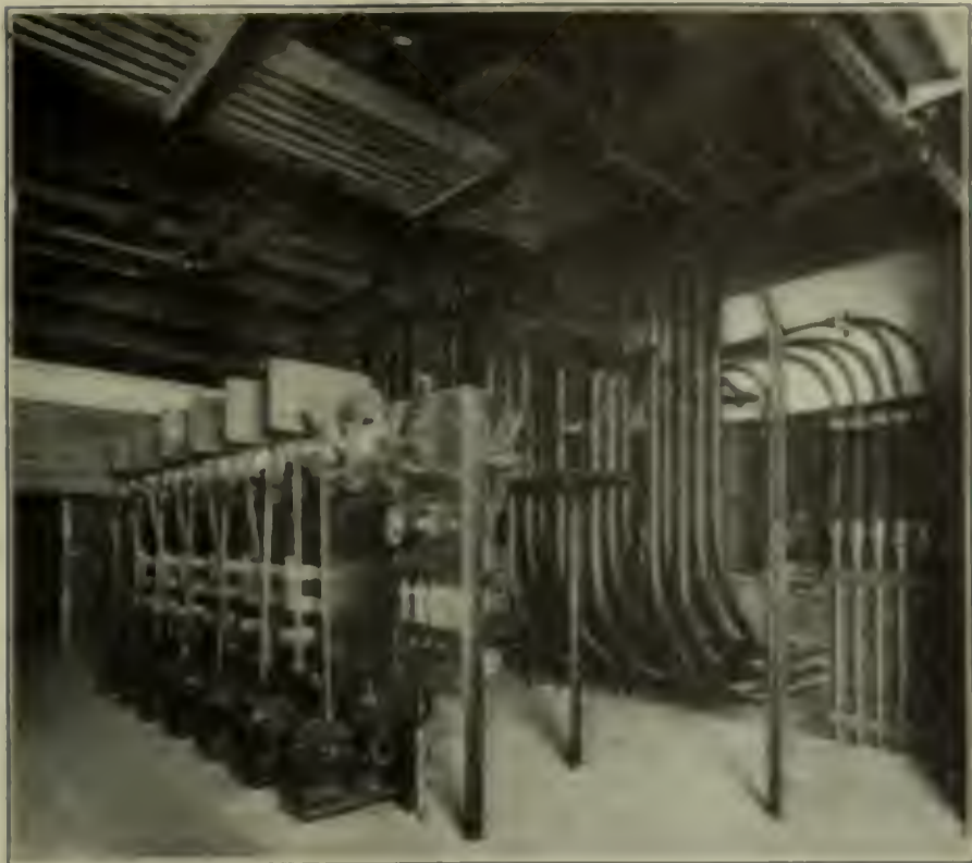
FIG. 4. DIRECT-CURRENT SWITCHBOARD
