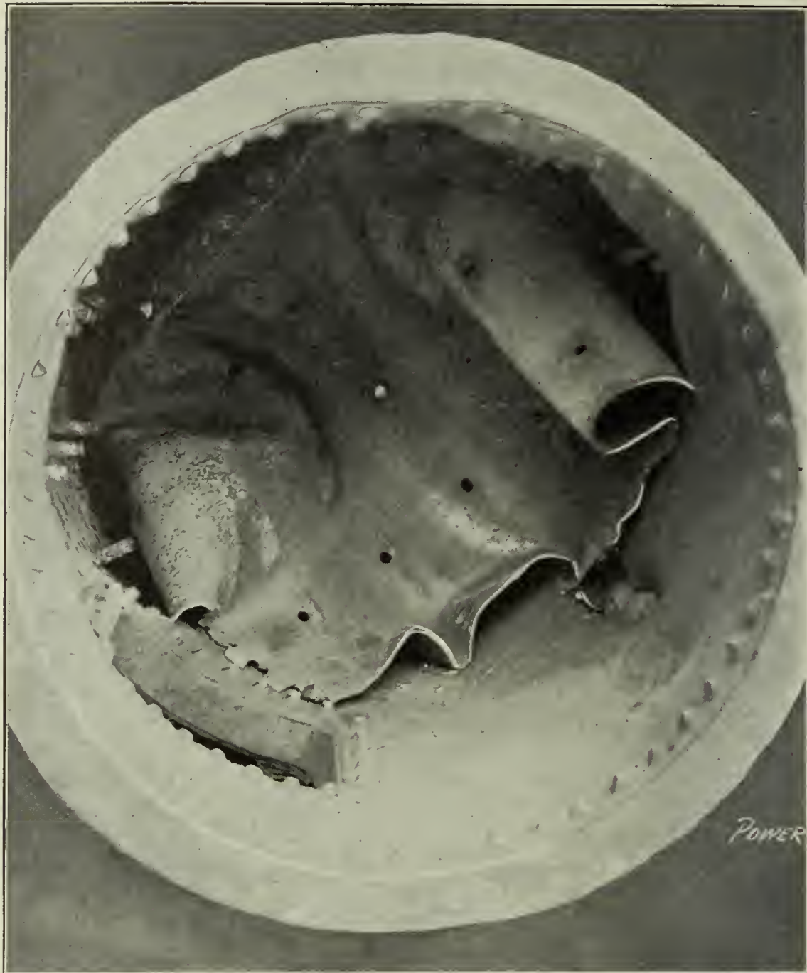
FIG. 3. INTERIOR OF FIREBOX AFTER EXPLOSION
