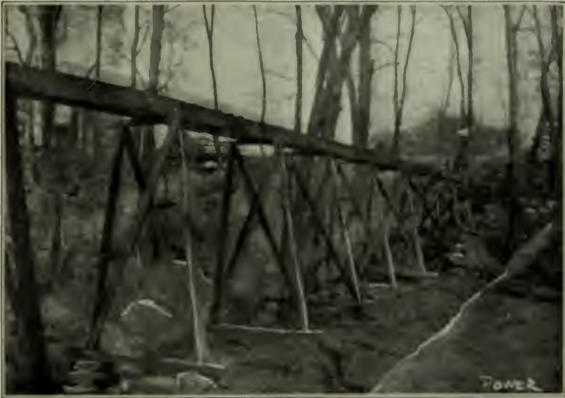
FIG. 3. SLUICWAY AND SUPPORTING TIMBERS
