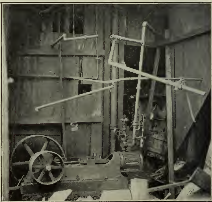
FIG. 2. DAMAGE TO ENGINE ROOM
