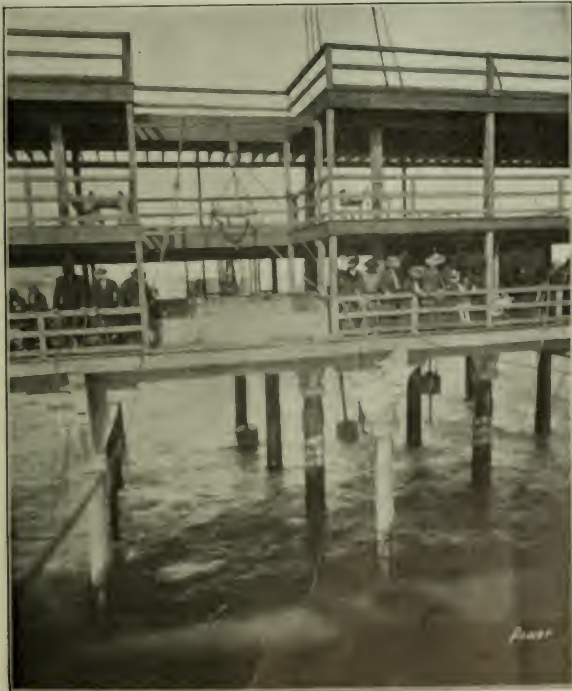
FIG. 2. THREE OF THE FLOATS WHICH ACTUATE THE MACHINERY.
