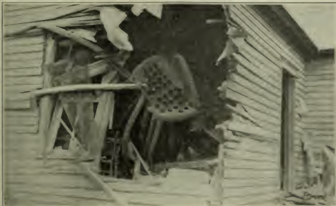
FIG. 1. HEAD AND TUBES HURLED THROUGH KITCHEN WALL
