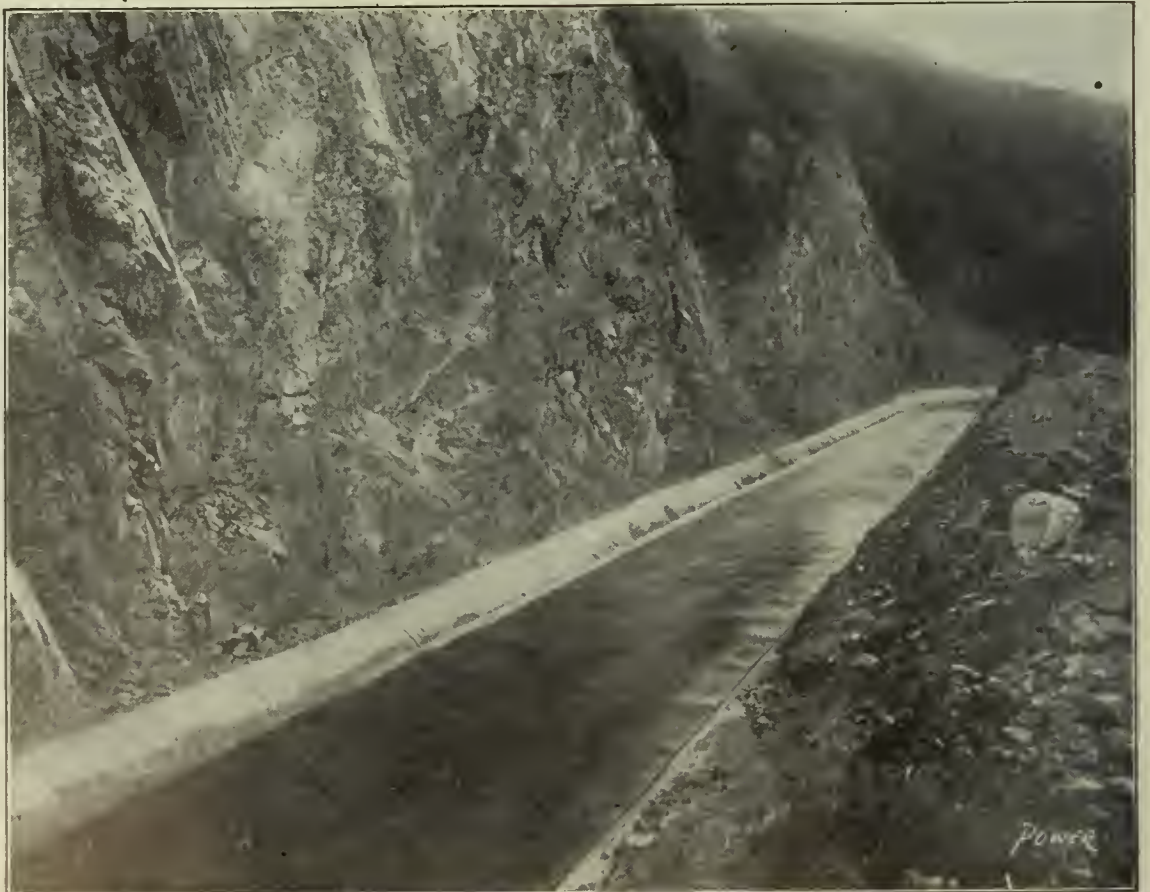
FIG. 2. PART OF 20-MILE CANAL FROM SALT RIVER TO POWER STATION
