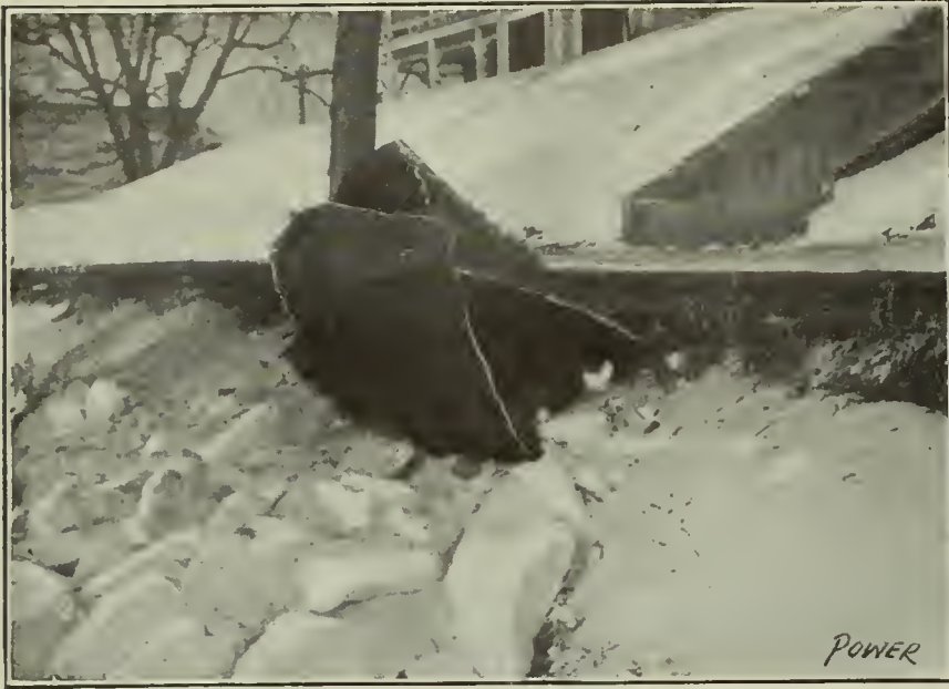
FIG. 4. SECTION OF SHELL THROWN 350 FEET
