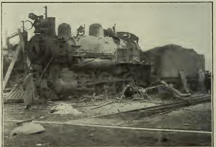
FIG. 3. DAMAGE TO ENGINE NEARBY
