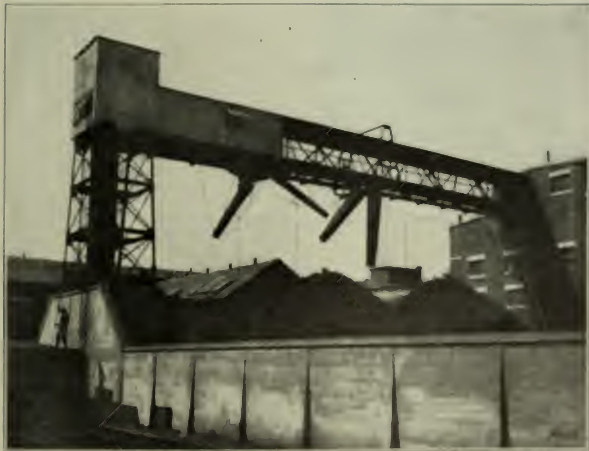
FIG. 8. COAL CONVEYER AND COAL STORAGE YARD
