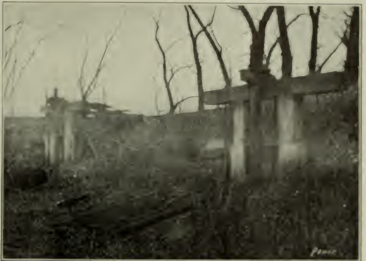
FIG. 5. ALL THAT IS LEFT OF THE OLD GATE CONTROL
