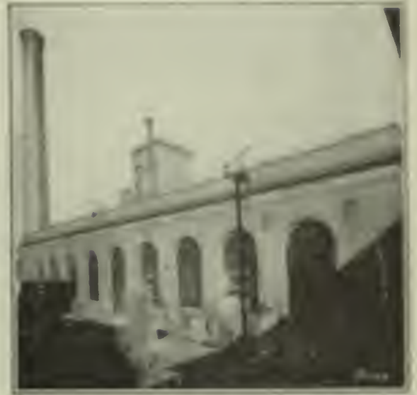
FIG. 7. POWER HOUSE OF NORTHSHORE TERMINAL
