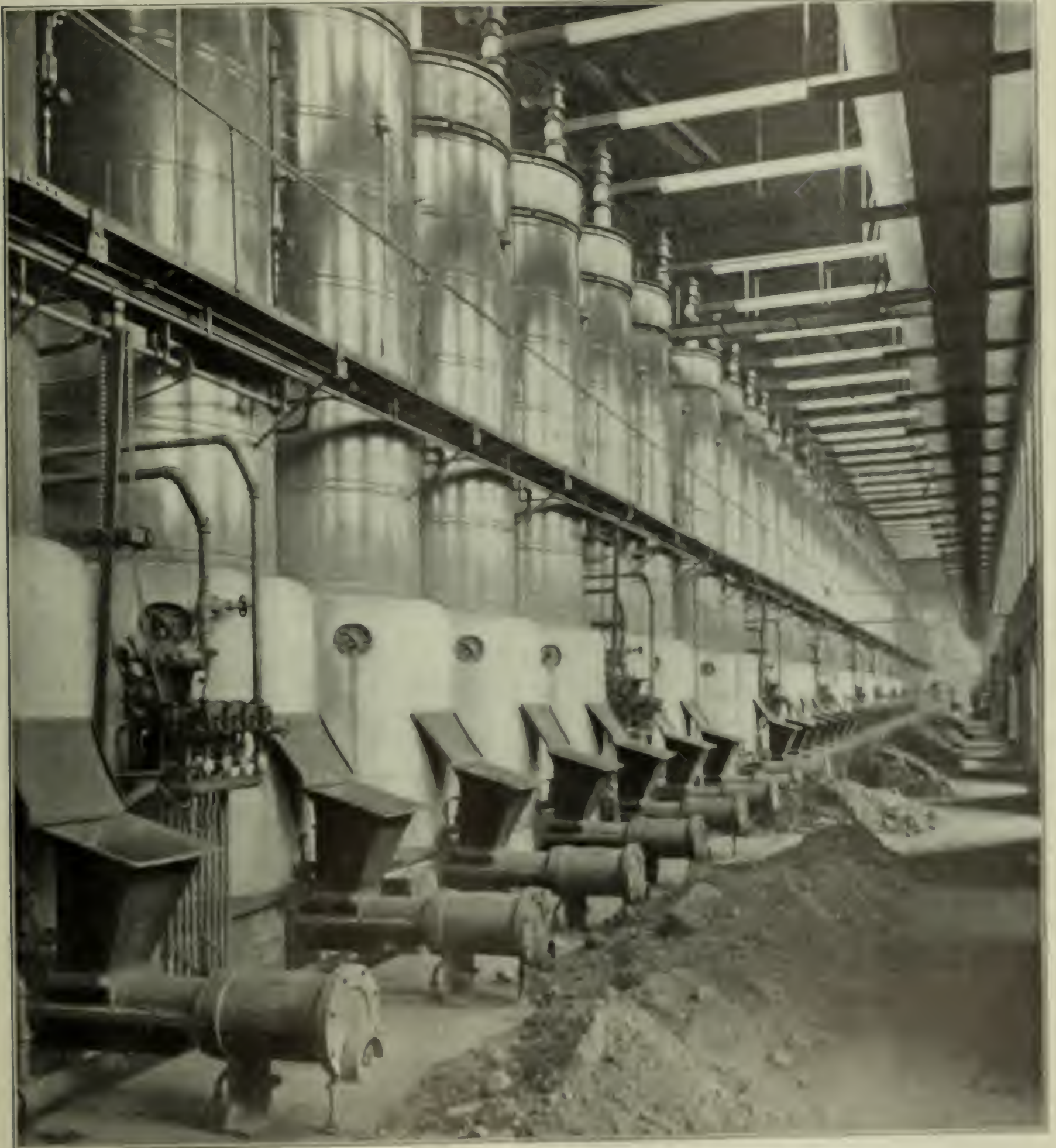
FIG. 2. THE SIXTY-FIVE MARRIOTT BOLLES SYSTEM UNIT FROM BUREAU
