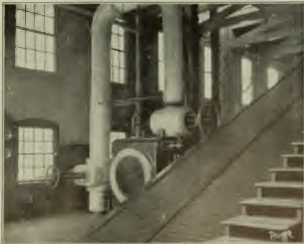
FIG. 2. DOUBLE THROTTLE VALVE AND STEAM TRUNK.
