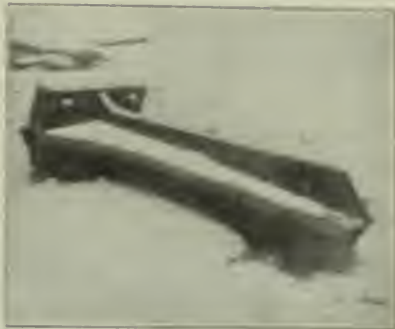
FIG. 2. PIECE OF WHEEL ON ROOF AND HOLE THROUGH WHICH IT CAME
