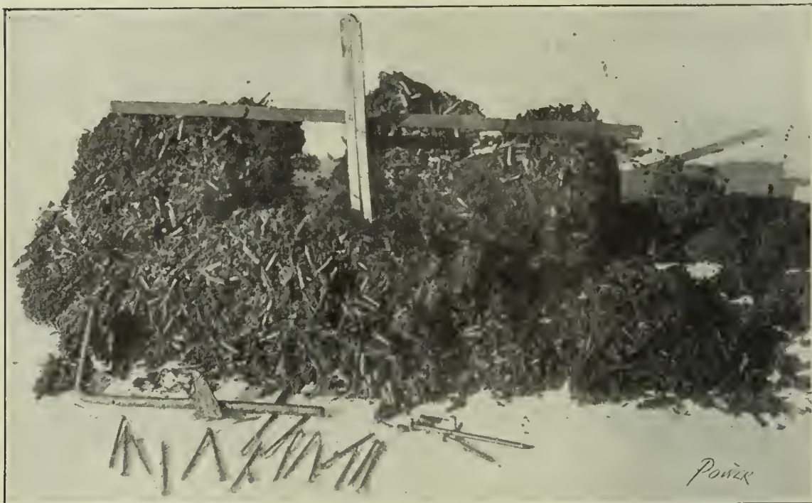
FIFTY-NINE POUNDS OF JUNK TAKEN FROM LOW-PRESSURE CYLINDER
