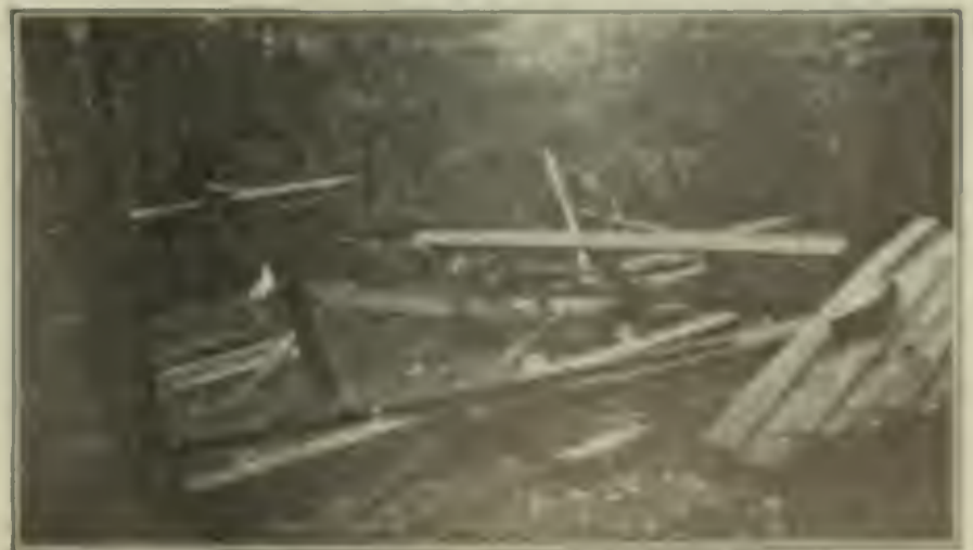
FIG. 2. REMAINS OF BOILER
