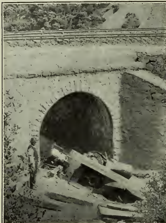
FIG. 1. SHOWING WHERE THE TURBINE LANDED
