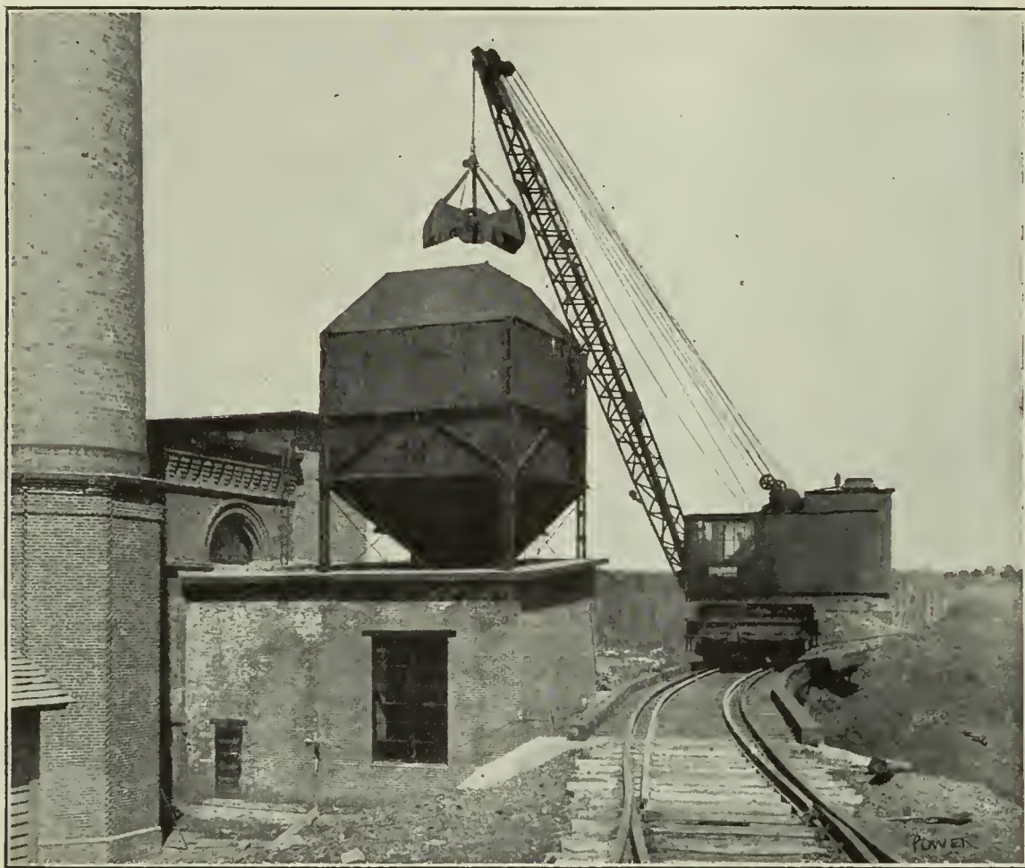
FIG. 4. COAL-HANDLING TRAVELING LOCOMOTIVE
