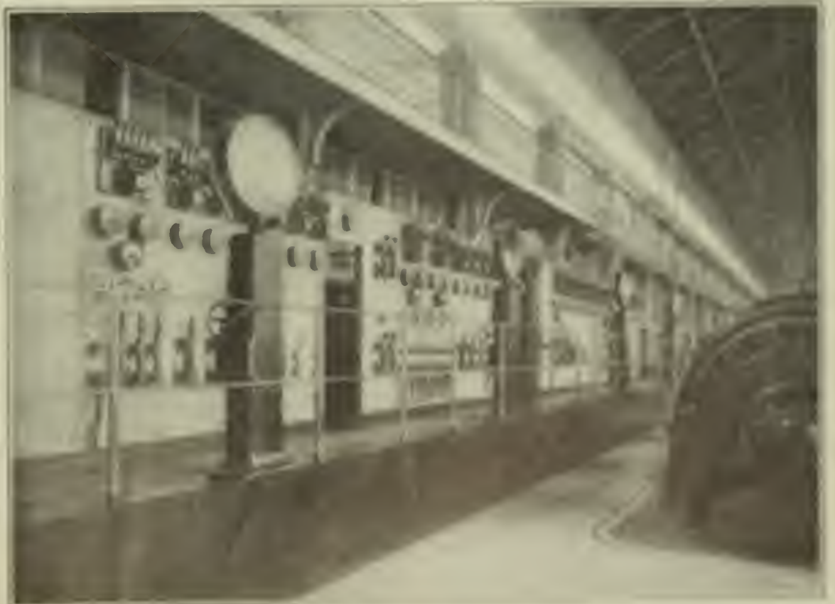
FIG. 11. LOW-TENSION SWITCHBOARD
