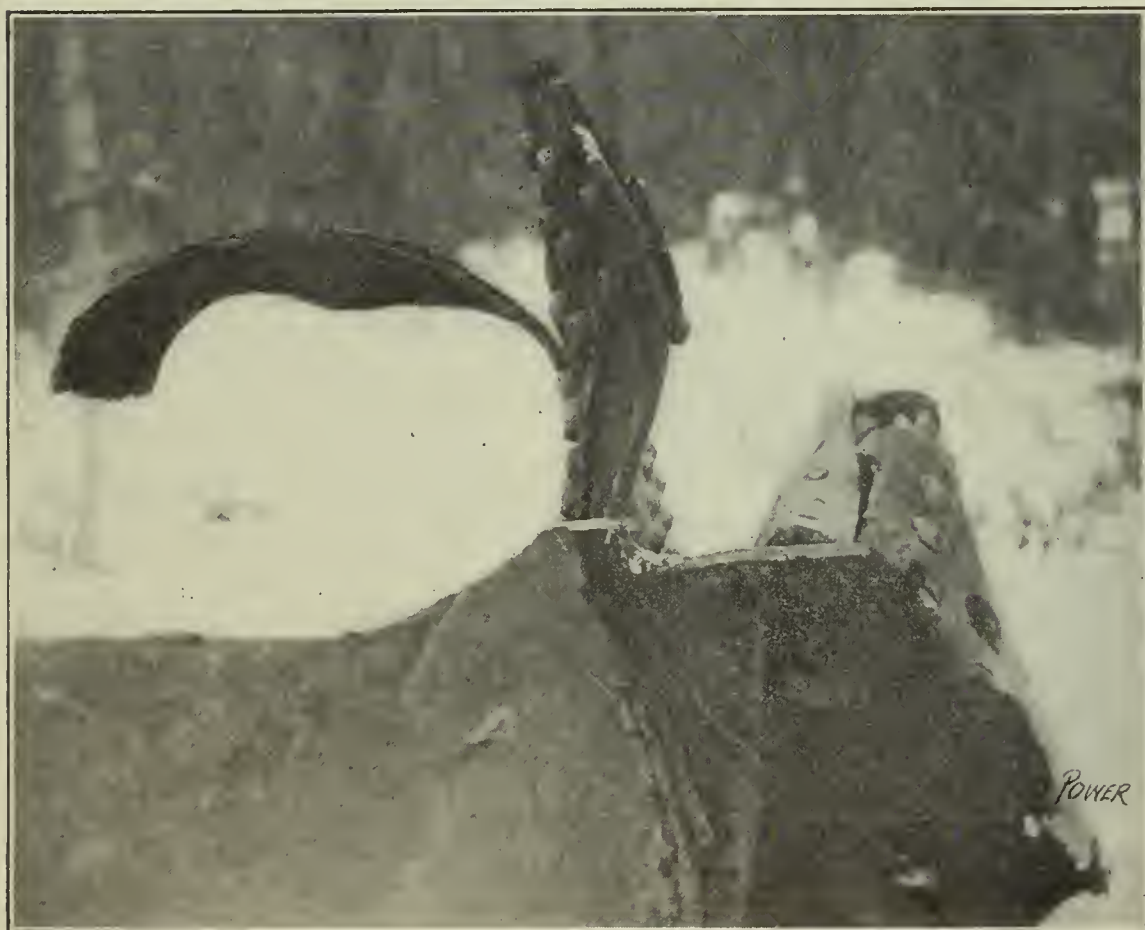
FIG. 4. PART OF MIDDLE COURSE WITH PART OF WATER LEG
