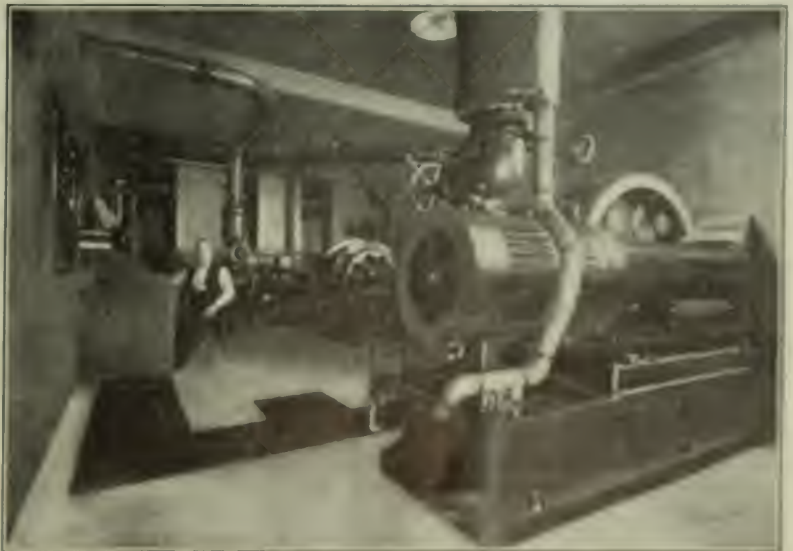
FIG. 5. GENERAL VIEW OF ENGINE ROOM
