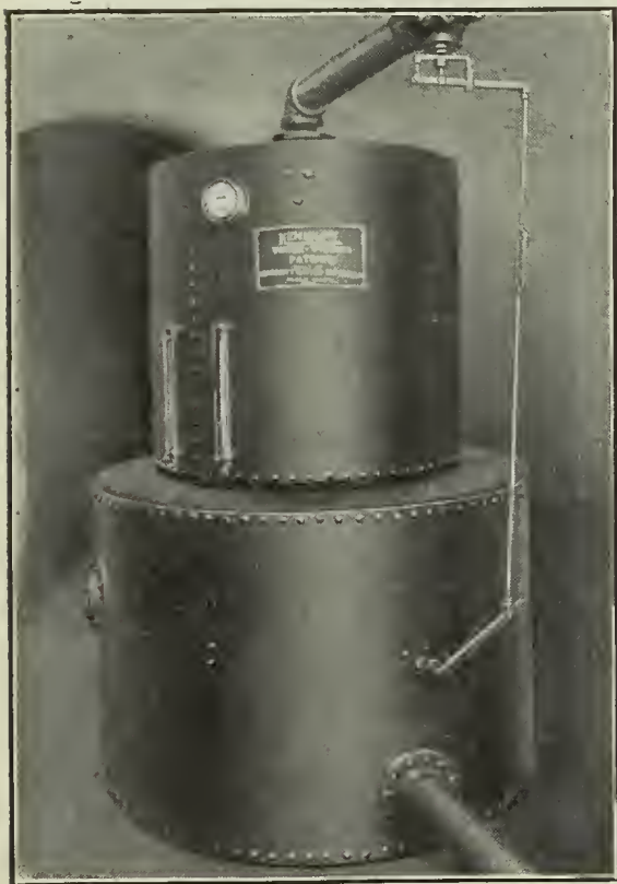
FIG. 3. WEIGHER AND ATTACHED STORAGE TANK
