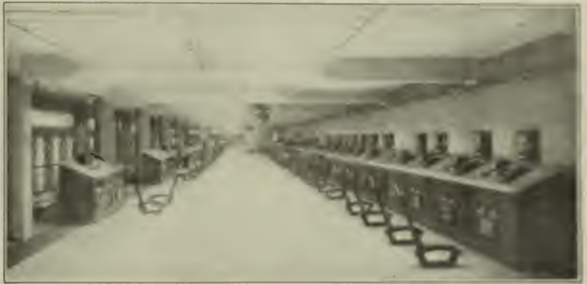
FIG. 10. GALLERY CONTAINING REMOTE-CONTROL MACHINERY
