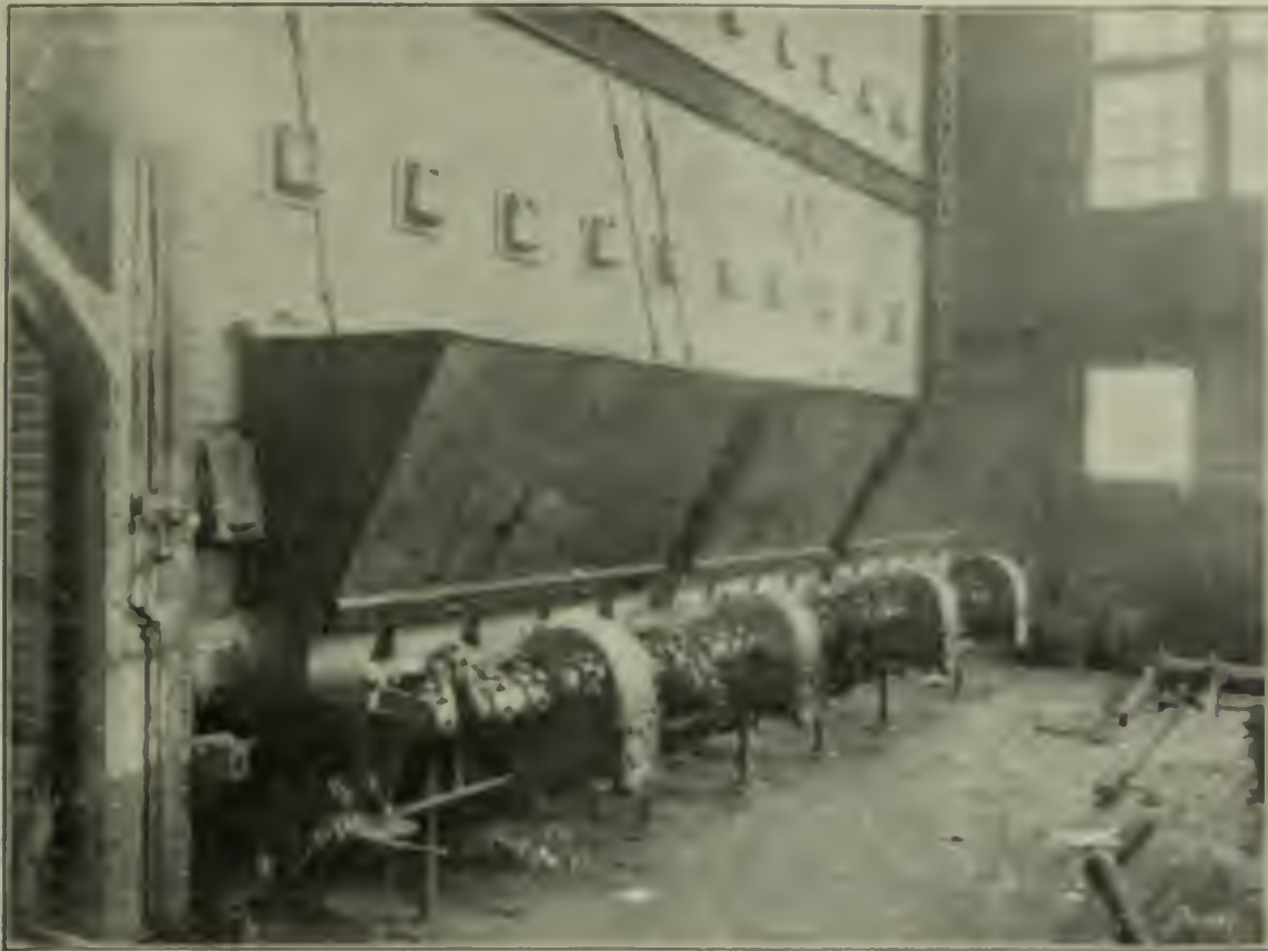
FIG. 2. FRONT OF BOILERS SHOWING STOKER
