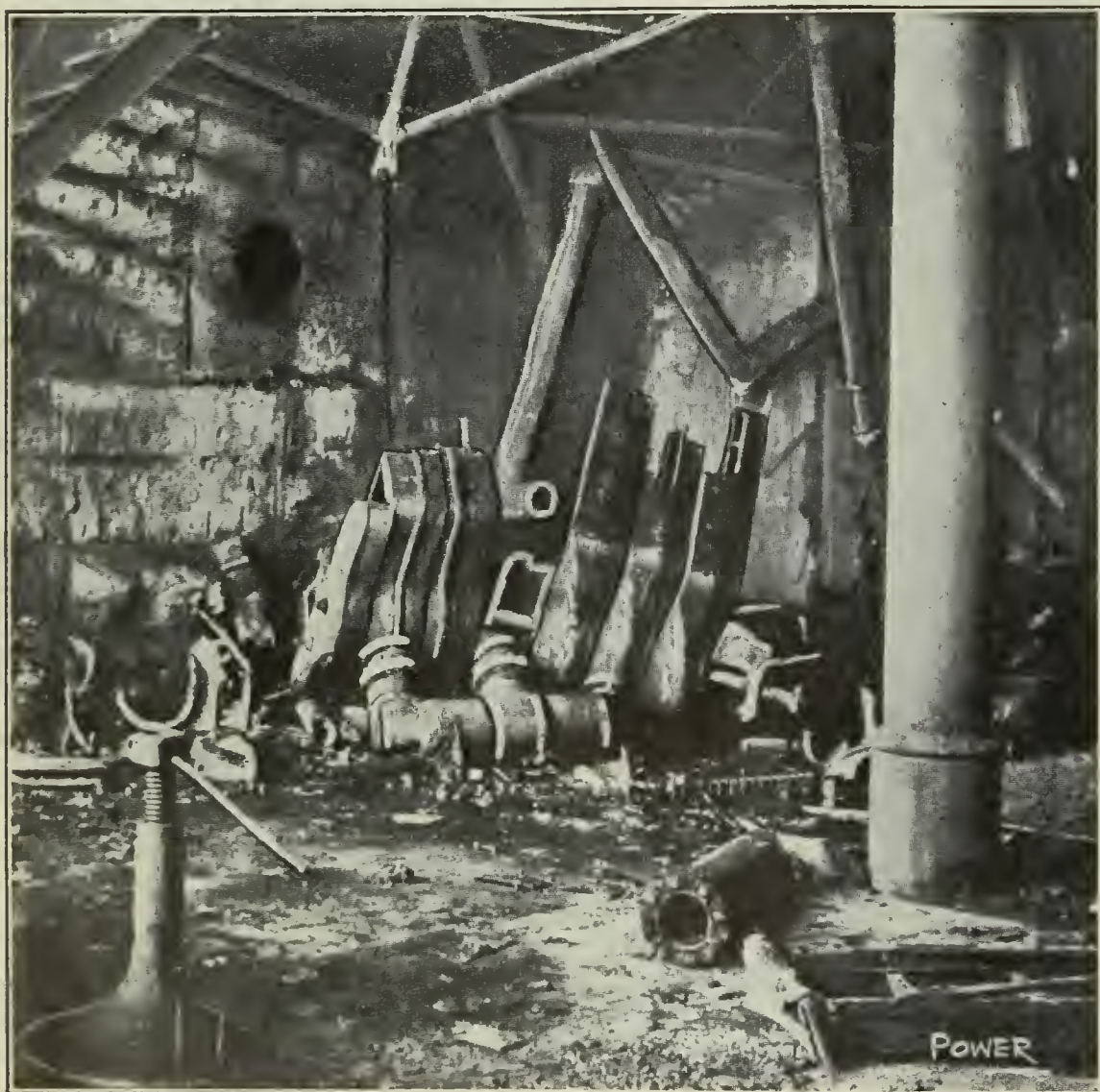
REMAINS OF HEATING BOILER WHICH KILLED TWO MEN
