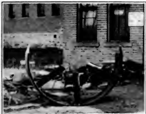
FIG. 4. PART OF BANDWHEEL WITH PIECES OF FLYWHEEL IN BACKGROUND
