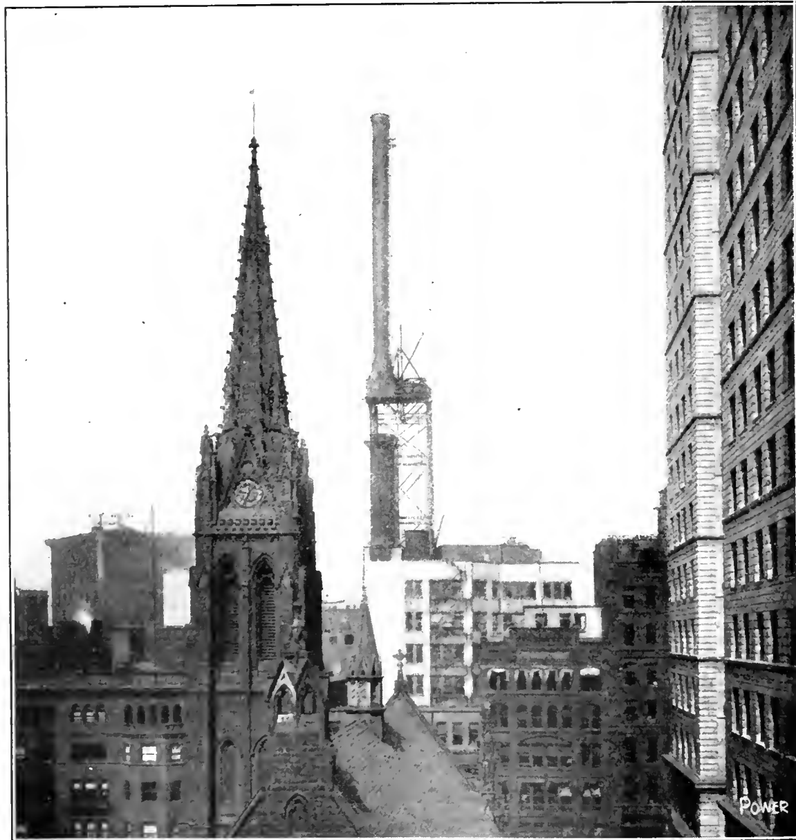
FIG. 1. NEW STACK IN PLACE WITH 18-FOOT SECTION OF OLD STACK REMOVED
