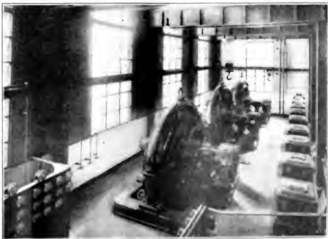
FIG. 15. ROTARY CONDENSER FOR THE REFRIGERATING SYSTEM.
