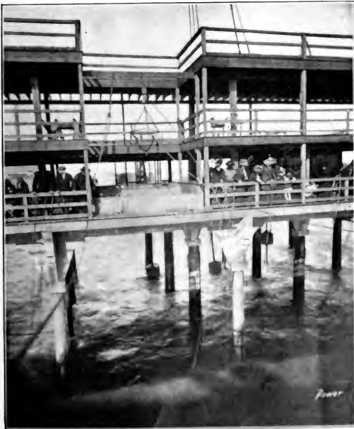
FIG. 2. THREE OF THE FLOATS WHICH ARE USED IN THE MECHANISM
