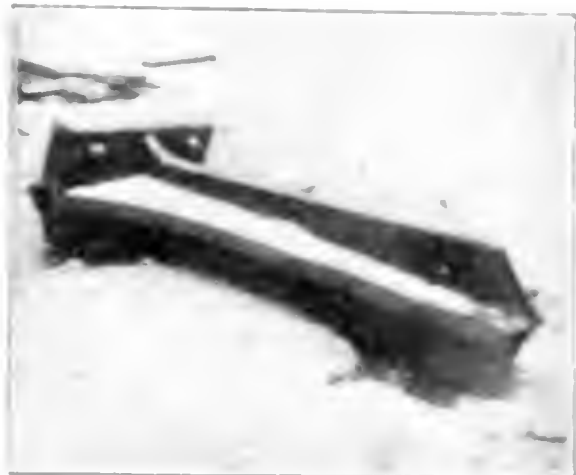
FIG. 2. PIECE OF WHEEL ON RIM AND HOLE THROUGH WHICH IT CAME.
