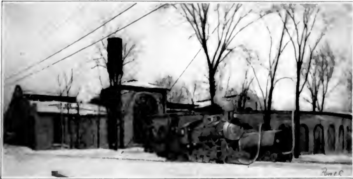
FIG. 1. LOCOMOTIVE PUMPING AIR INTO TANK CAR, FORCING WATER INTO THE RESERVOIR
