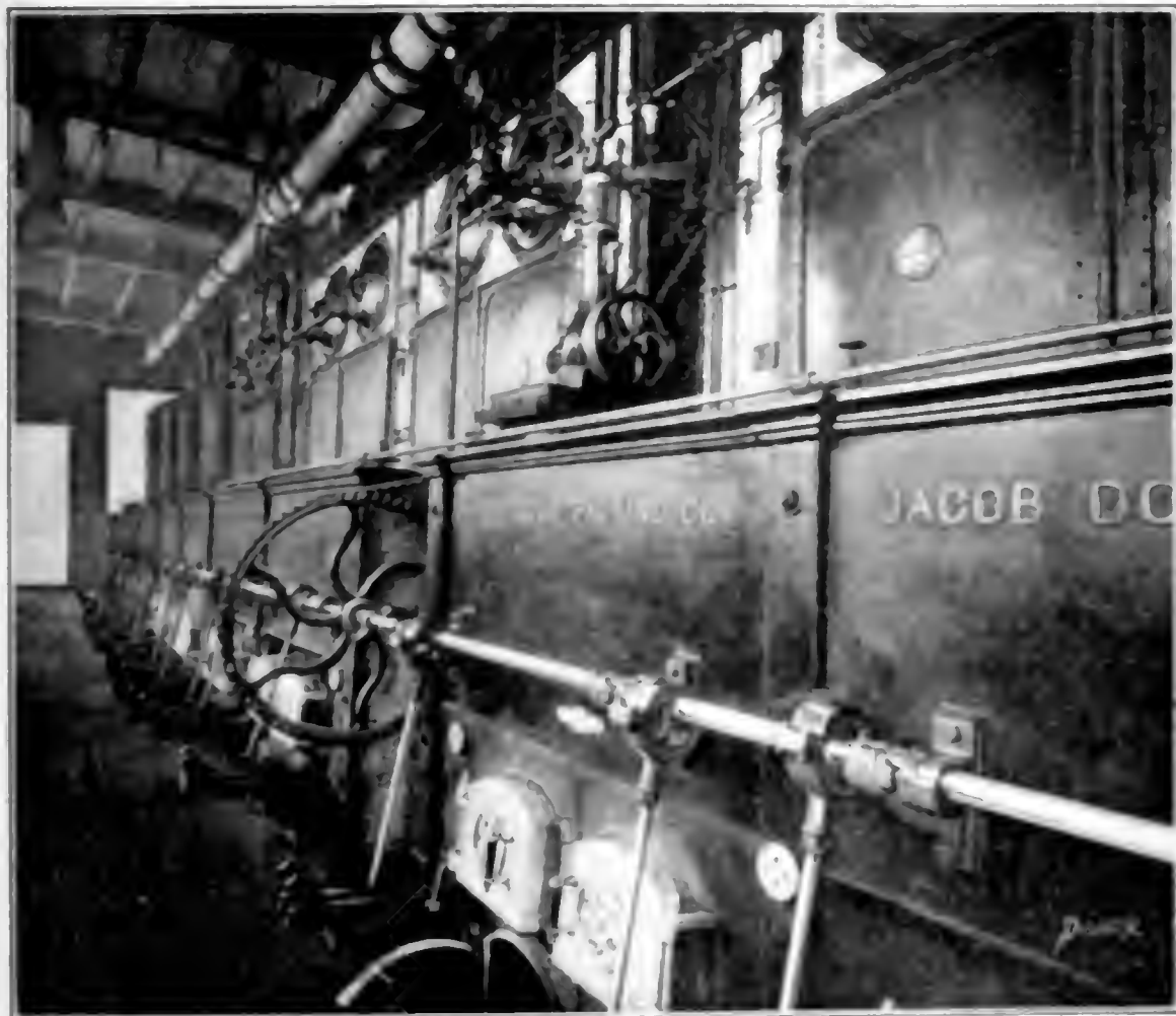
FIG. 1. MECHANISM FOR AUTOMATICALLY SHAKING THE GRATES.
