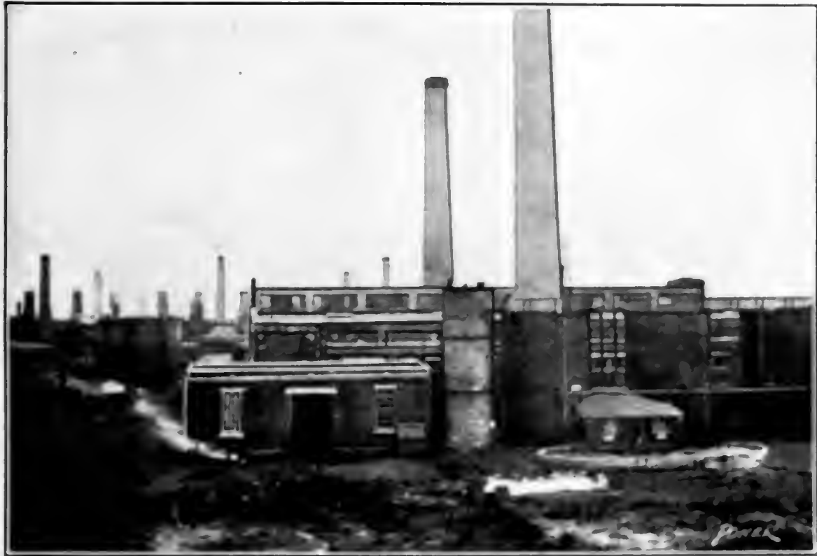
FIG. 3. GENERAL VIEW OF BOILER HOUSE, FAN HOUSE AND WATER-SOFTENING PLANT
