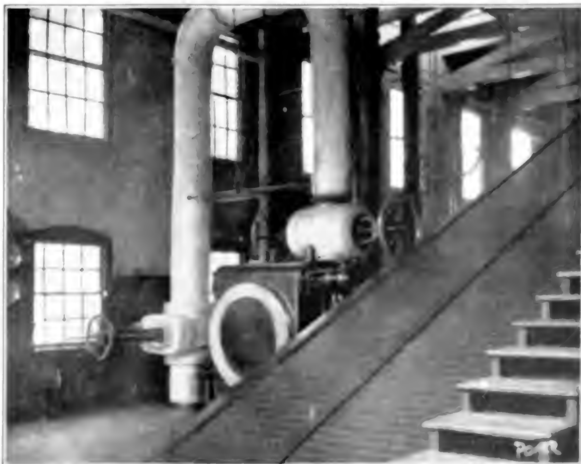
FIG. 2. DOUBLE THROTTLE VALVE ON RECIPROCATING ENGINE
