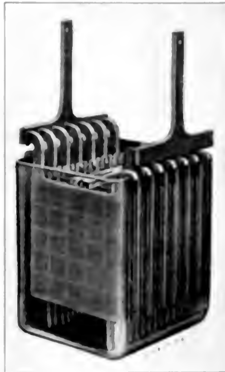
FIG. 2. CELL IN GLASS JAR
