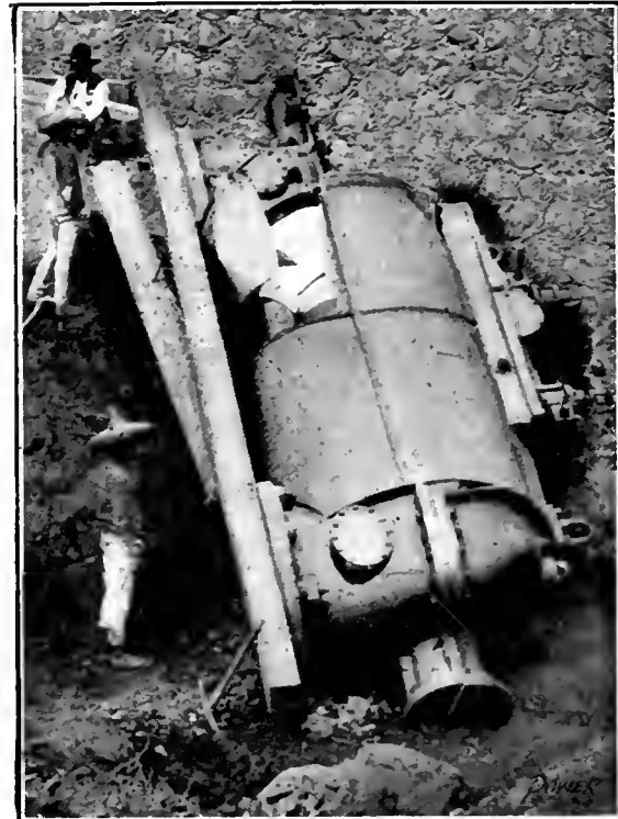
FIG. 2. BROKEN PLATFORM AND LAGGING
