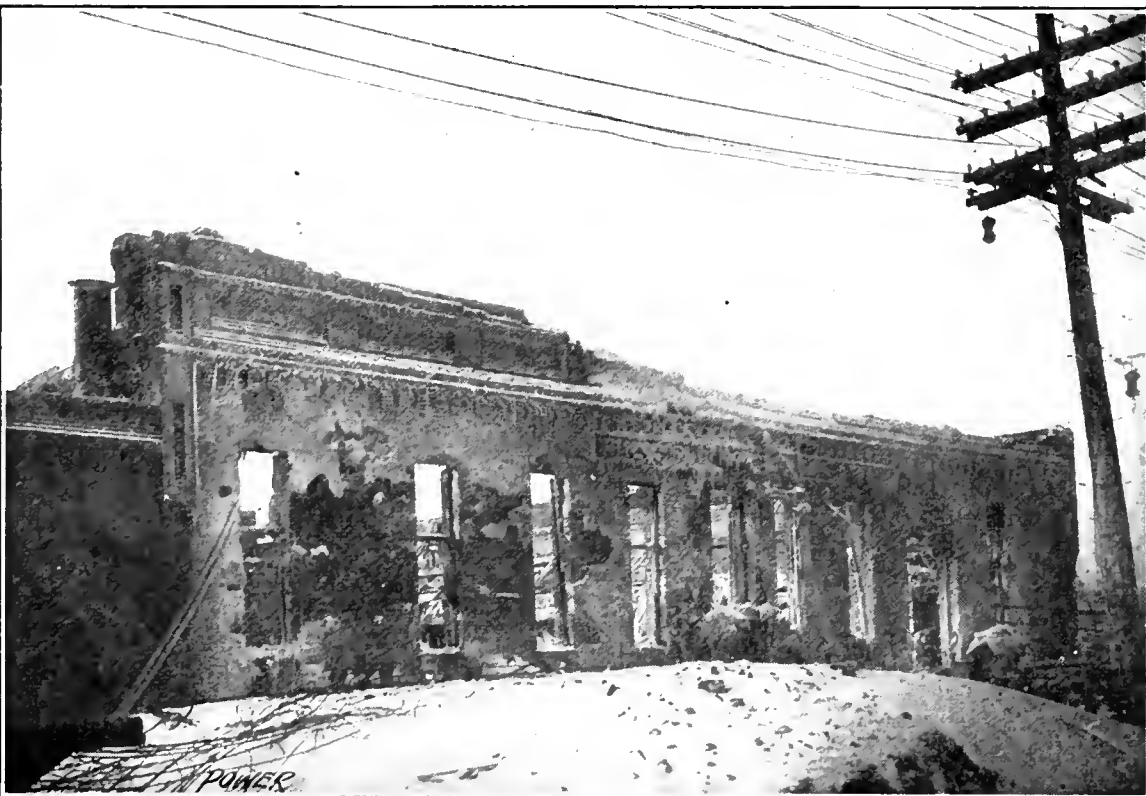
FIG. 2. REMAINS OF THE BUILDING
