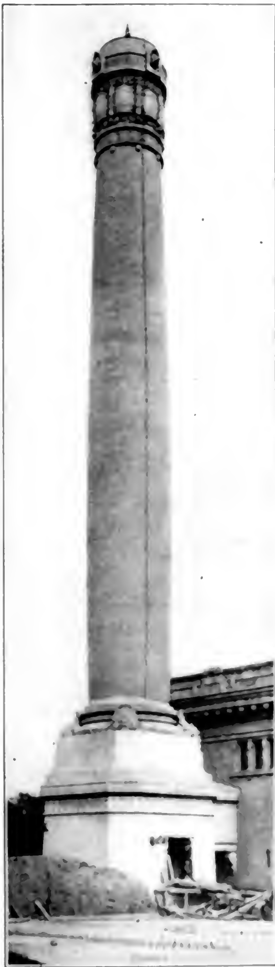
CHIMNEY AT QUEEN LANE FILTER PLANT, PHILADELPHIA
