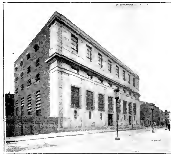
FIG. 3. EXTERIOR VIEW OF SERVICE PLANT
