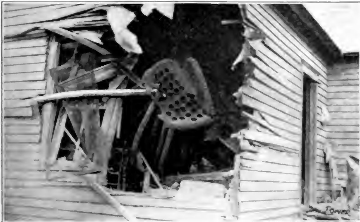
FIG. 1. HEAD AND TUBES HURLED THROUGH KITCHEN WALL
