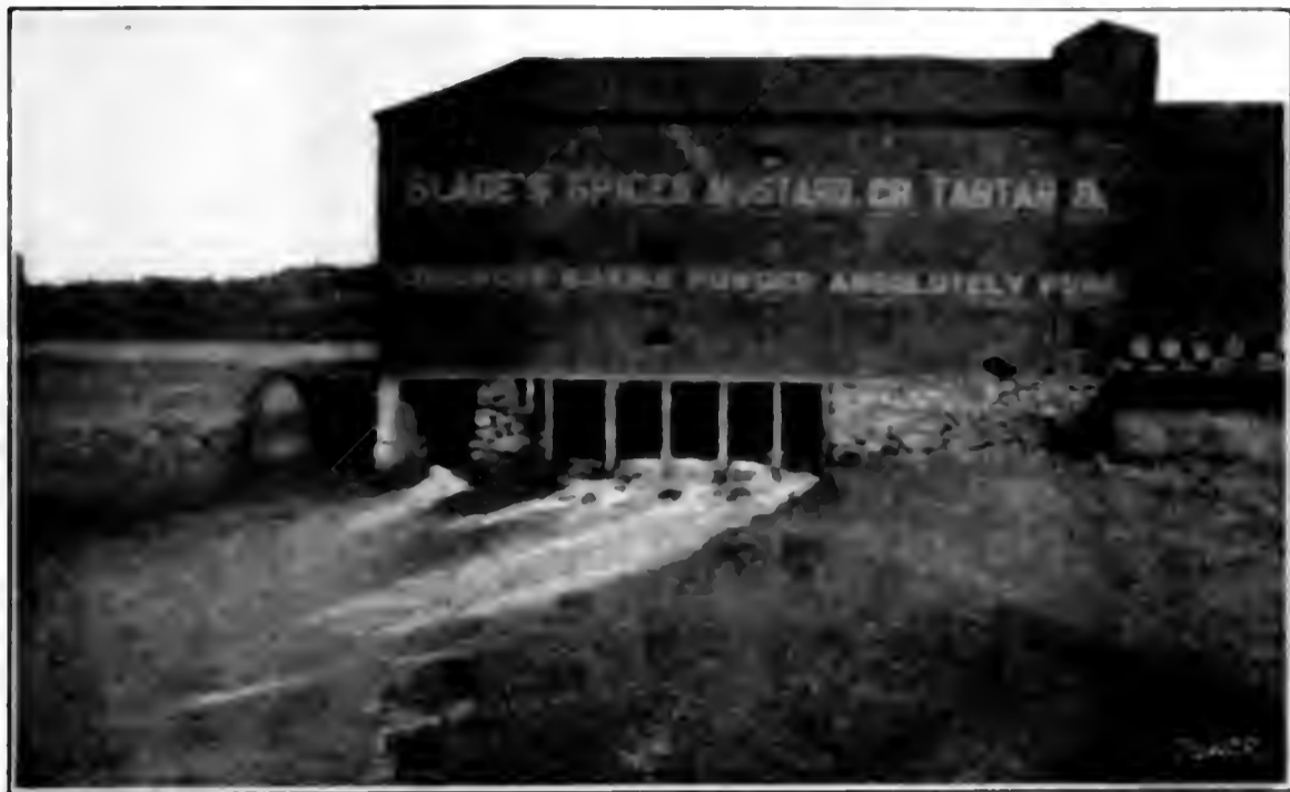
FIG. 1. SLADE'S TIDE MILL, SHOWING WATER FLOWING FROM THE WHEELS AT LOW TIDE
