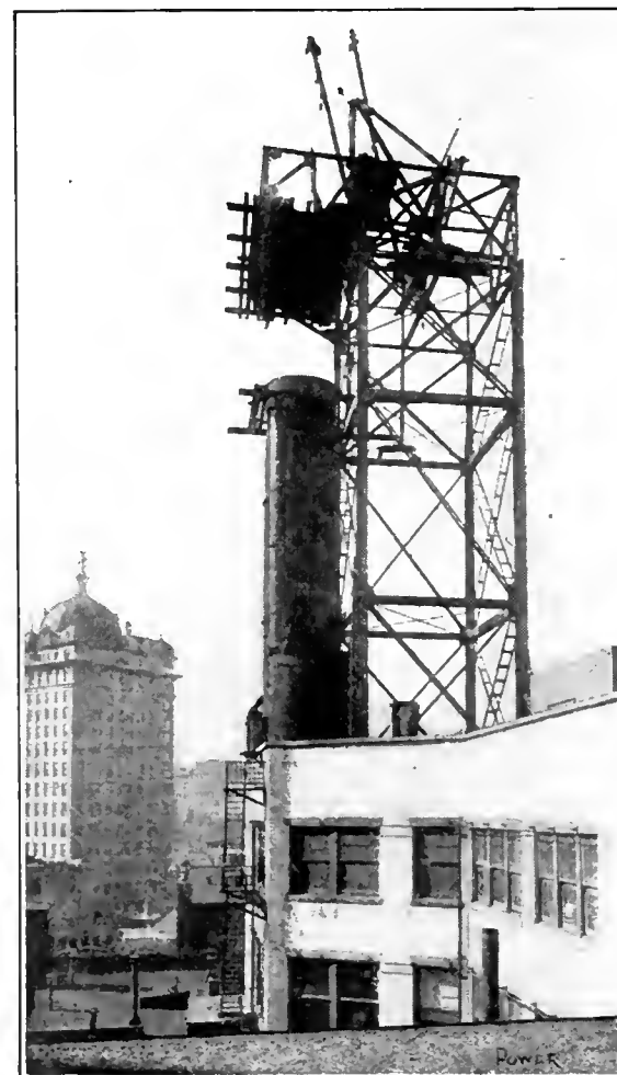
FIG. 2. TOWER IN PROCESS OF CONSTRUCTION
