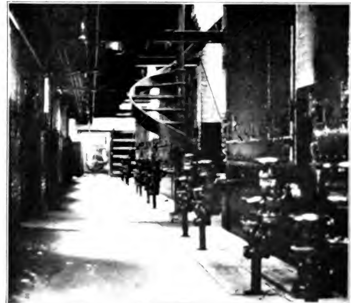
FIG. 4. VIEW OF DAMPER IN PLACE
