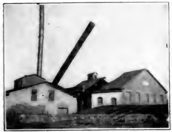
FIG. 1. TILTED IRON STACK
