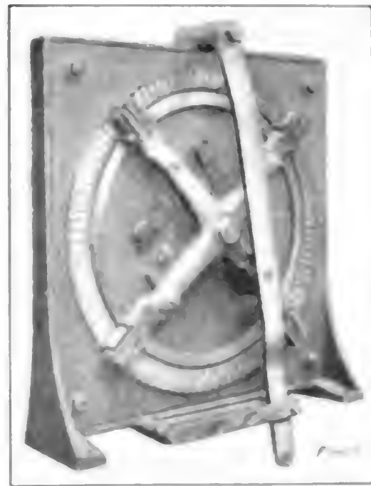
FIG. 12. CONTACT PLATE FOR A THREE-WAY CONTROLLER
