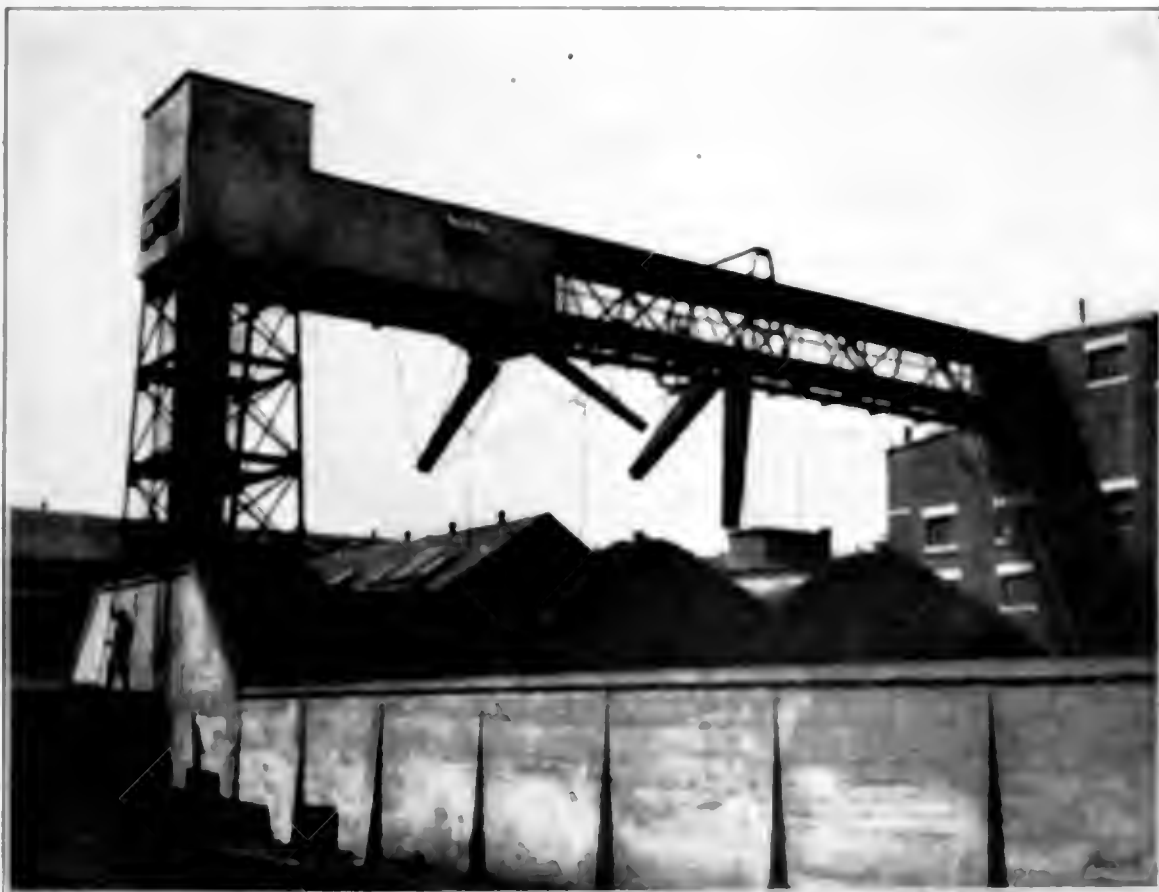
FIG. 8. COAL CONVEYER AND COAL STORAGE YARD.
