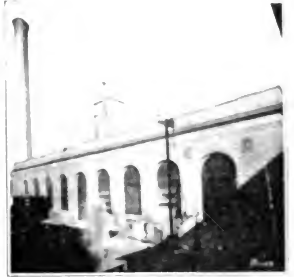
FIG. 7. THE BOILER ROOM. (Continued from page 10.)
