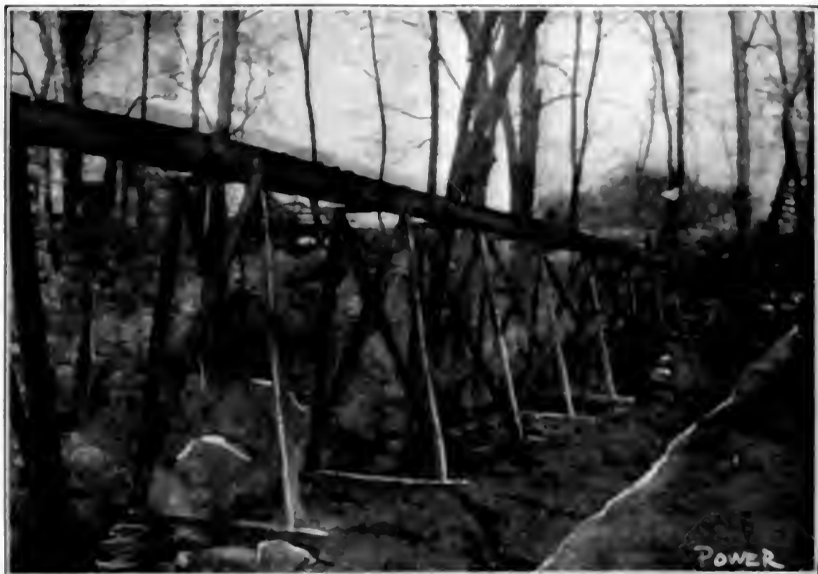
FIG. 3. SLUICWAY AND SUPPORTING TIMBERS
