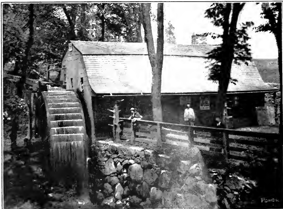
FIG. 1. THE OLD MILL AT NEW LONDON, BUILT IN 1650
