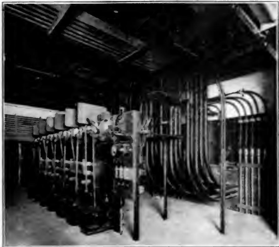
FIG. 4. DIRECT-CURRENT SWITCHBOARD
