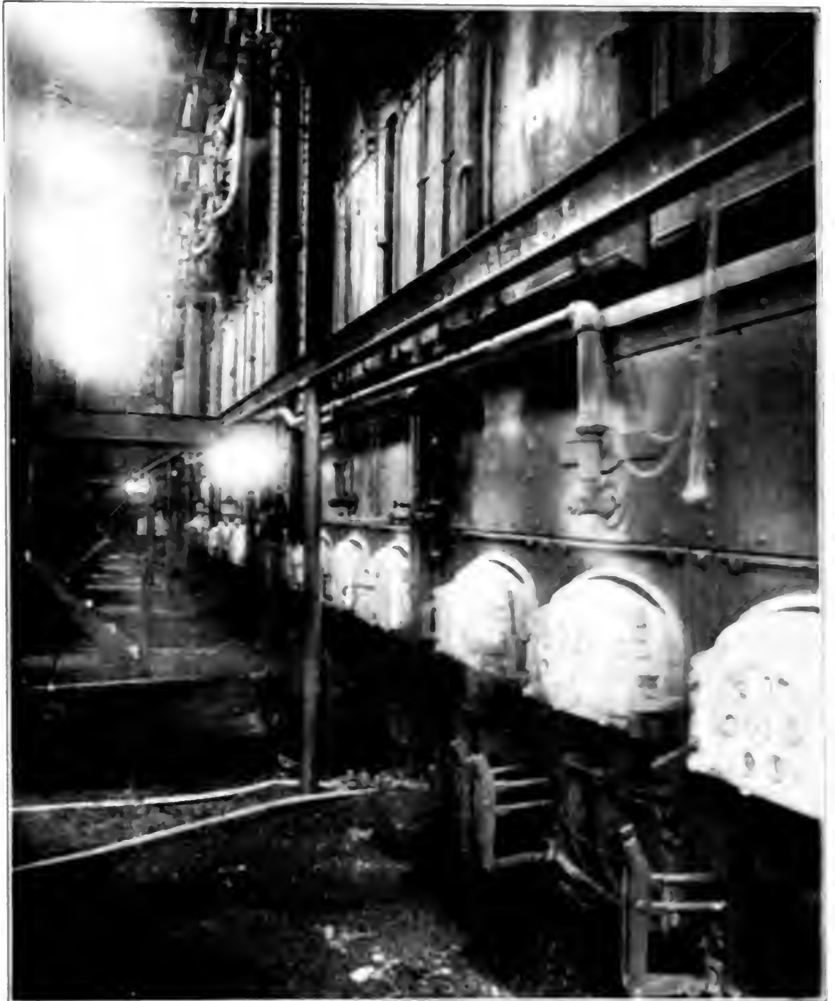
FIG. 2. FRONT OF BOILER WITH AIR FLOW DUCT.
