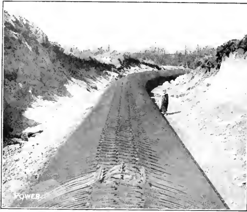
FIG. 5. TWELVE-FOOT WOOD-STAVE PENSTOCK
