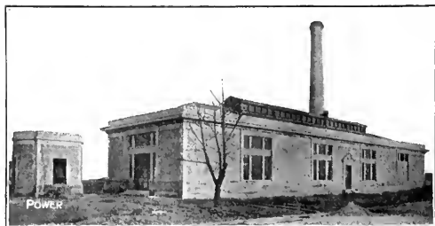
FIG. 2. FAIRVIEW SEWAGE-PUMPING STATION
