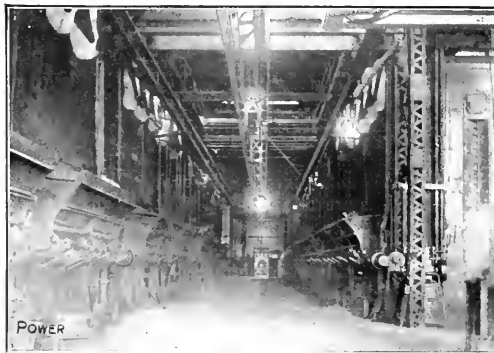
FIG. 5. OLD BOILER ROOM
