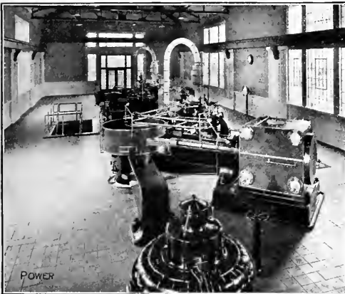
FIG. 4. ANGLE-COMPOUND PUMPING ENGINES
