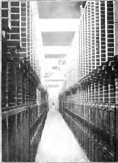
FIG. 11. BUSBAR COMPARTMENTS
