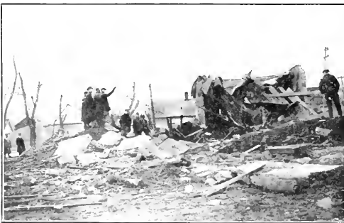
FIG. 1. WRECKAGE AFTER BOILER EXPLOSION
