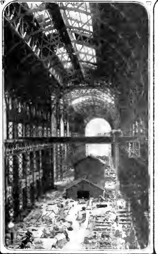
HANDLING MATERIAL WITH OVERHEAD CRANE
