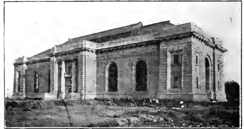
FIG. 1. NEW PUMPING STATION IN WATERWORKS PARK, DETROIT
