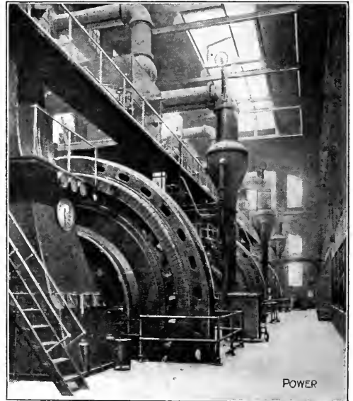
FIG. 2. VIEW OF THE OLD ENGINE ROOM, WESTPORT POWER HOUSE
