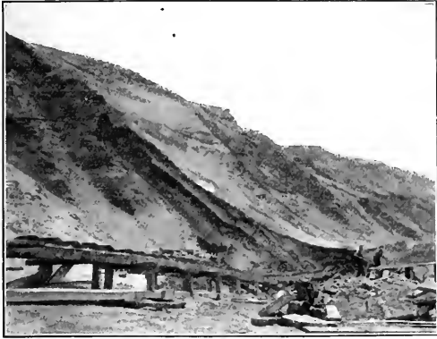
FIG. 8. CULM BANK AND SCRAPER CONVEYOR
