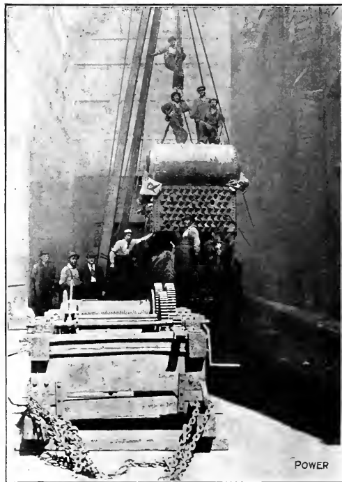
FIG. 2. HOISTING A BOILER ONTO A WAGON
