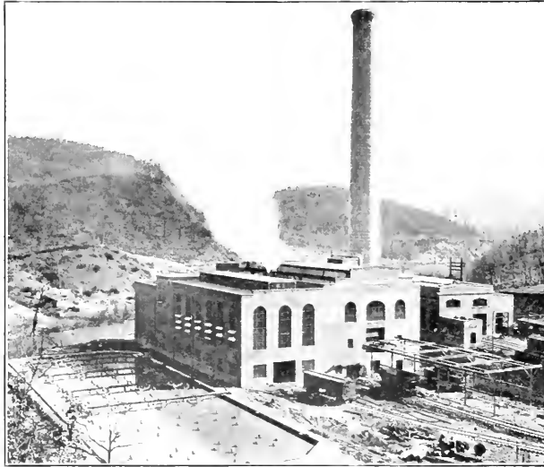
FIG. 1. POWER-PLANT BUILDING AND SPRAY POND
