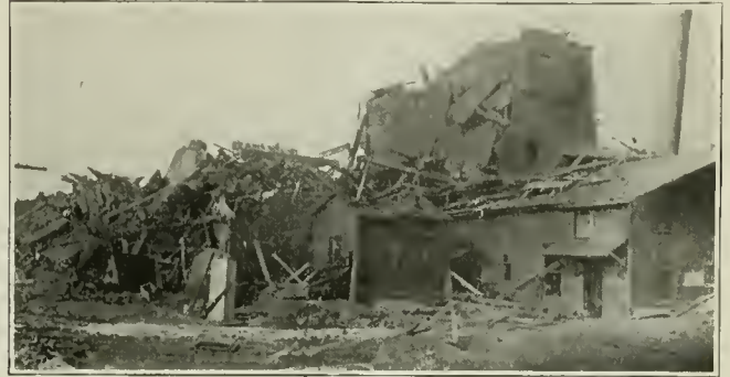
FIG. 1. WRECKED BY AN EXPLODING GARBAGE DIGESTER
