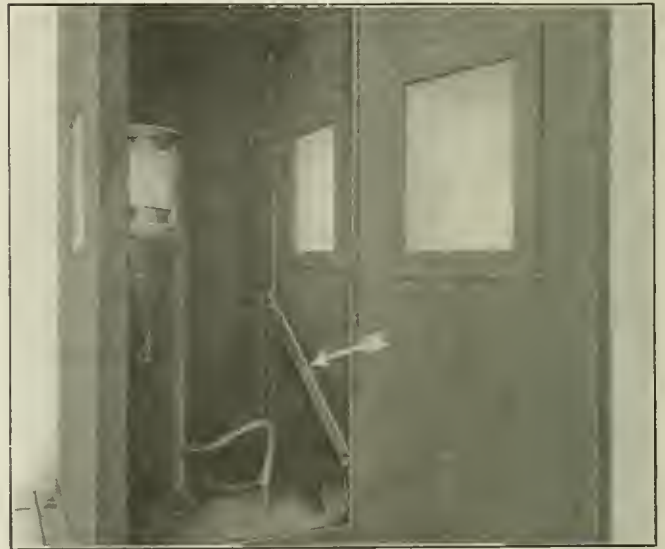
HEATER INSTALLED IN GAS-VALVE HOUSE
