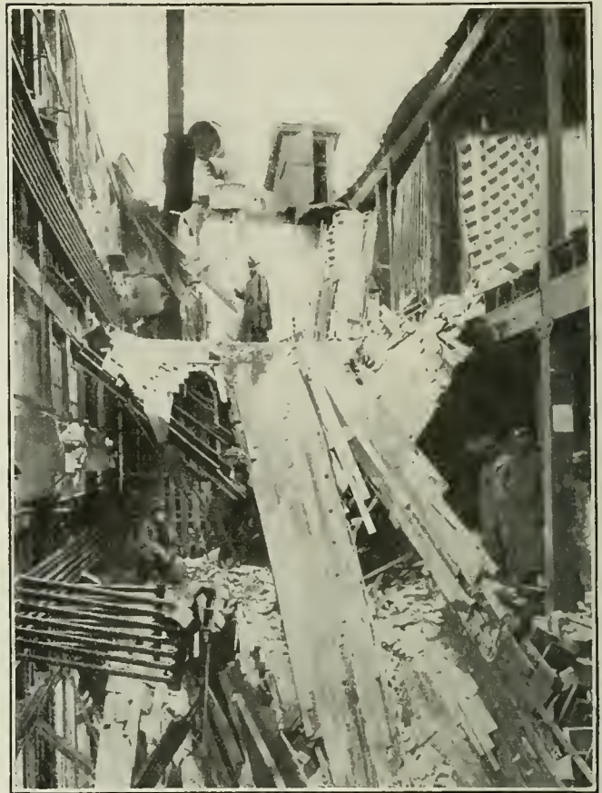
FIG. 2. THREE FLOORS WERE DEMOLISHED
