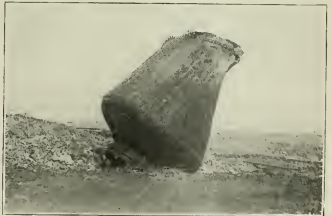
FIG. 2. TOP OF THE EXPLODED DIGESTER
