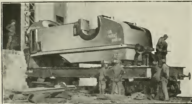
FIG. 1. UNLOADING THE ENGINE BEDPLATE AT THE PLANT
