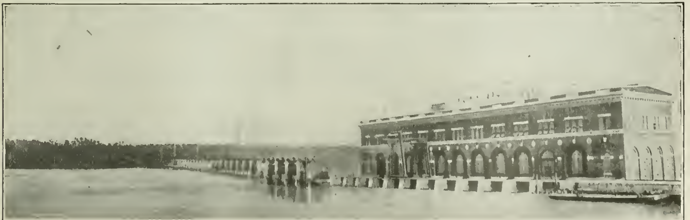
FIG. 9. LOCK 12, HYDRO-ELECTRIC PLANT—UPSTREAM VIEW
