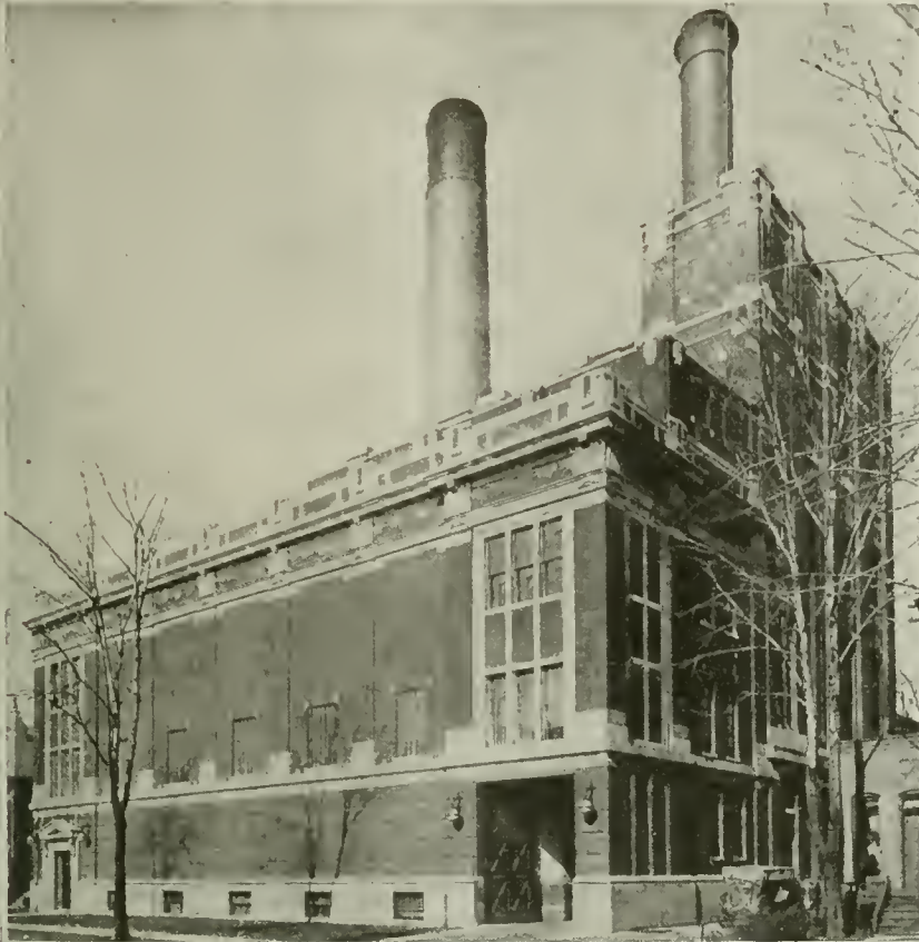
Willis Ave. Plant
