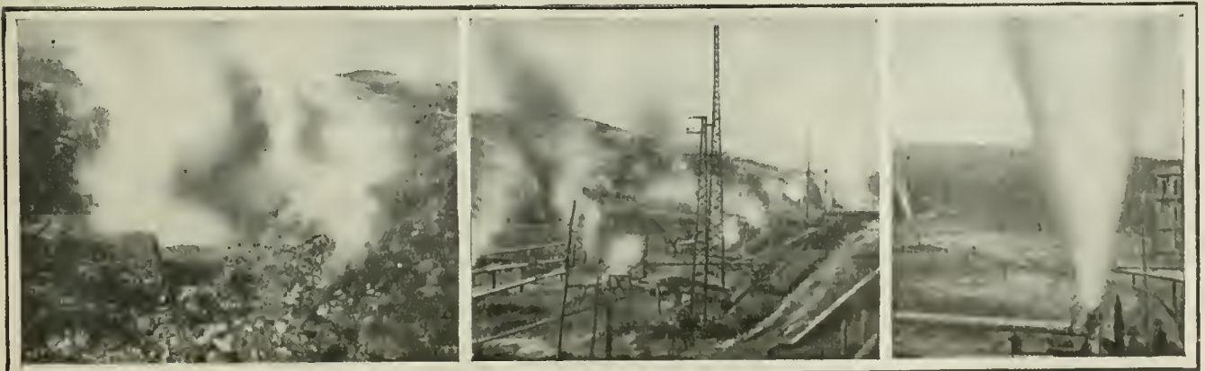
STEAM FROM EARTH FISSURES, STEAM-PIPE LINES AND STEAM JET ISSUING FROM A PIPE
