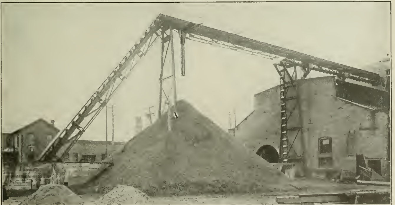
FIG. 5. BUCKET CONVEYOR AT THE AMERICAN RAILWAYS CO., DAYTON, OHIO
