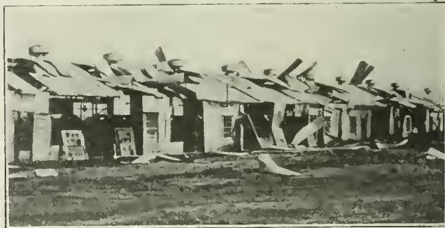
BUILDING WRECKED BY GAS EXPLOSION
