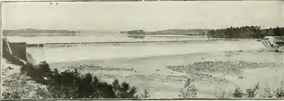
FIG. 14. "YADKIN" RIVER POWER CO., BLEWETT FALLS, DAM AND POND
