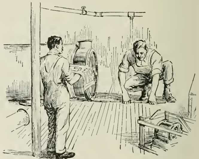
PROVIDING SPACE TO MAKE REPAIRS
