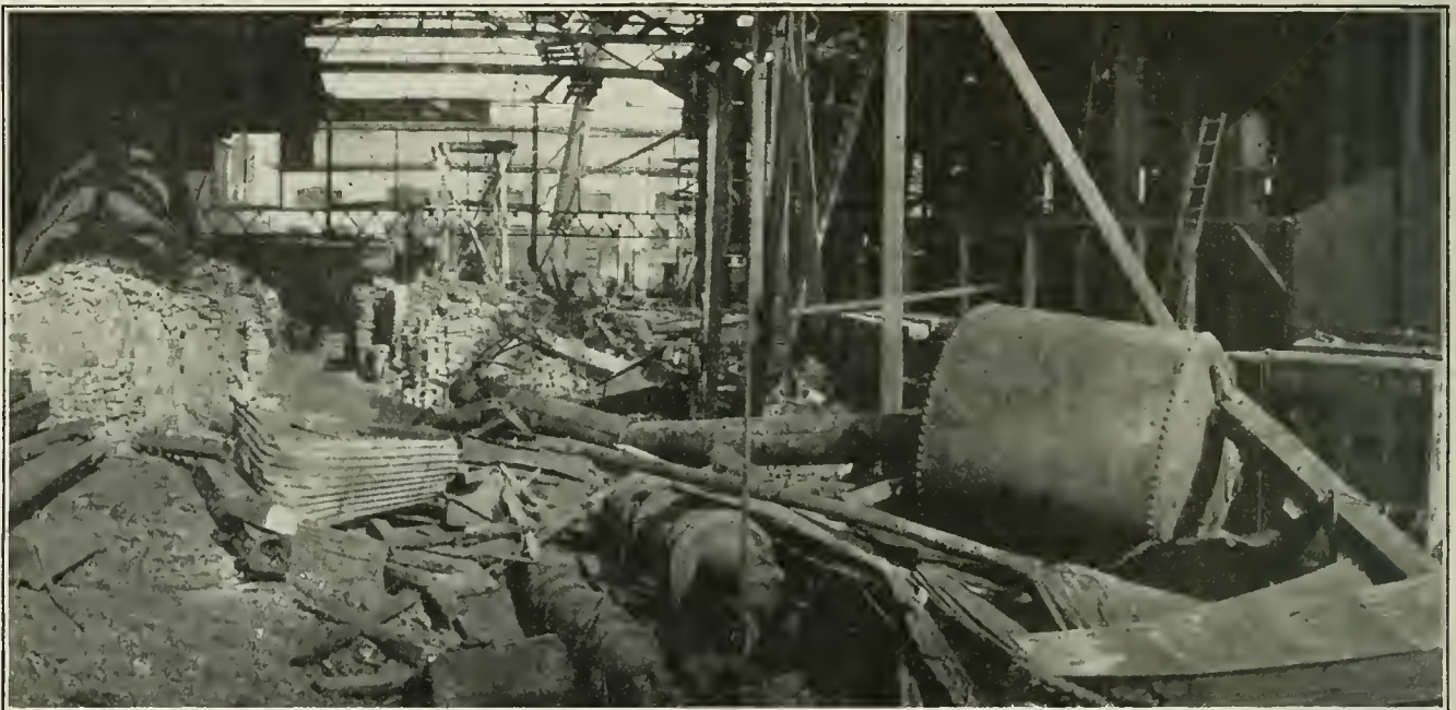
FIG. 1 GENERAL VIEW OF WRECKED BUILDING; STACK STICKING IN BOX-CAR IN BACKGROUND
