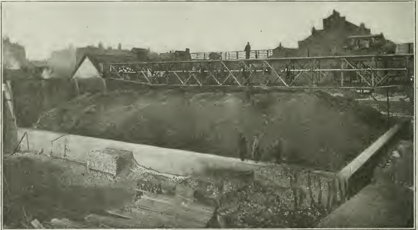
FIG. 1. CONCRETE COAL-STORAGE PIT OF THE OMAHA ELECTRIC LIGHT AND POWER CO.
