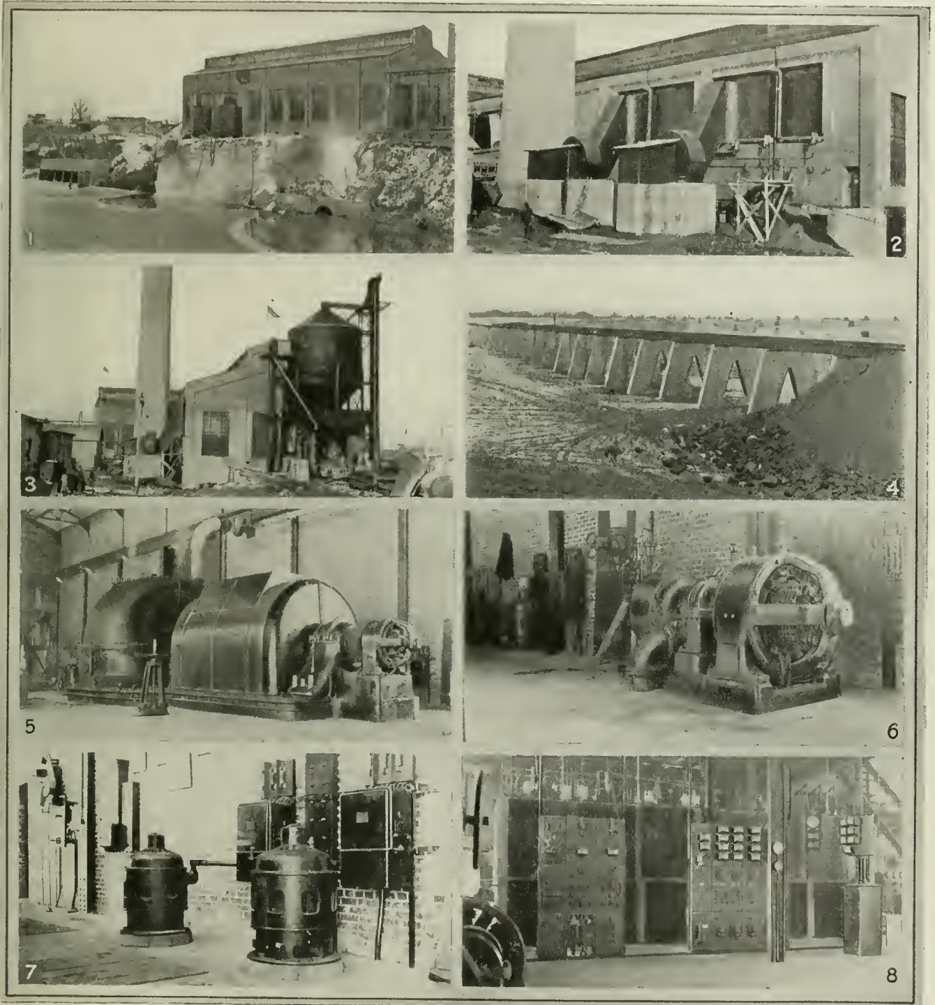
FIGS. 1 TO 8. GENERAL VIEWS IN AND ABOUT THE NEW POWER PLANT
