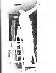
Workman finishes painting the church lobby.
