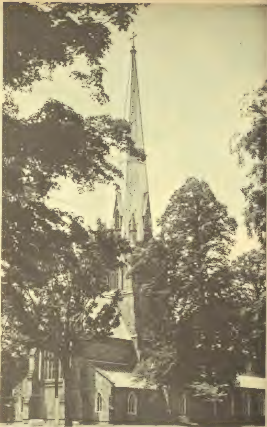
Christ Church Cathedral, a good example of Gothic architecture in North America.
