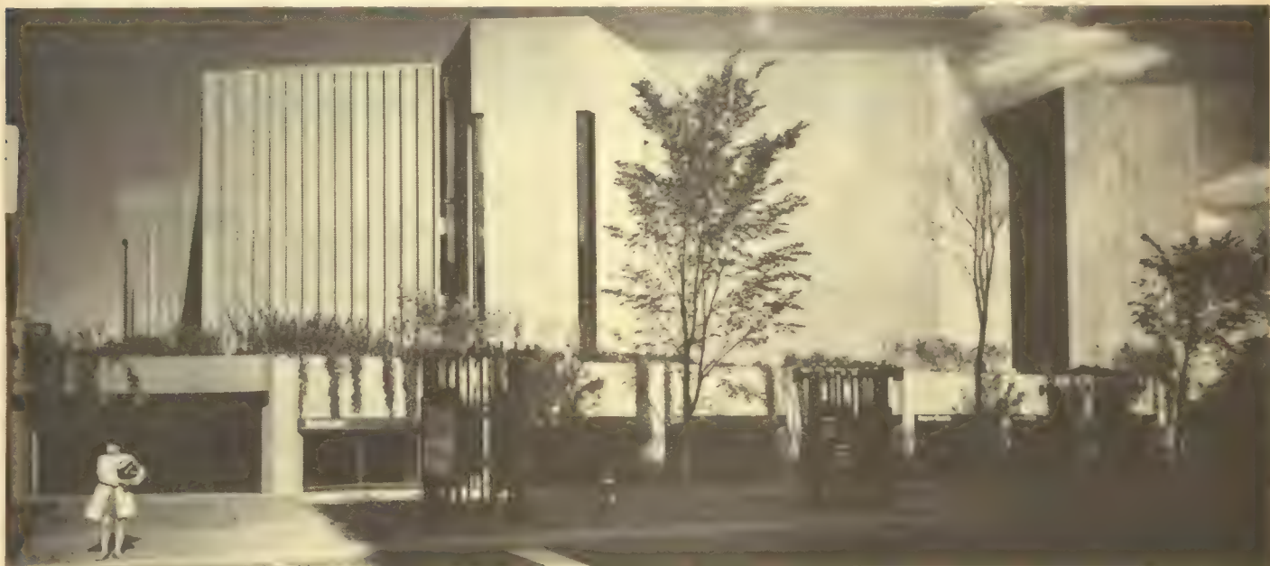
This front view of the National Arts Centre gives some idea of its multi-faced character. The complex, developed as a series of hexagonal buildings on terraces of varying levels, is situated on six and one-half acres in the heart of downtown Ottawa.
