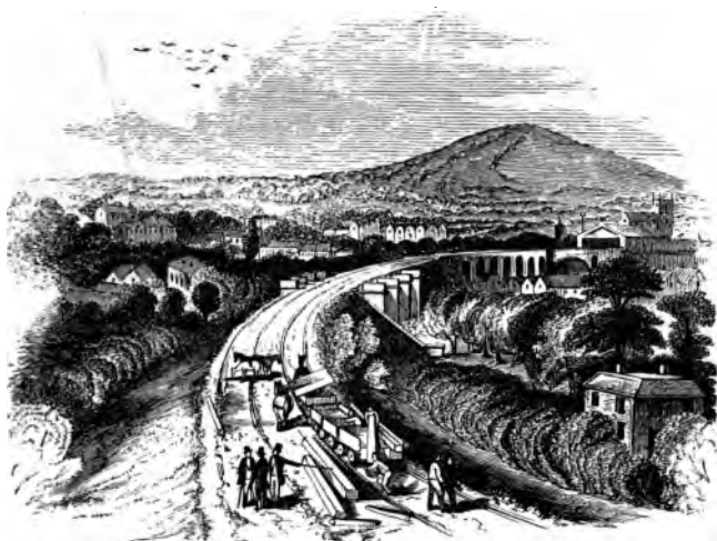
RAILWAY EMBANKMENT NEAR BATH.
