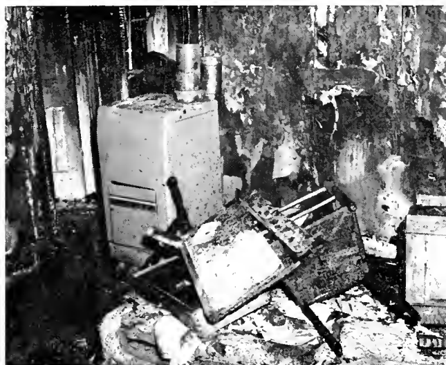
Reports indicate oil from a space heater leaked out over the floor and ignited.
